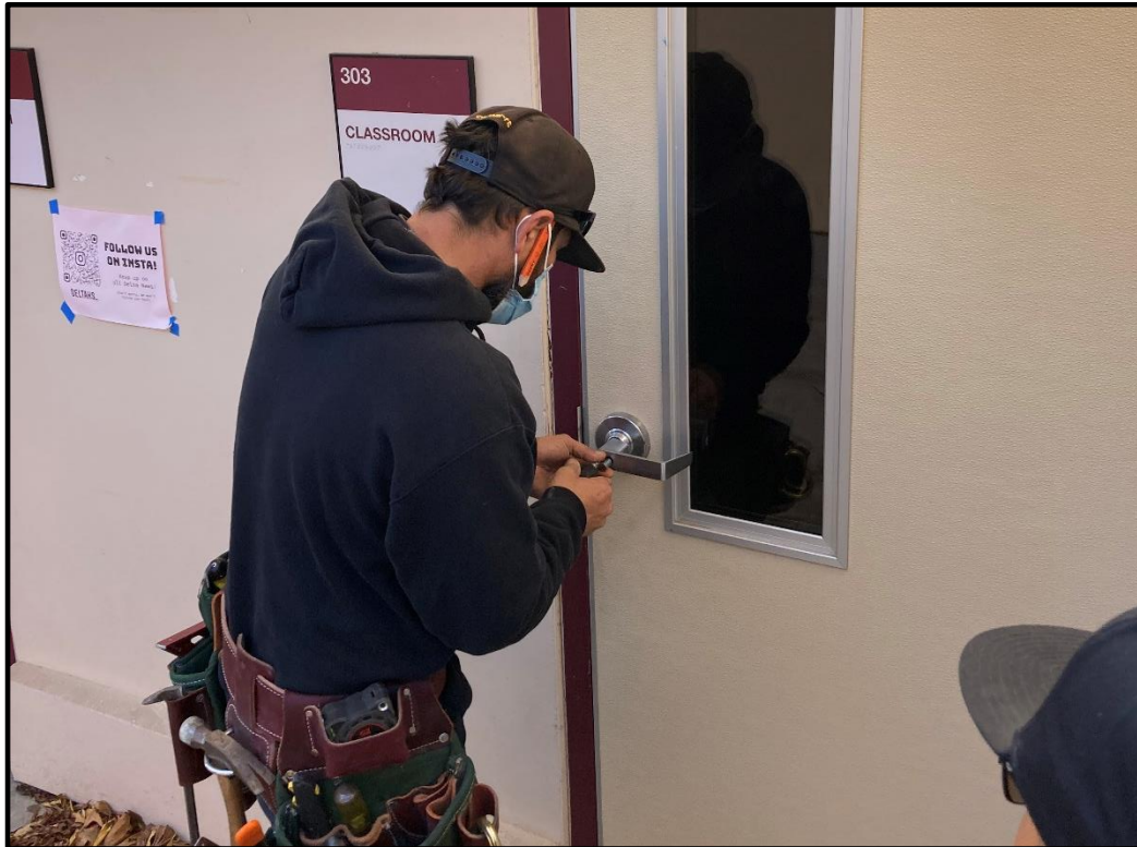
DHS – Tom Harbold Replaces Cyber Lock Cores on Exterior Doors
