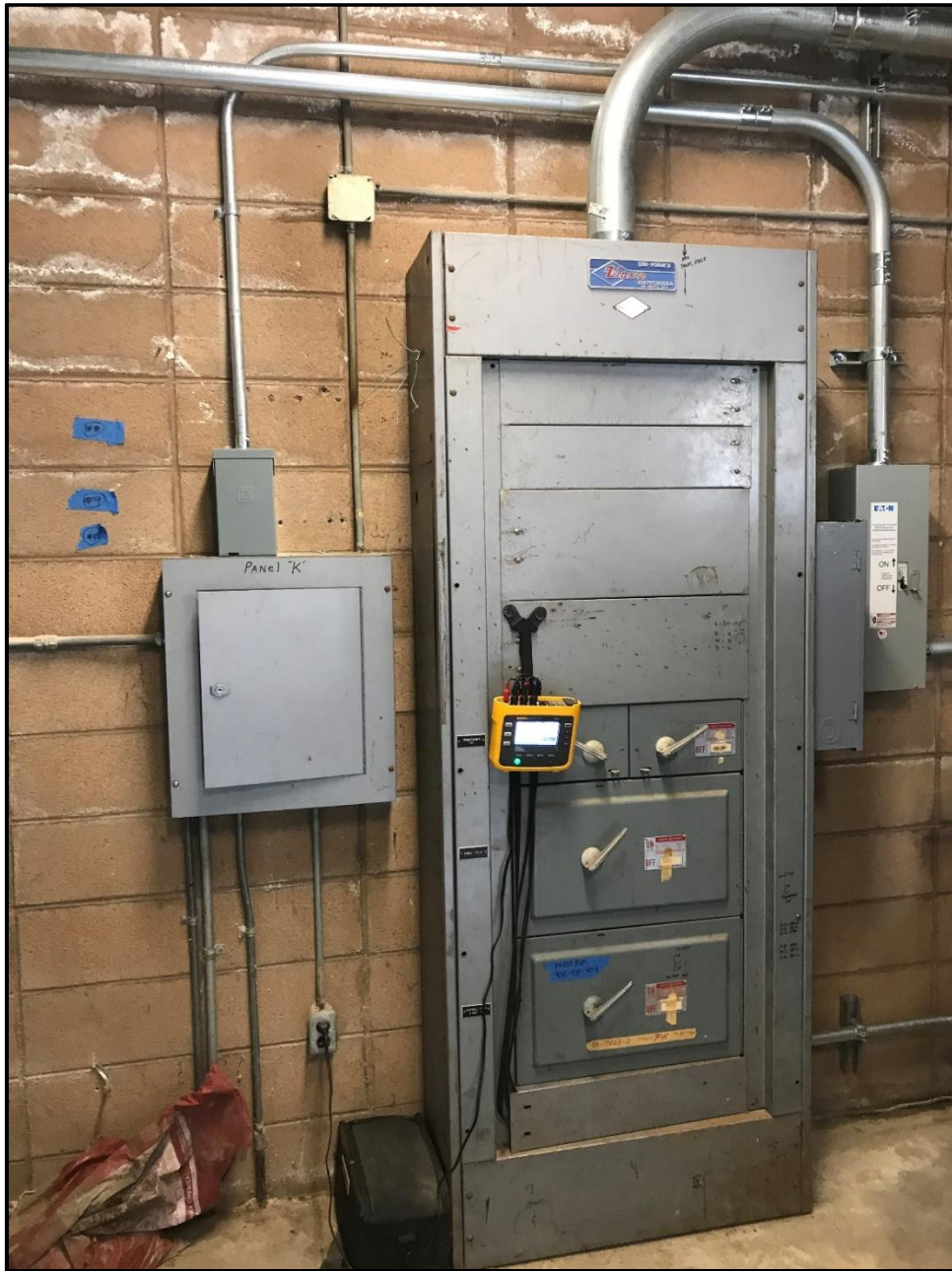
ERHS Maintenance and Operations Building – Original Zinsco Electrical Switchgear to be Replaced
