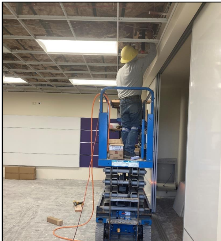
ERHS Modernization – Monitor Mounts are Installed above the T-Bar Ceiling
