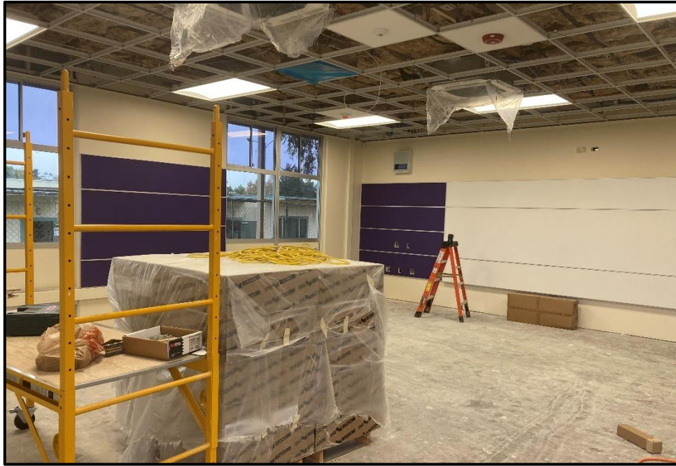
ERHS Modernization – Pinable Surfaces and Whiteboards Dress up the Classrooms
