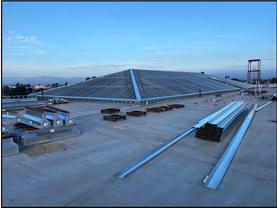
SMHS 50-Classroom Building – Roof Framing is Underway...Bell Tower in the Background
