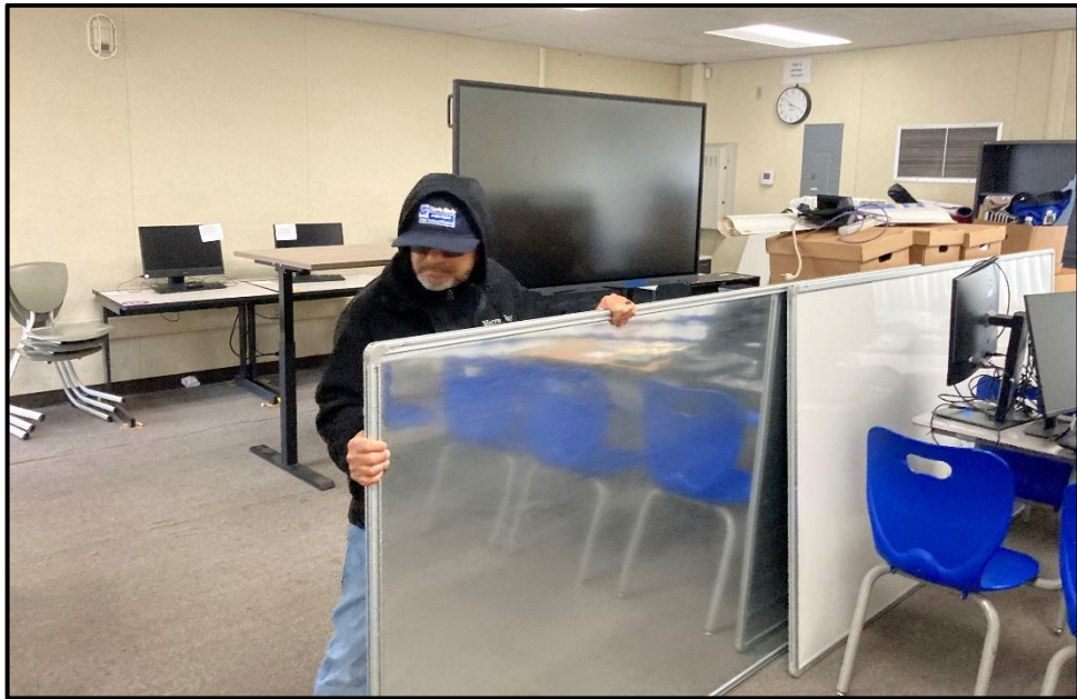
ERHS – Jimmy Salutan Removes a Whiteboard for Classroom Modernization
