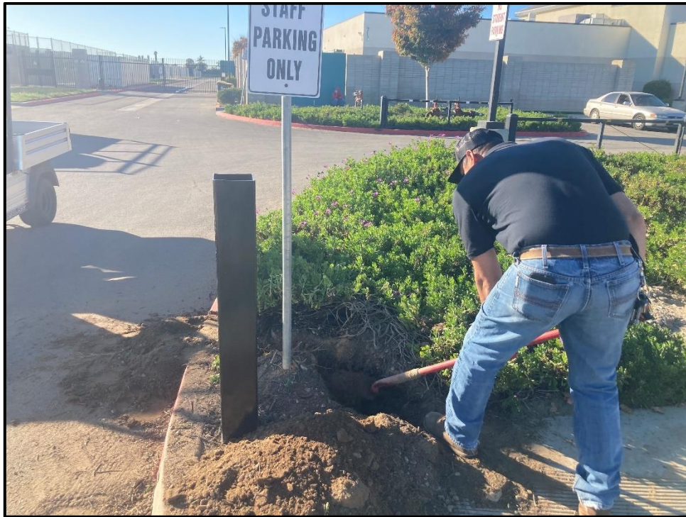
PVHS – Jose Gamino Repairs a Broken Sprinkler in the Front Planter
