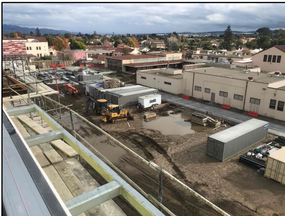
SMHS 50-Classroom Building – Overall View of the Future Quad from the Third Story Roof
