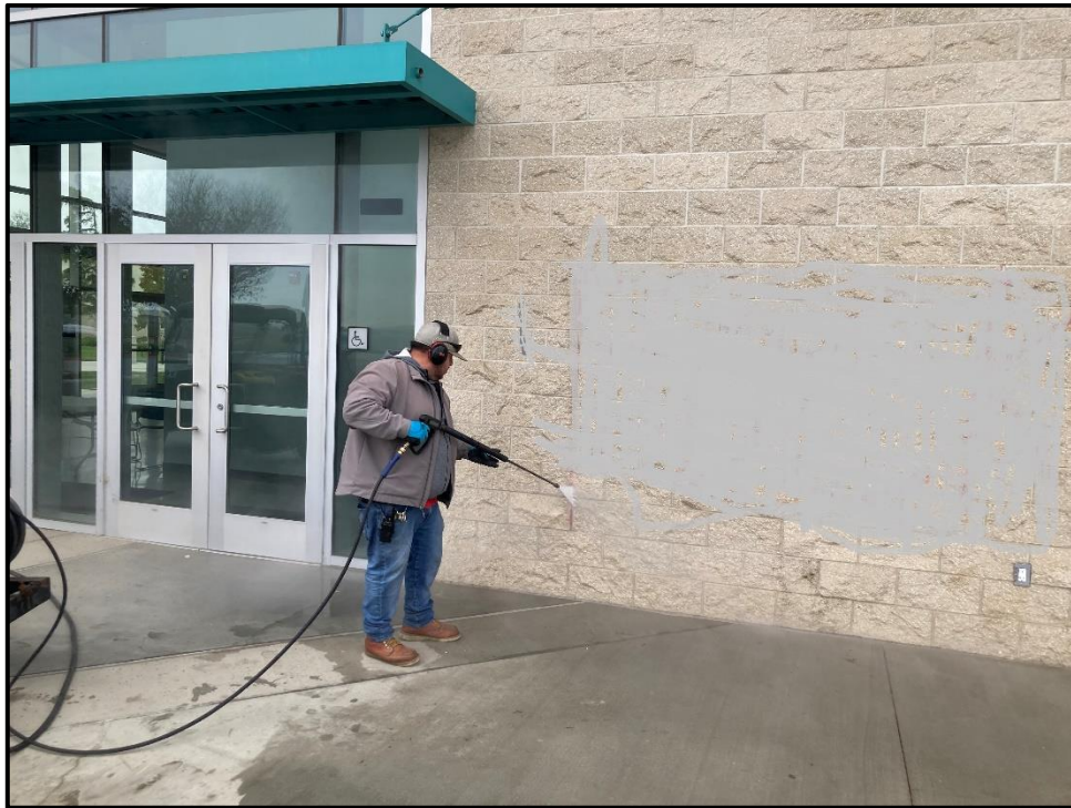
PVHS – Paul Alavarez Pressure Washes Graffiti on the Performing Arts Center
