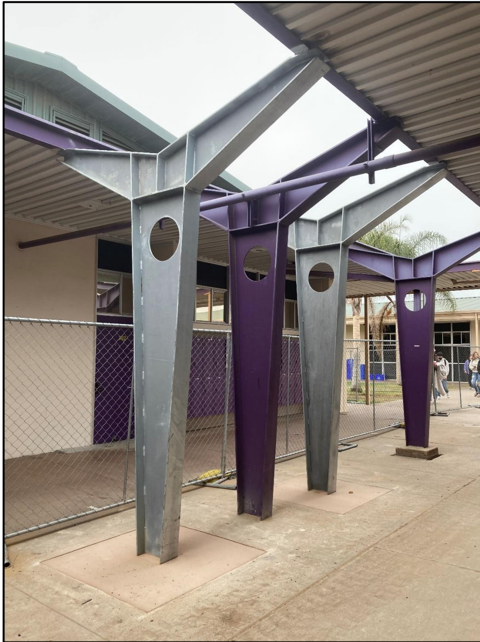
ERHS Modernization – Heating and Air Conditioning Requires Reinforcement of Covered Walkways
