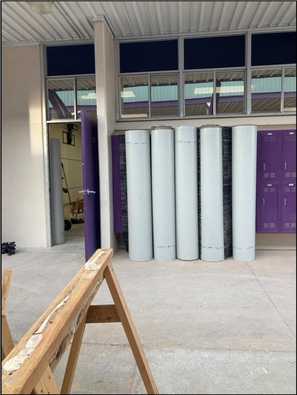
ERHS Modernization – New Classroom Carpeting Awaits Installation
