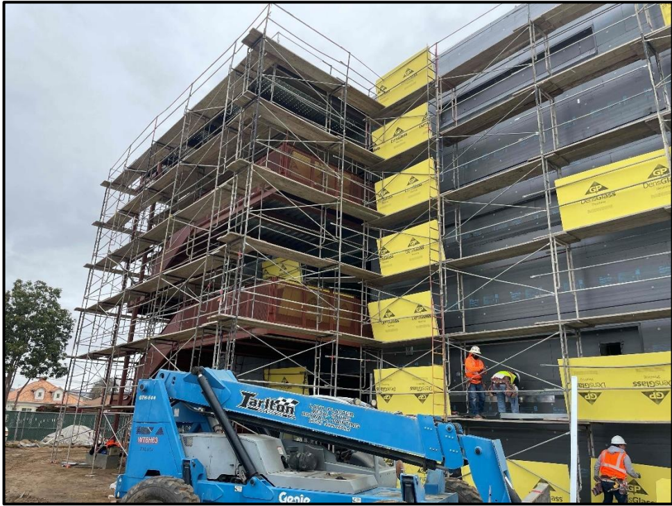
SMHS 50-Classroom Building – Exterior Installation Requires Multiple Layers of Scaffolding
