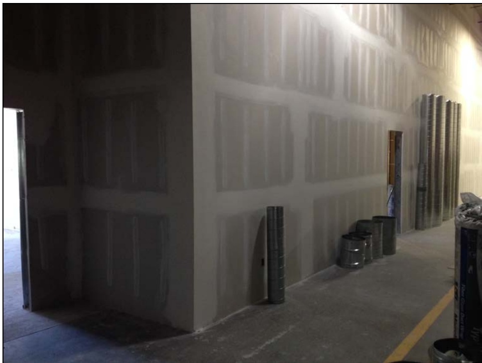
Support Services Center – Multi-purpose Room Exterior Drywall in Place
