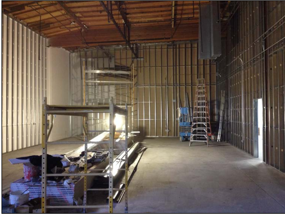
Support Services Center – Multi-purpose Room Framed and Electrical Conduit Installation Begins
