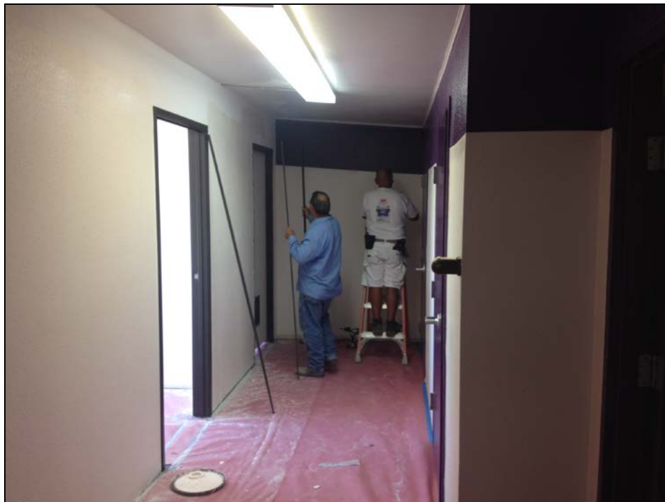
ERHS – Finish Carpentry and Painting in the Football Press Box Before the Big Game
