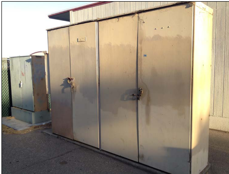
SMHS – Portable Classroom Electrical Panel Locks Repaired
