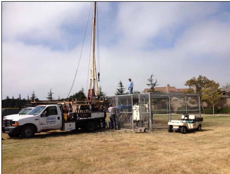
PVHS – Irrigation Well Submersible Pump and Motor Removed for Replacement
