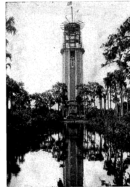
The Bok tower nearing completion.
