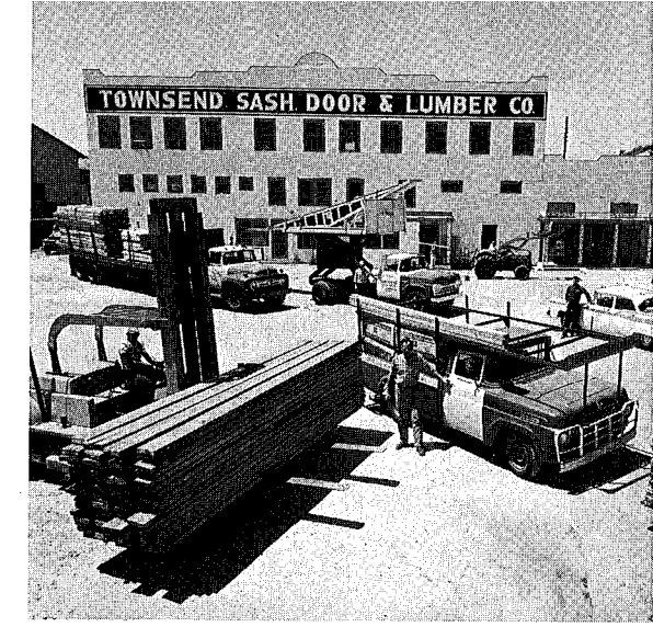
TOWNSEND SASH DOOR & LUMBER CO. Paint—Repair—Re-roof
