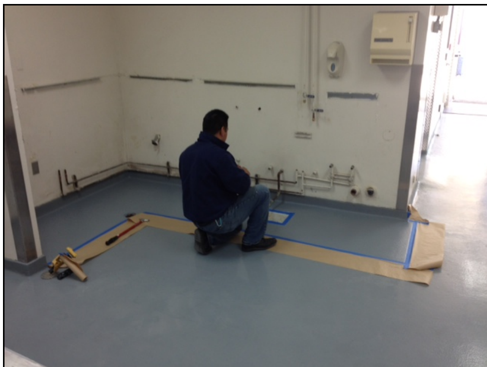
ERHS - Cafeteria Kitchen Floor Patch in Progress
