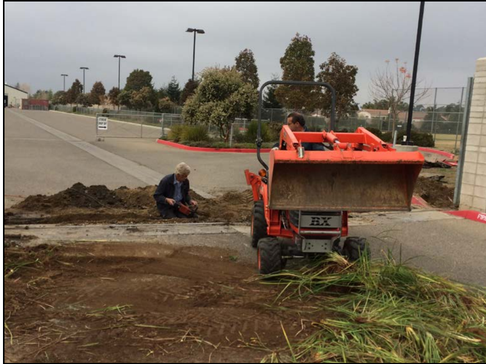
PVHS – José Placencia & John Swanson Prepare for Remote Gate Operator
