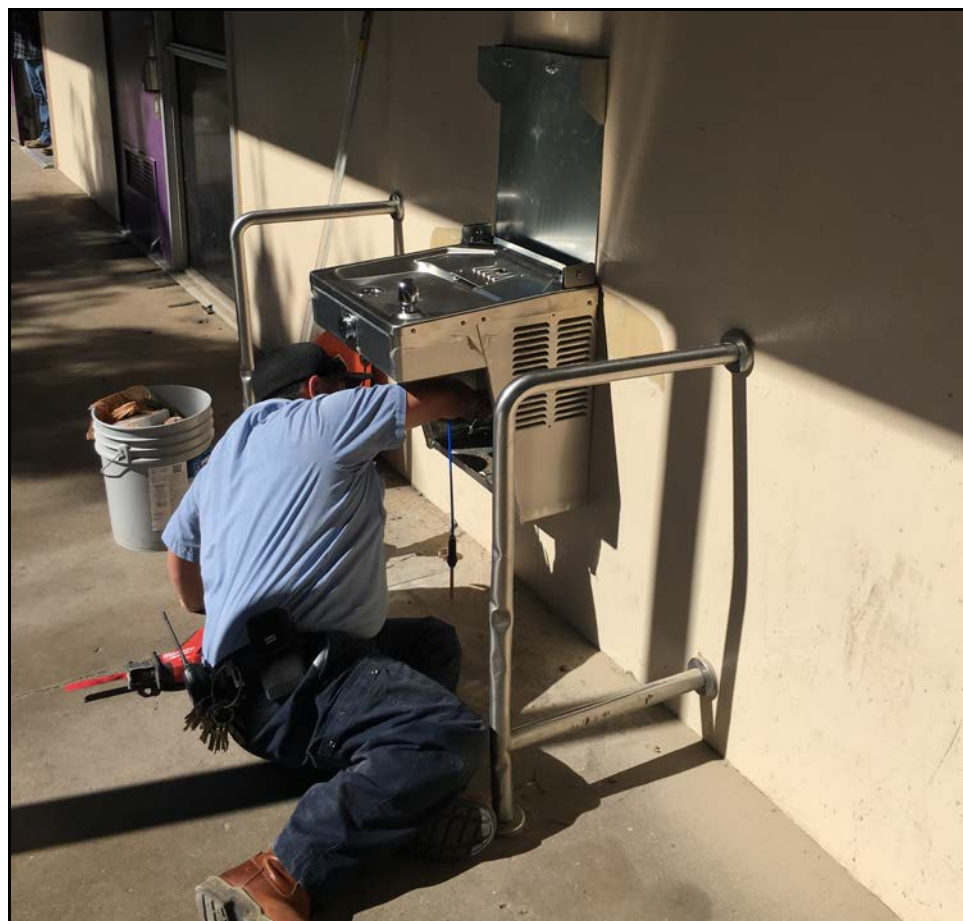
ERHS – Jesus Reyes Installs a New Hydration Station on the Gymnasium/Industrial Arts Level of Campus
