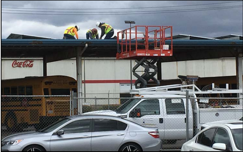
SSC Solar Power – Electricians Connect Panels on the Bus Barn Roof
