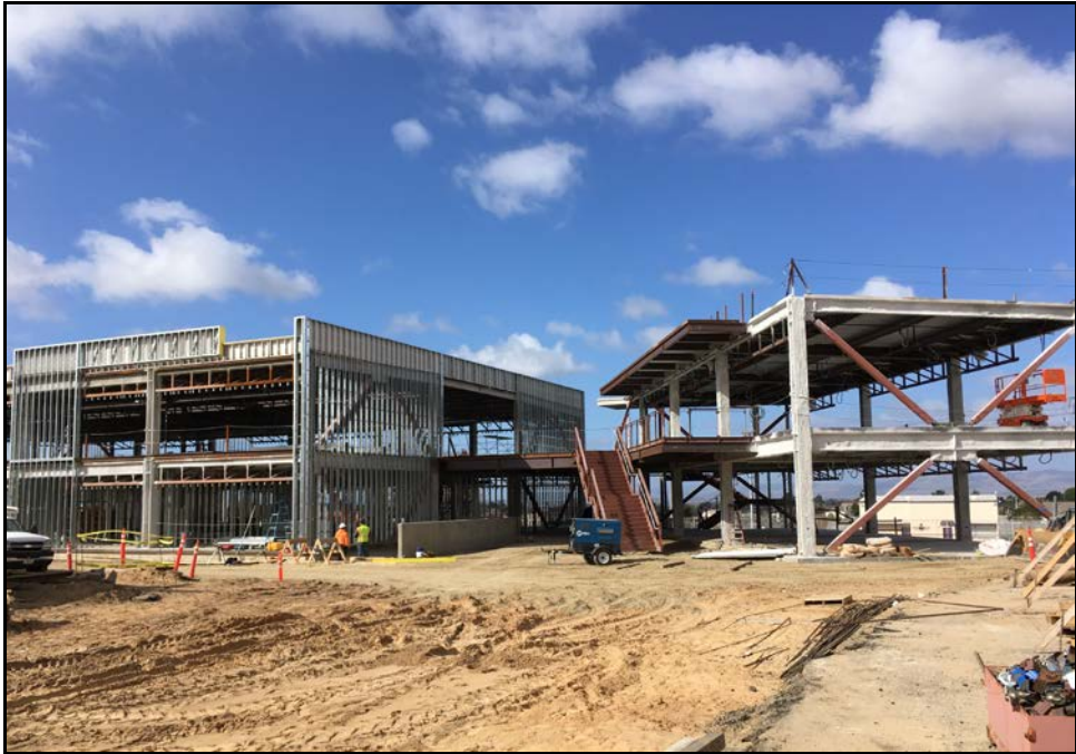
ERHS 38-Classroom Building – Metal Stud and Stairway Installation
