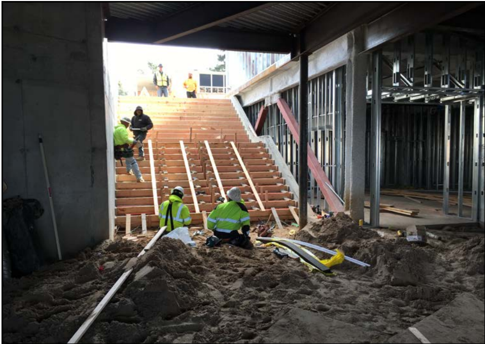
ERHS 38-Classroom Building – Forming Concrete Stairway to the First Floor
