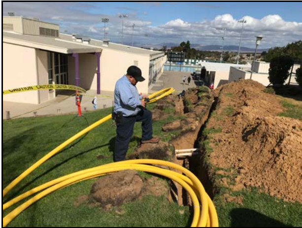
ERHS – Maintenance Crew Replaces a Natural Gas Line
