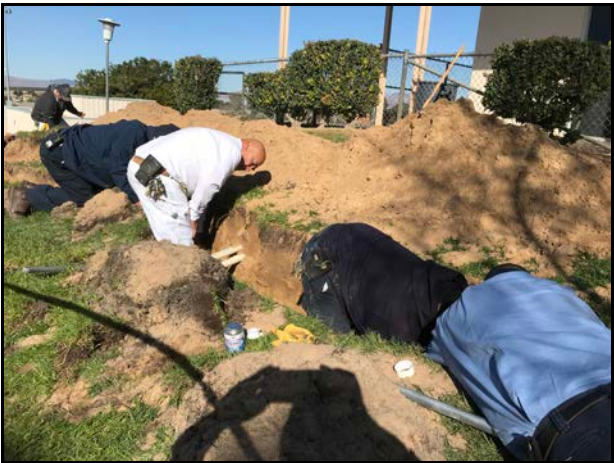
ERHS – Maintenance Crew Replaces a Natural Gas Line
