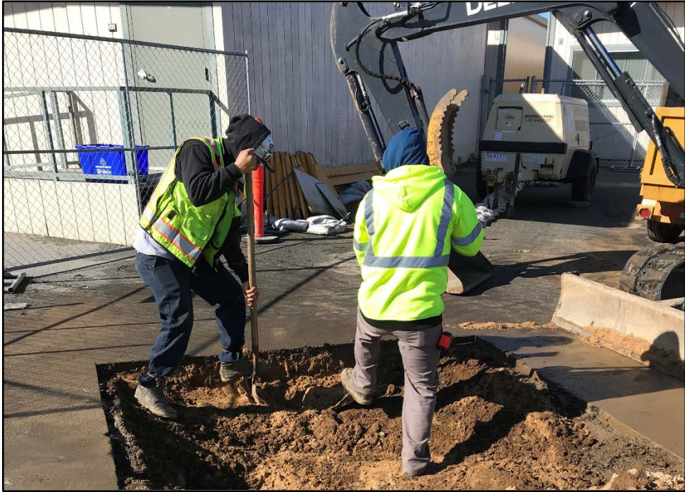
ERHS - Excavation Progresses to Control the erosion at the Bradley Road Parking Lot
