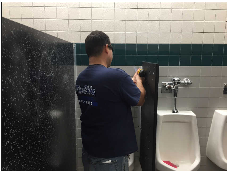
PVHS - Elias Camacho Re-installs a Damaged Restroom Partition
