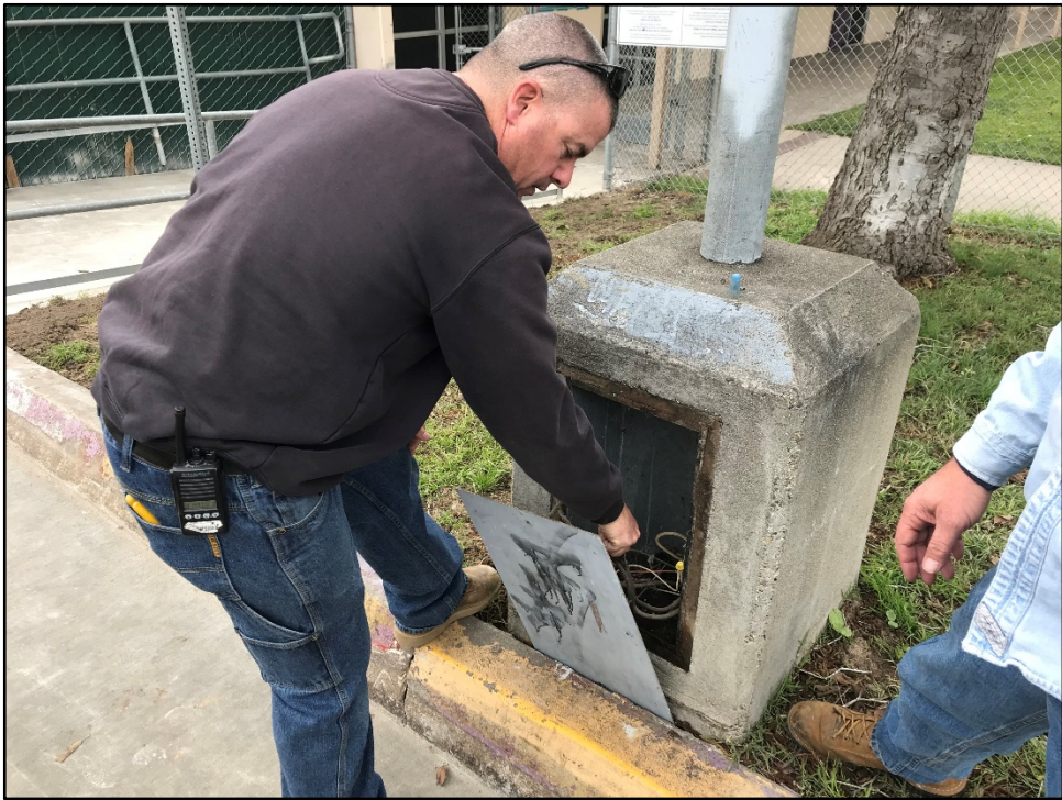
ERHS - Electrician Andy Freitas Repairs the Student Parking Lot Lighting
