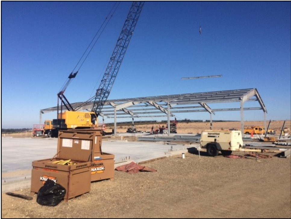
CTE Ag Center – Shop Building B Steel Assembly is Underway
