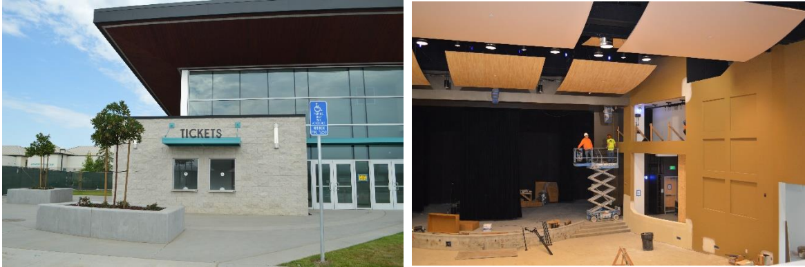
Pioneer Valley High School Performing Arts Center Construction Progress (August 2017)
