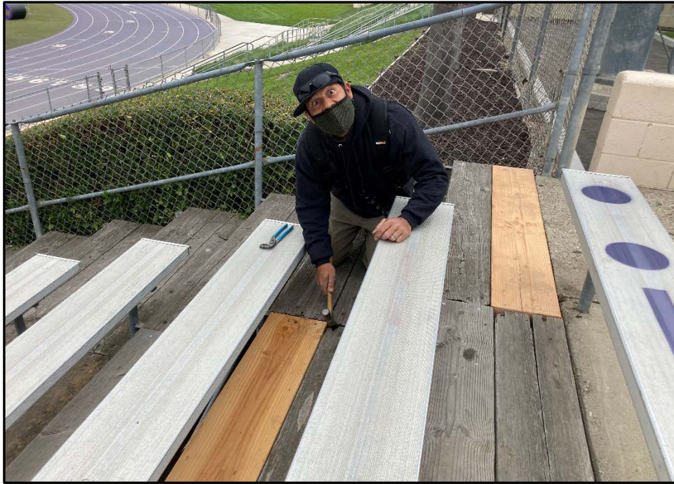
ERHS - New Carpenter Tom Harbold Prepares the Bleachers for Graduation
