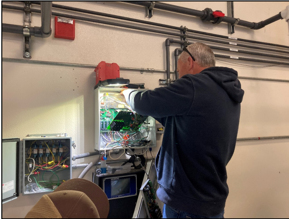
ERHS - Del Ward Diagnoses Pool Control Problems
