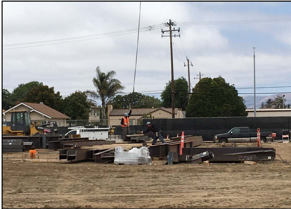
SMHS 50-Classroom Building – Sorting and Preparing Steel Columns
