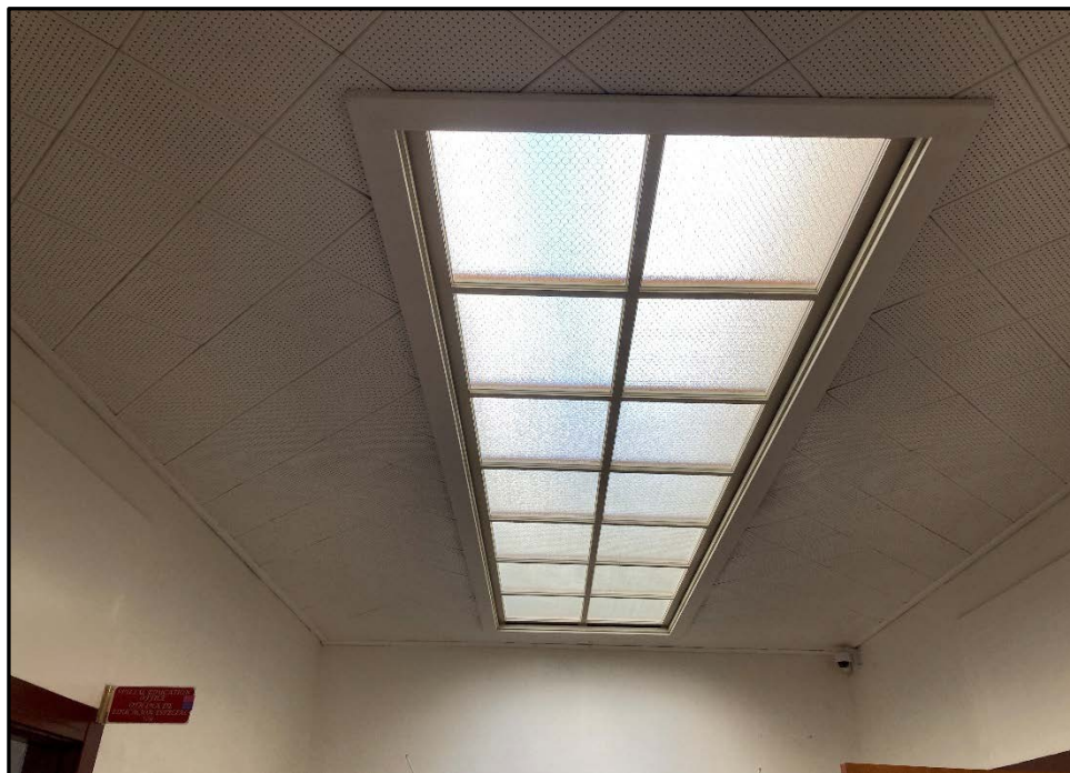
SMHS – Maintenance of the Administration Building Includes Cleaning the Skylights
