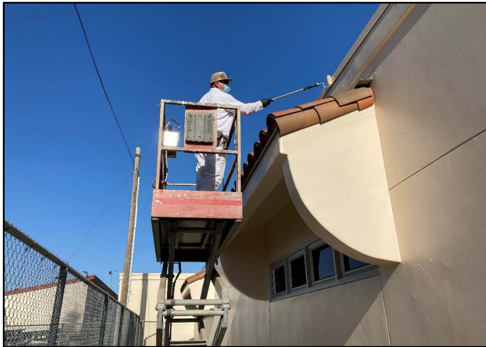
SMHS – Ernest Paz Paints the 230 Business Building Exterior
