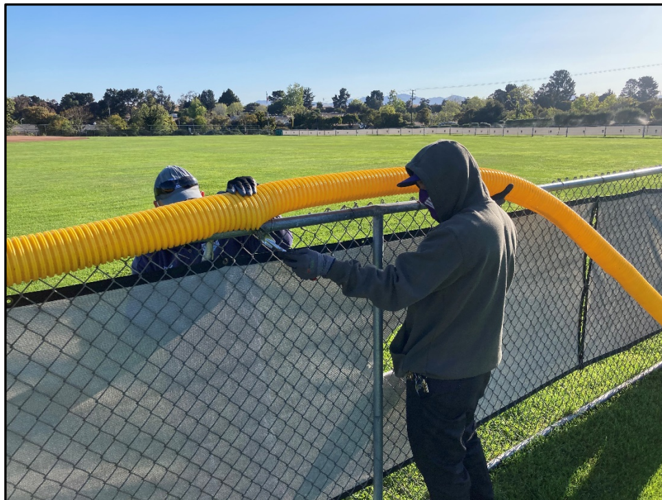
ERHS - Jordan Markstone and Joseph Campos Replace the Safety Cap on the Baseball Outfield Fence
