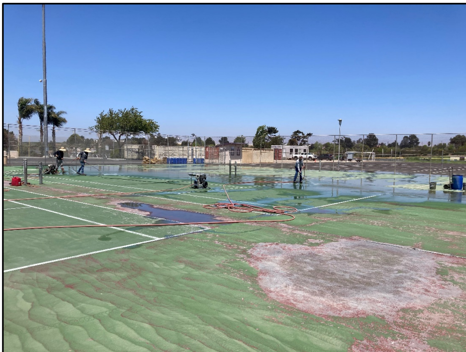
ERHS - Tennis Court Resurfacing Begins as Soon as Tennis Season Ends
