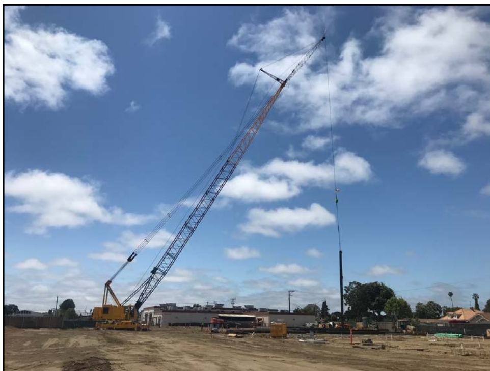
SMHS 50-Classroom Building – The First Steel Column is Set in Place!
