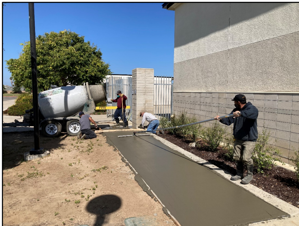
PVHS – The Crew Pours New Concrete Walkways at the Gymnasium for Improved Traffic Control
