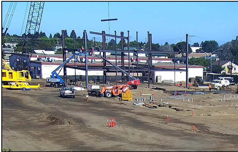
SMHS 50-Classroom Building – The Erector Set Begins Near the Industrial Arts Building
