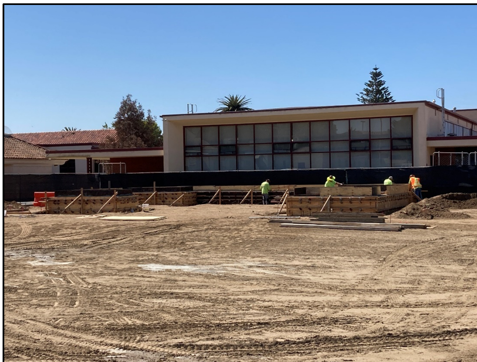
SMHS 50-Classroom Building – Forming Planters North of the Existing Library
