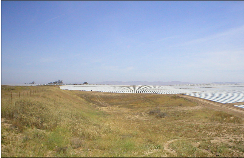
Photo 1: View of a drainage basin located at the southwest corner of the Project Site.
