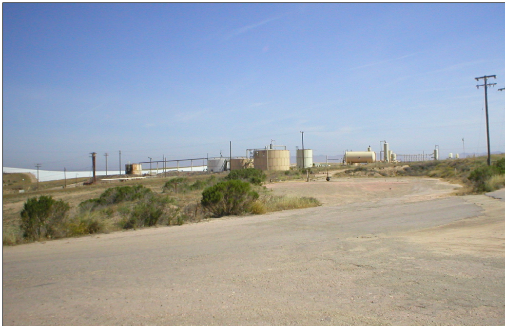
Photo 14: Greka oil field facility located approximately 1,500 feet east-northeast of the Project Site.
