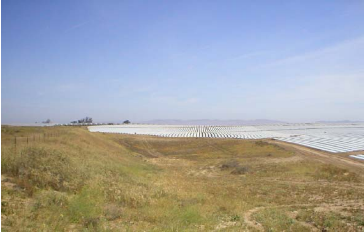
View of a drainage basin located at the southwest corner of the Project Site
