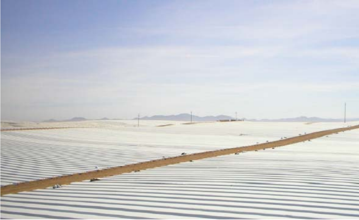
Looking northeast across the Project Site
