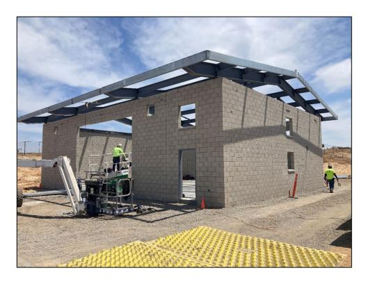
MRCTECAF M&O Building – Roof Support Installation is Completed
