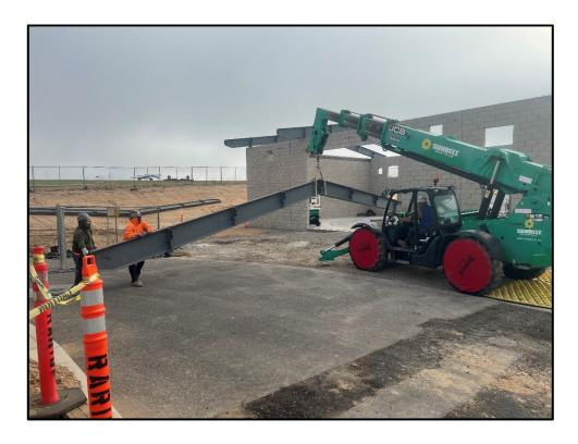
MRCTECAF M&O Building – Roof Supports are Being Installed
