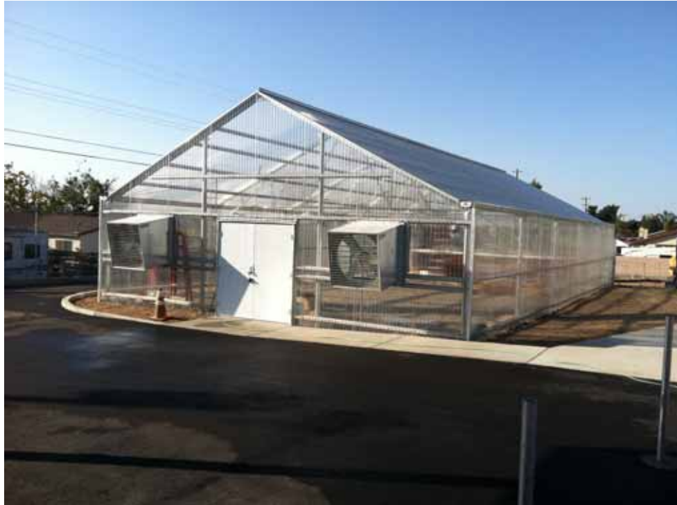
New Righetti Green House almost finished.
