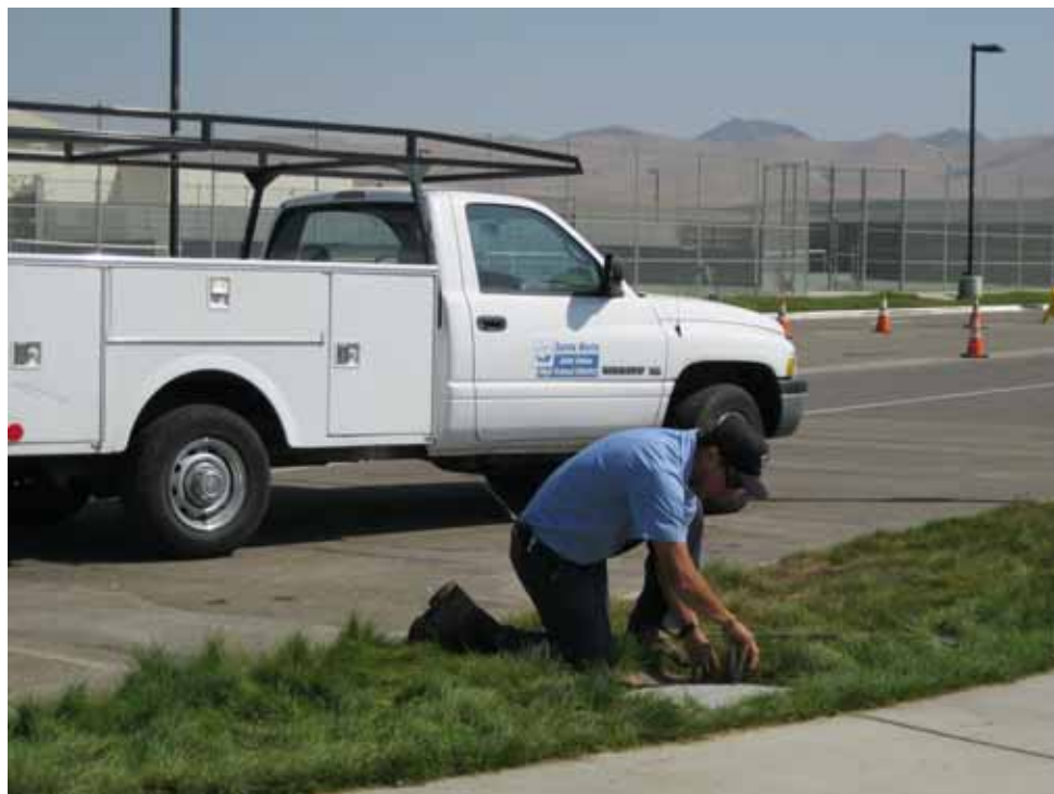
New sprinkler heads and casings at Pioneer Valley
