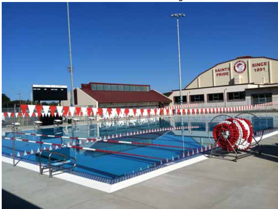
Santa Maria High School Pool ready for the Grand Opening
