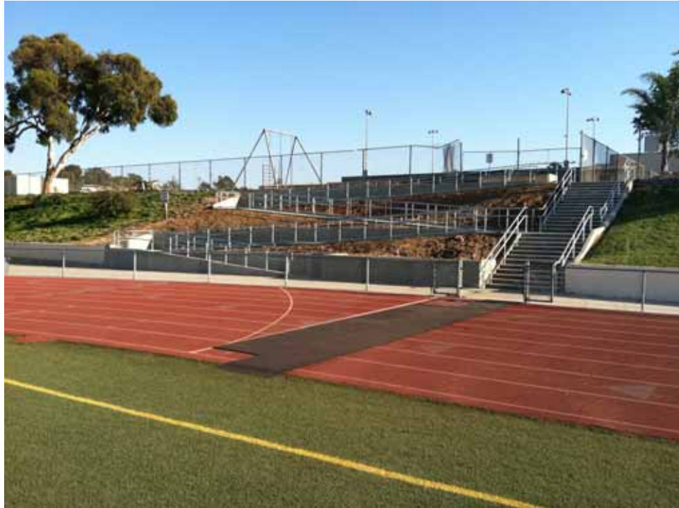
New Righetti Stadium Handicap Ramp ready for landscaping.
