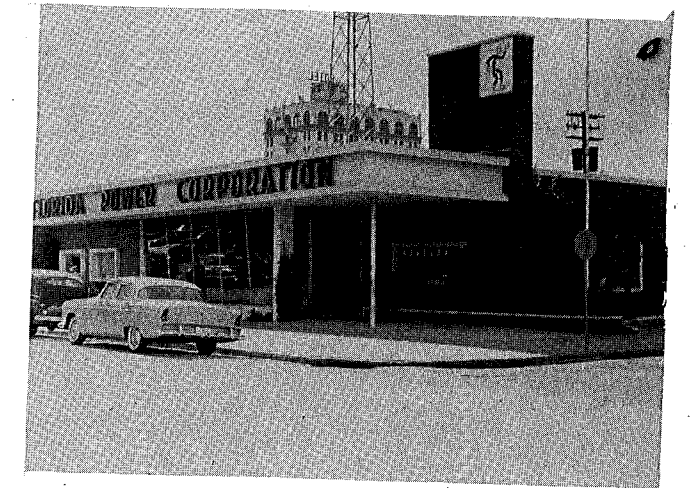
FLORIDA POWER CORPORATION
