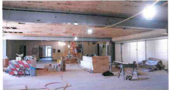
Nestucca High School Gym/Cafeteria seismic retrofit during construction, 2020
