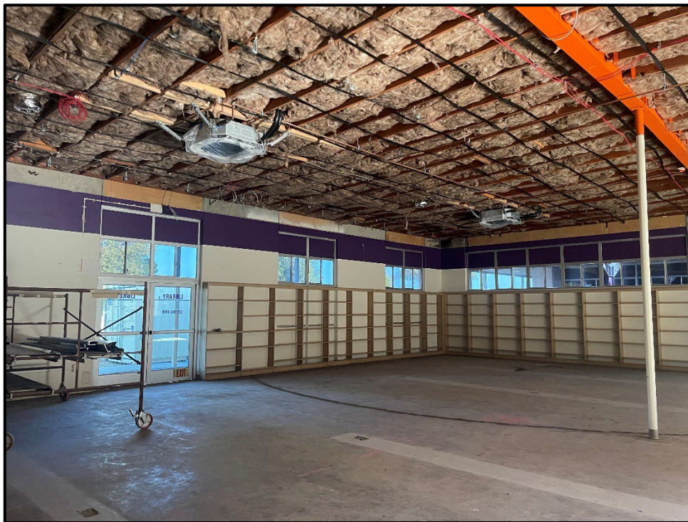
ERHS Modernization – Library is Prepared for New Interior
