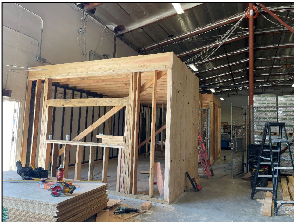
SSC Purchasing Office – Roof Joists and Shear Walls are in Place
