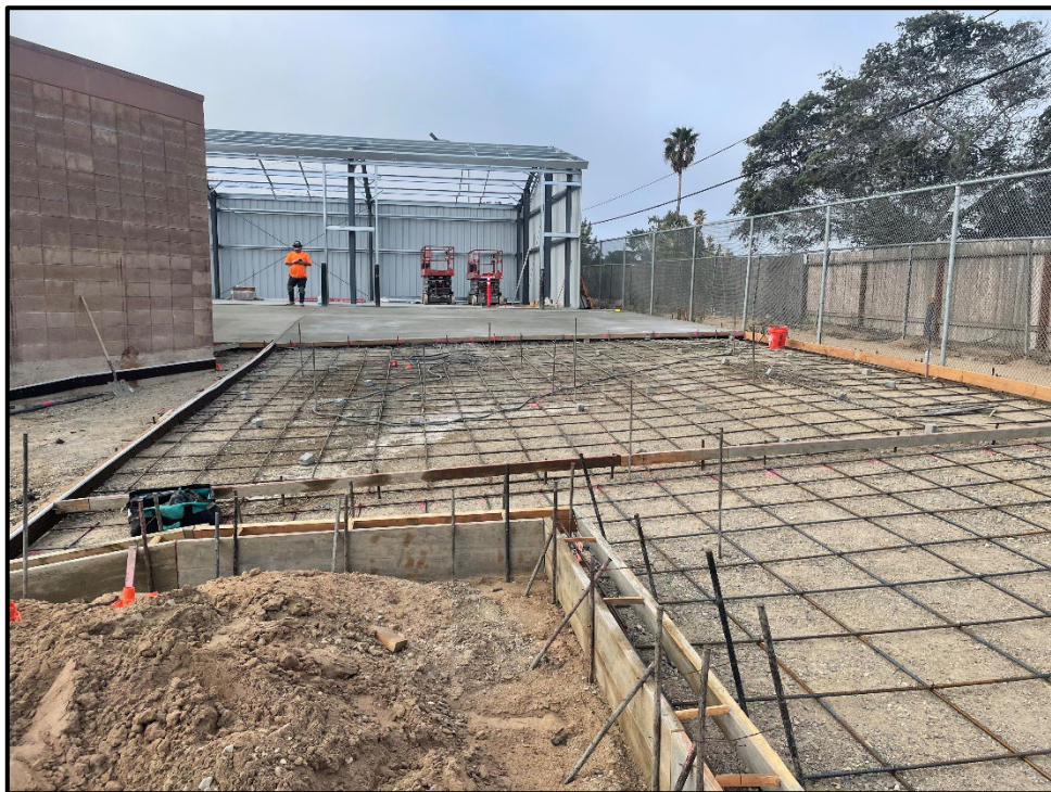
ERHS Maintenance and Operations Building – Preparation for Driveway and Parking
