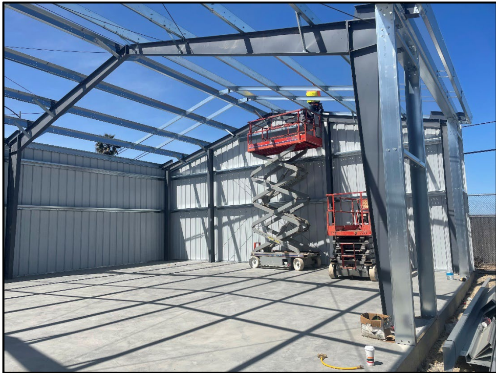
ERHS Maintenance and Operations Building – Steel Frame is Under Construction
