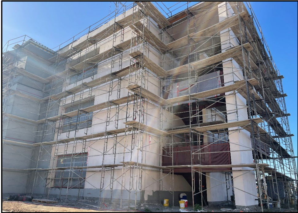
SMHS 50-Classroom Building – Exterior Stucco Process Continues
