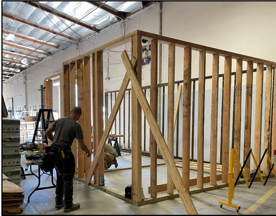
SSC Purchasing Office – Old Office Demolition is Complete and Framing Begins
