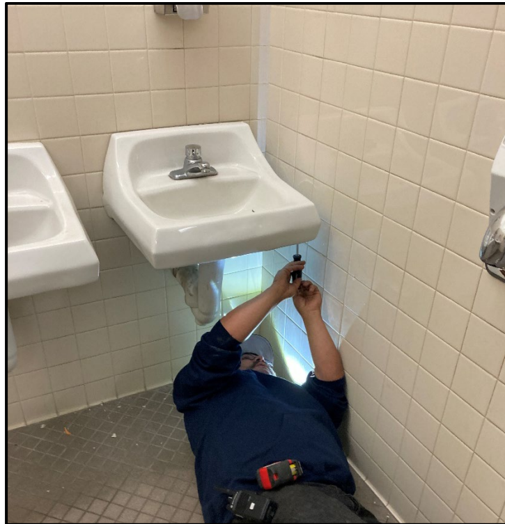
SMHS – Jesus Reyes Installing New Hardware to Re-Secure Sink
