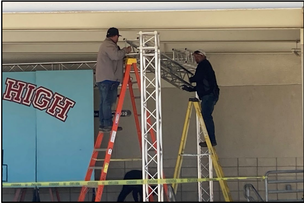
PVHS – Elias Camacho and Paul Alvarez Installing Lighting Trusses for the Grease Production
