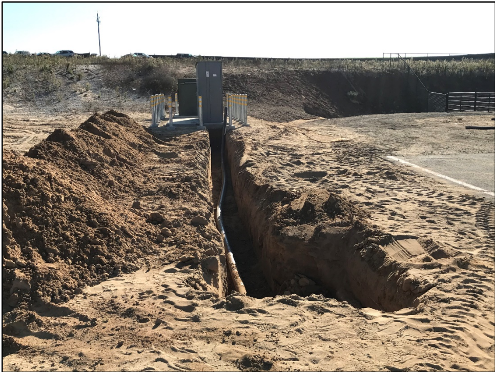
CTE / Ag Center - Conduit is Placed for Additional Power to Operate Machine Tools
