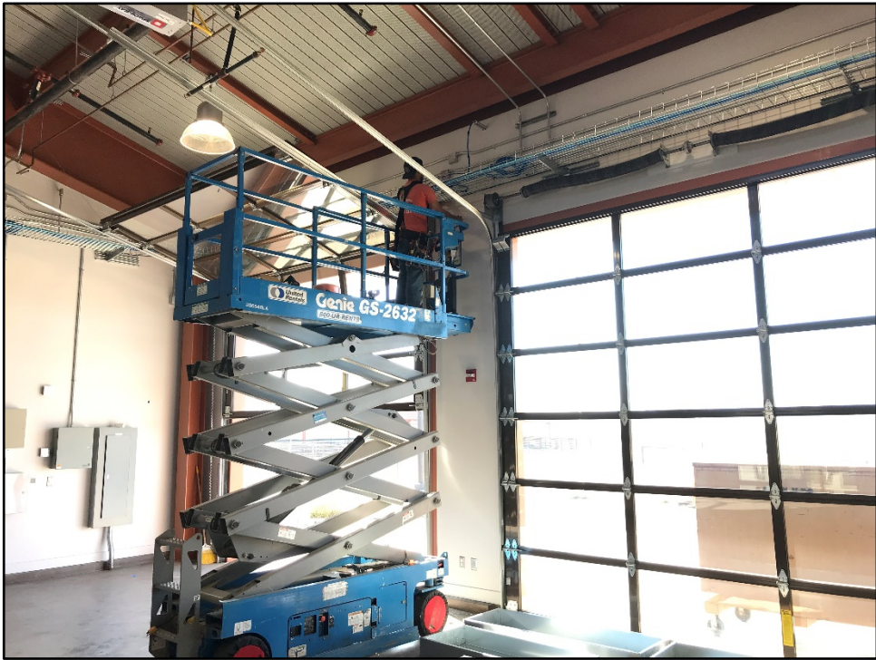
CTE / Ag Center – Instructor Public Address Speaker Installation In-progress
