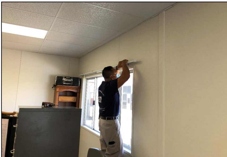
SMHS – Tim Lew Installs Window Coverings in New Portable Classrooms
