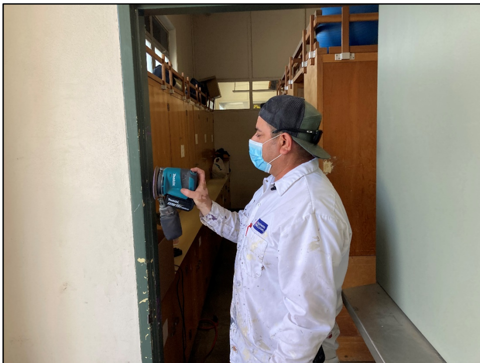
ERHS - Ernest Paz Prepares the Girls' Locker Room Doors for Paint
