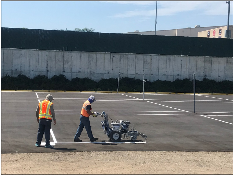
ERHS 2020 Paving – Final Striping for Volleyball Courts on the New Pavement
