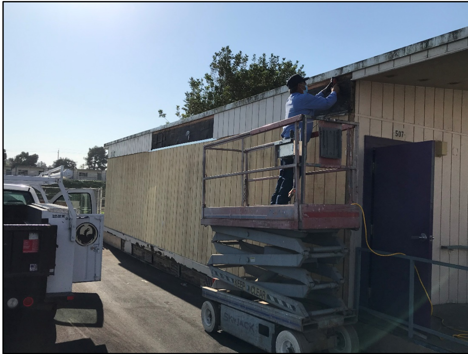
ERHS - José Placencia Replaces the Siding on Classroom 507
