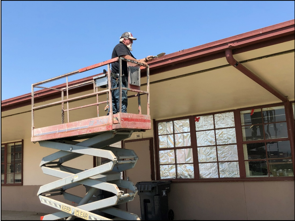
SMHS - Greg Matthews Clears Rain Gutters in the 360 Science Building
