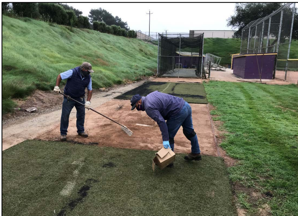
ERHS - Juan Rodriguez and Joseph Campos Install Artificial Turf in the Softball Pitchers' Bullpen
