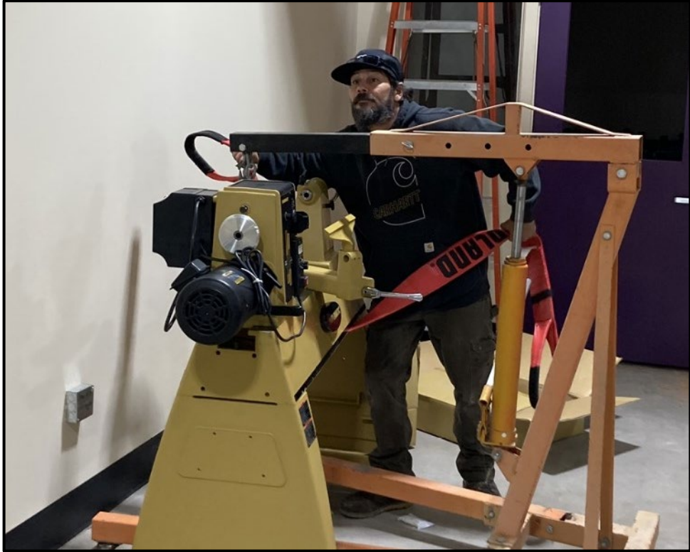
ERHS – Tom Harbold Installing New Equipment in the Woodshop
