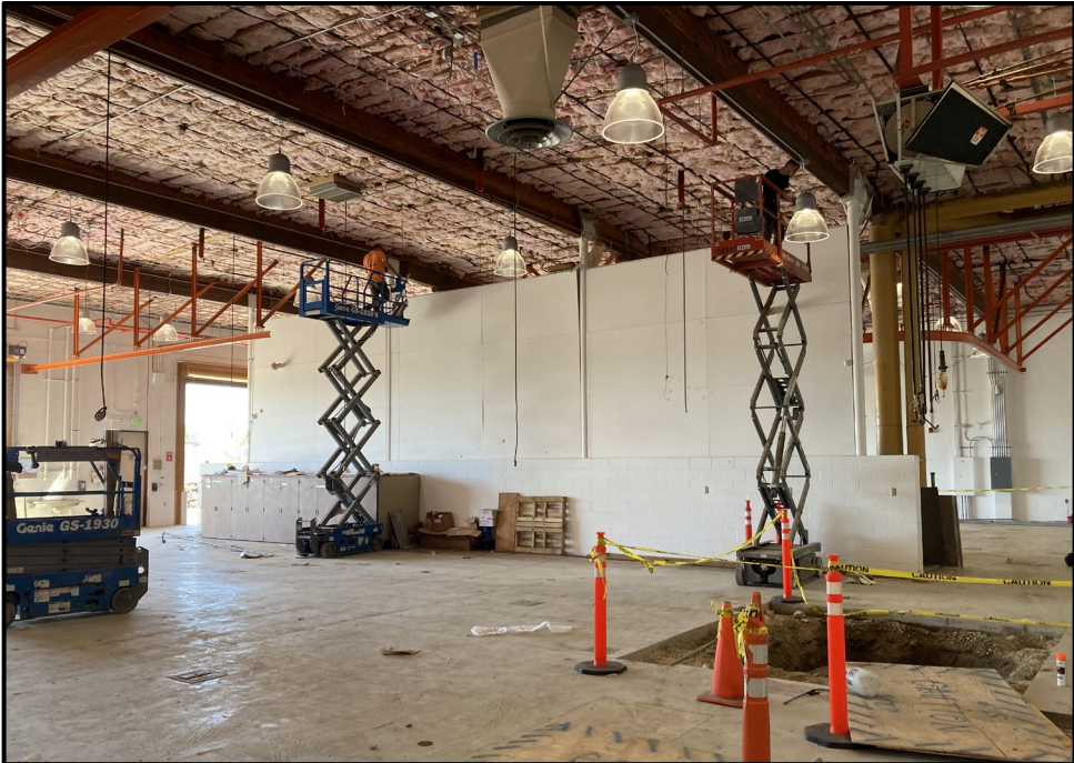
SMHS CTE Modernization – Installing Electrical in the Auto Shop
