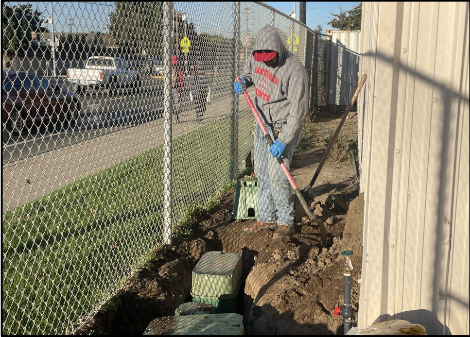
SMHS – Jordan Markstone Repairing a Broken Irrigation Valve
