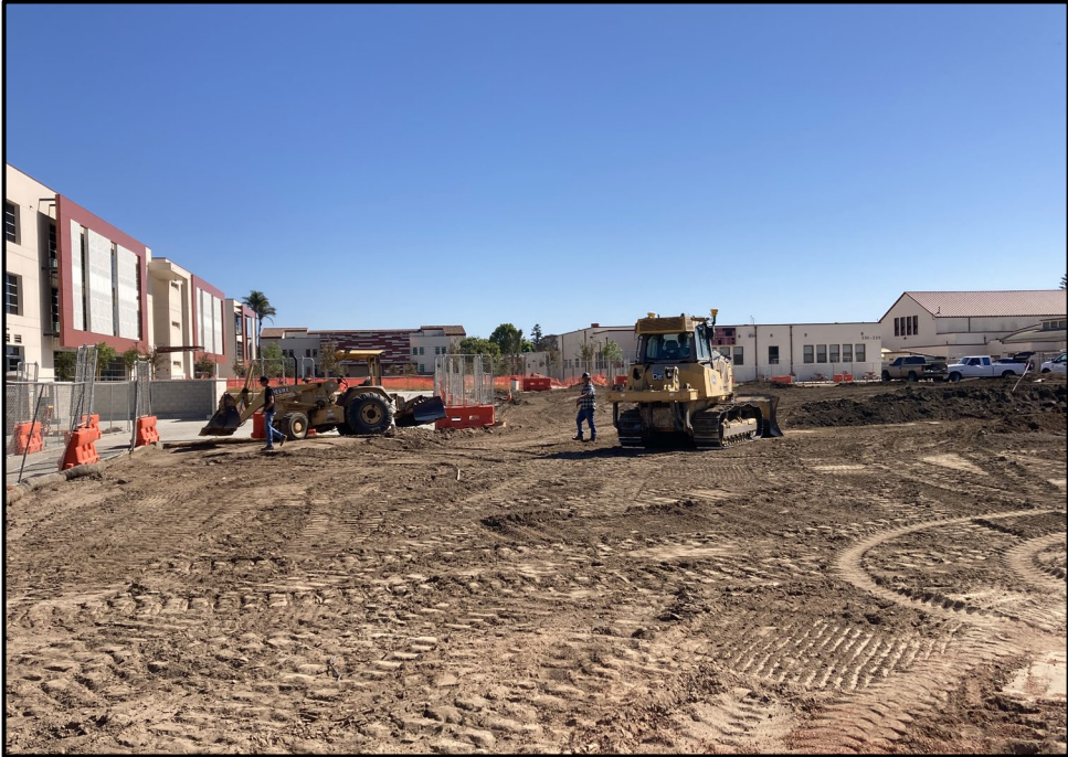
SMHS Softball Field – Grading the Softball Field
