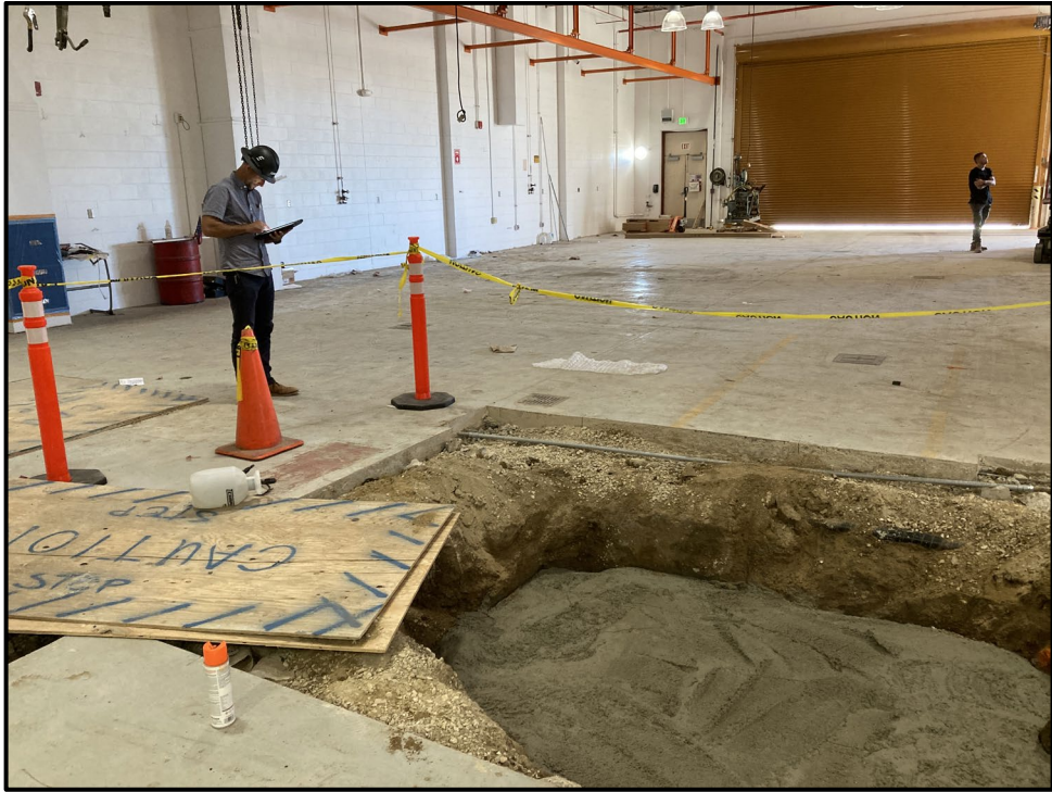
SMHS CTE Modernization – Inspecting the Concrete Backfill
