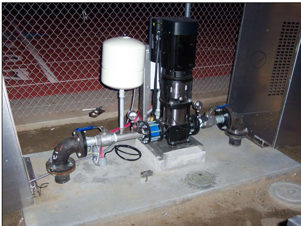
New irrigation booster pump at SMHS
