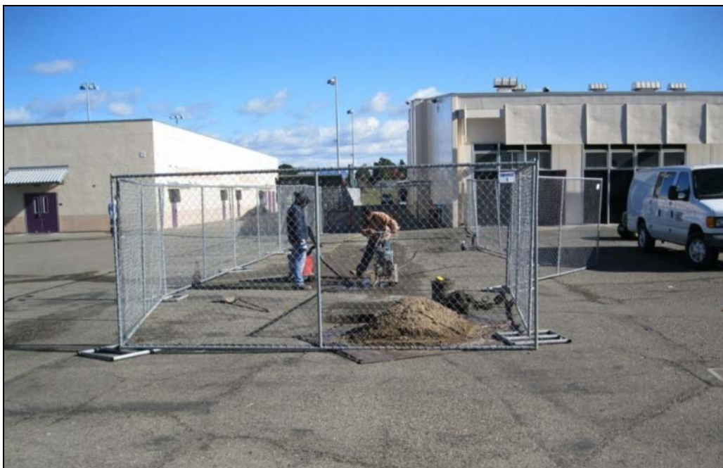
Replaced natural gas line at RHS Gymnasium
