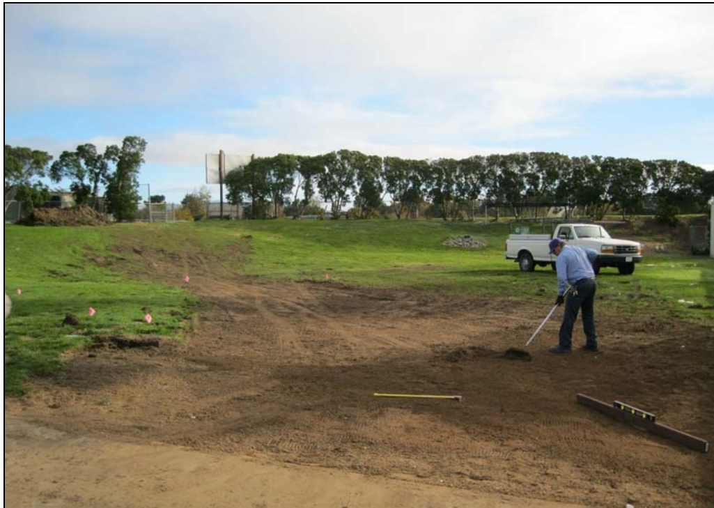
Improved drainage on the east end of the Righetti football stadium
