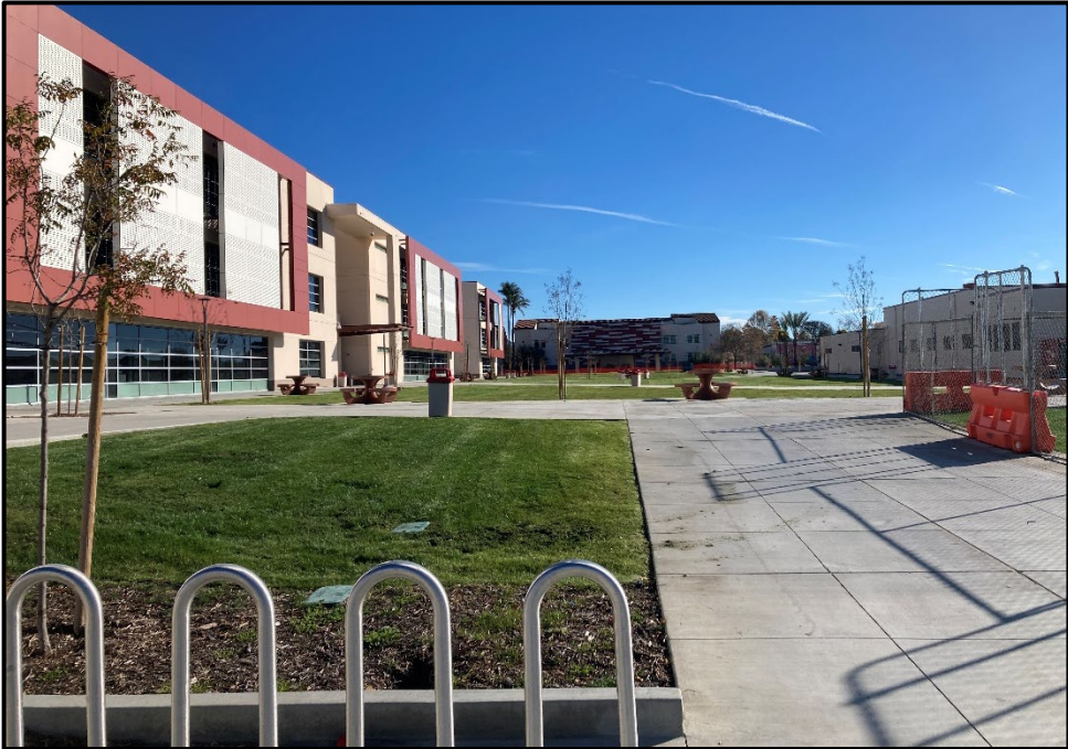
SMHS Reconstruction – Exterior Turf Fencing Removed and Accessible for Students
