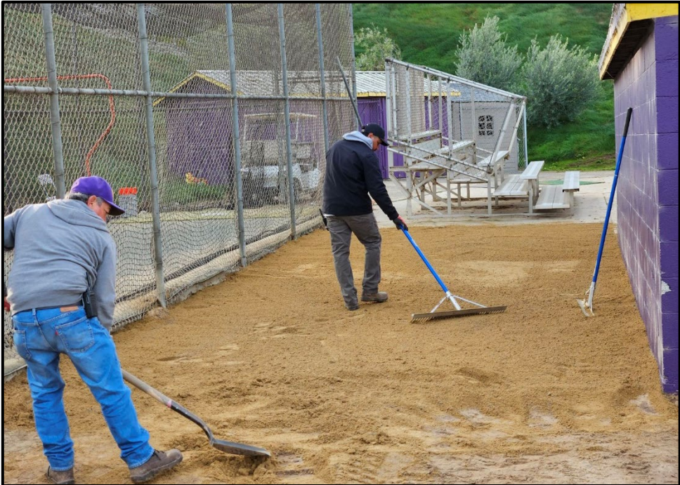
ERHS – Eric Escobar and Lorenzo Mendez Leveling Decomposed Granite Behind the Softball Dugout
