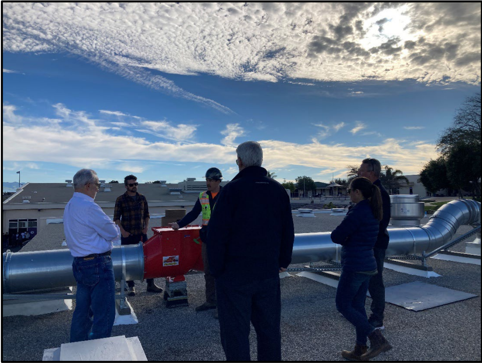
ERHS CTE Modernization – Reviewing Welding Shop Exhaust Ventilation
