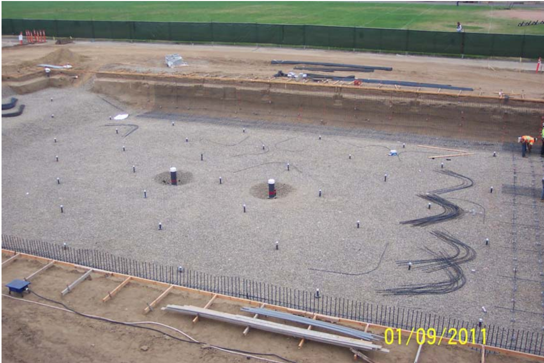
Santa Maria High Pool - Gravel Covering Water Pipes
