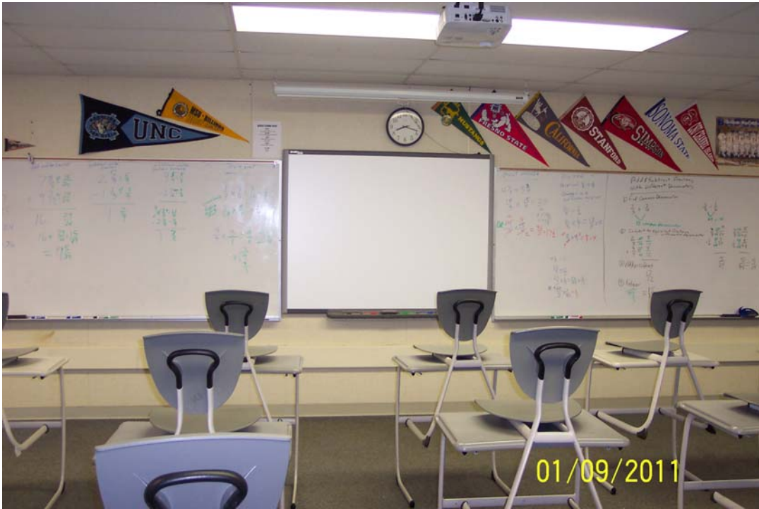
Typical New Smart board and Projector Installed
