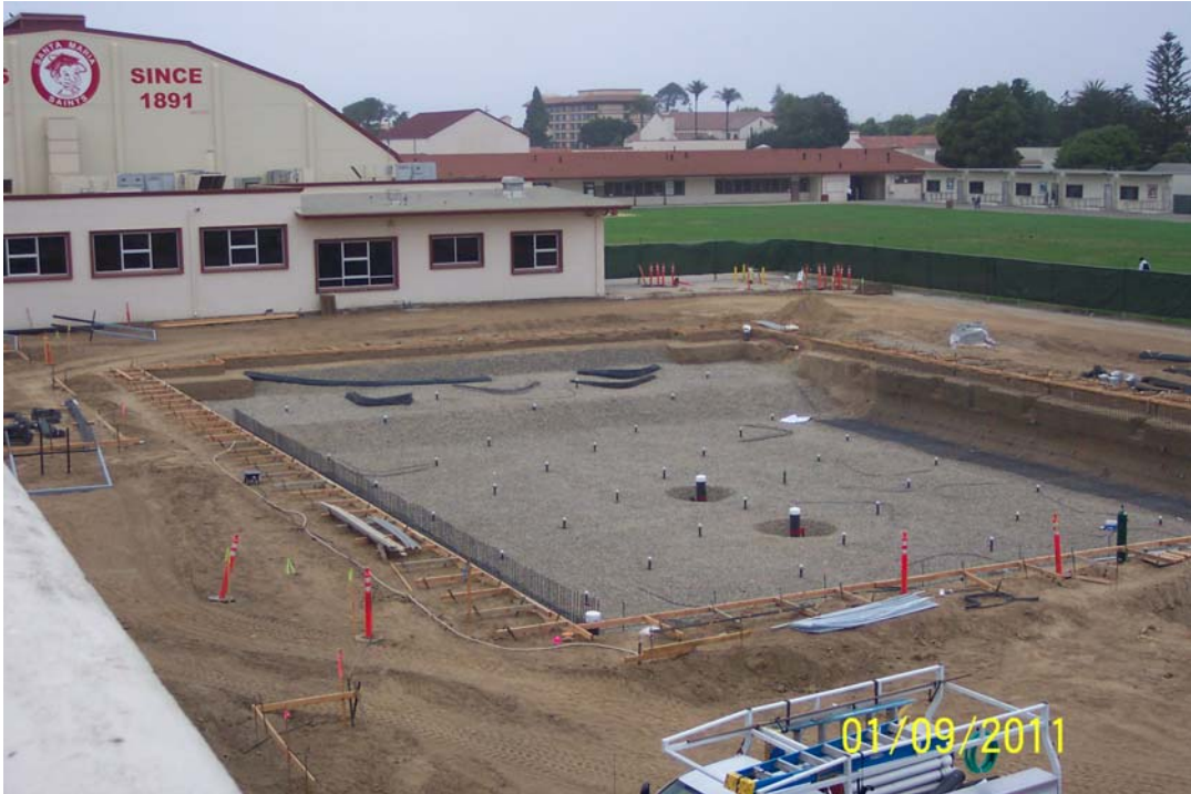
Santa Maria High Pool - August Progress
