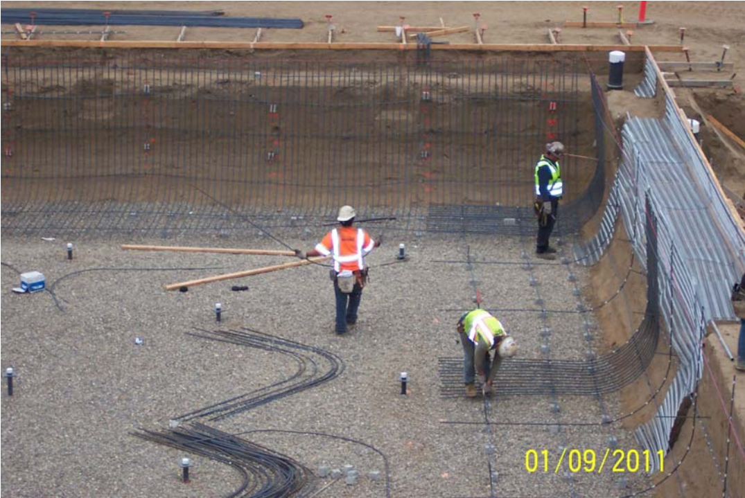
Santa Maria High Pool - Miles of Rebar to Bend, Place, and Tie
