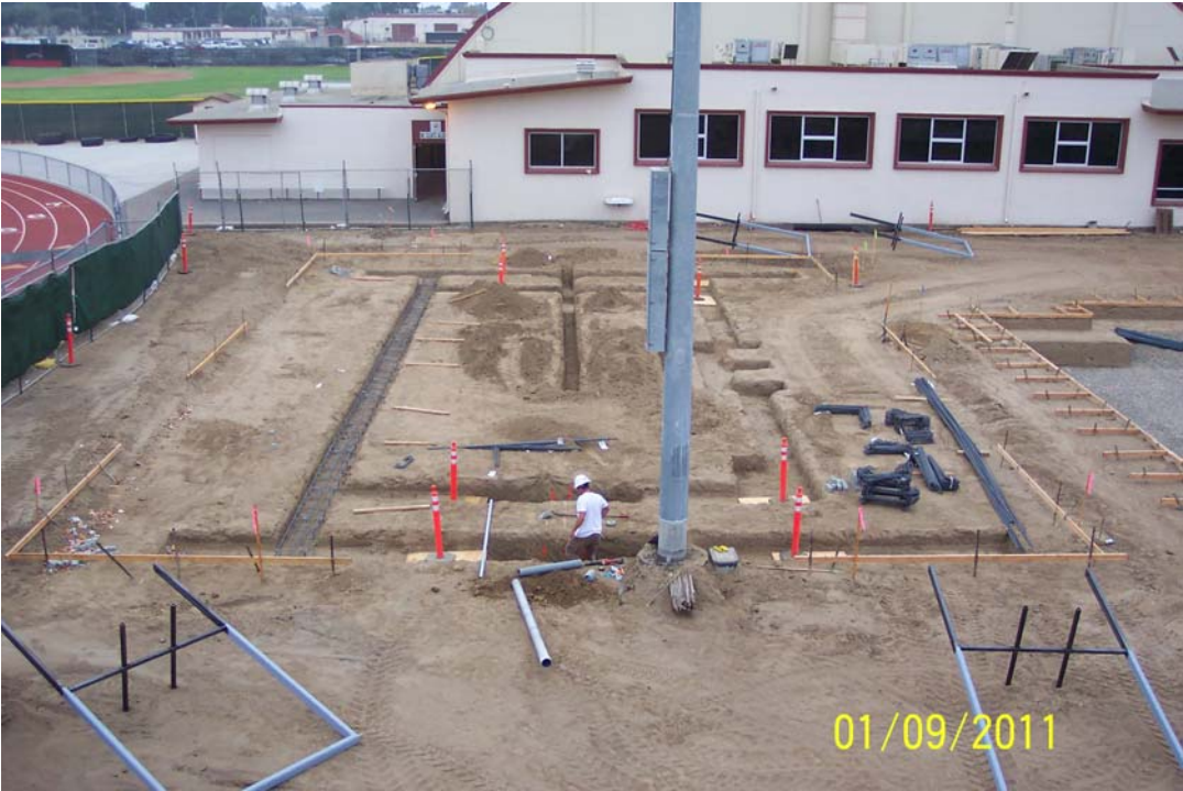
Santa Maria High Pool - Restroom and Snack Bar Footings
