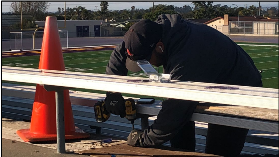
ERHS – Jordan Markstone Repairing the Bleachers in the Stadium
