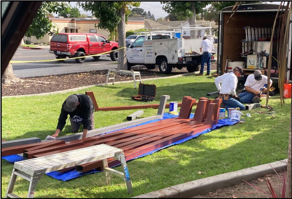
SMHS – Replacing Administration Building Rain Gutters and Downspouts
