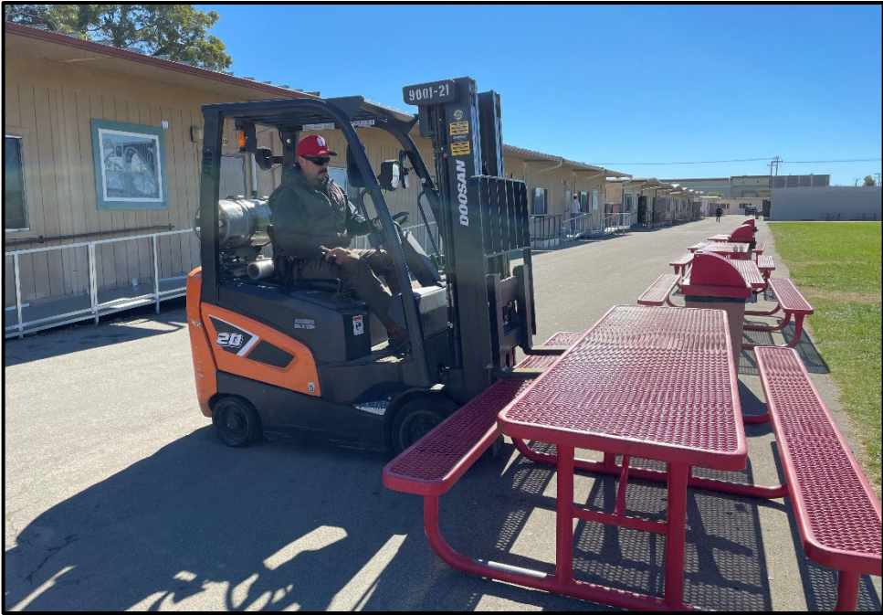
SMHS – Alan Rodriguez Removing the Old Tables in Preparation for New Concrete Lunch Tables
