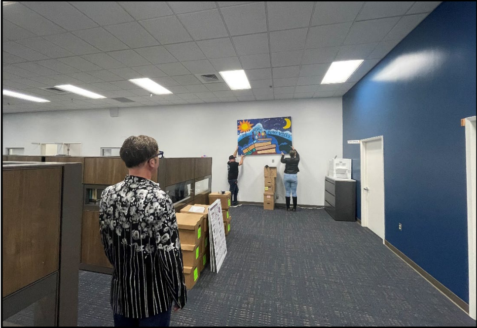
SSC Front Office Renovation – Designing the Wall Space in the Front Office
