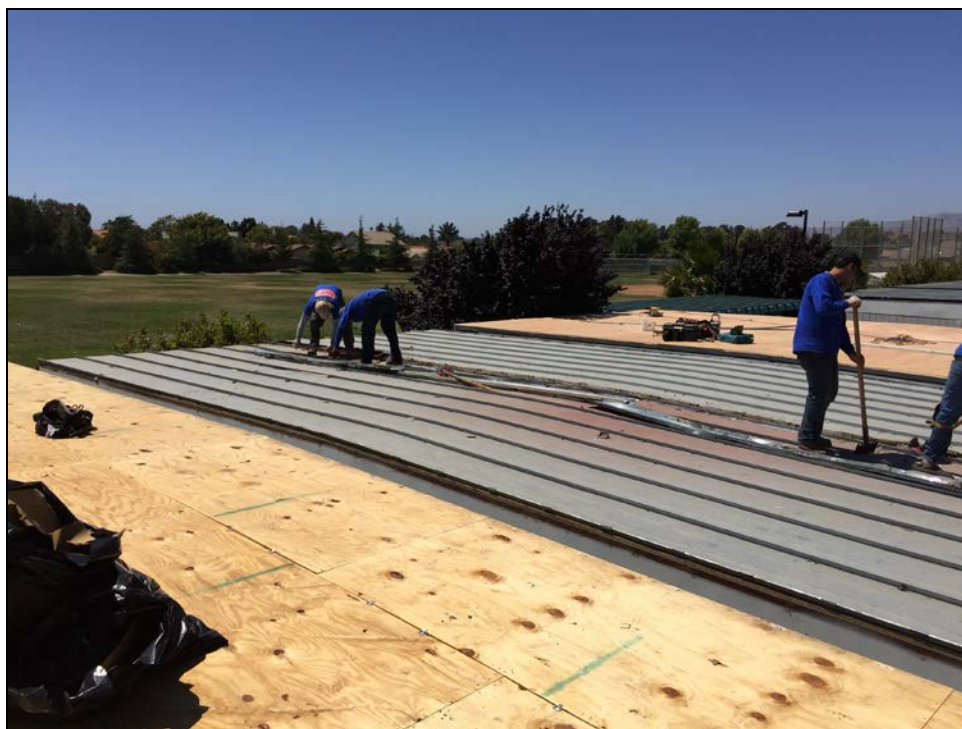
PVHS – Roof Replacement Underway on Six Portable Classrooms
