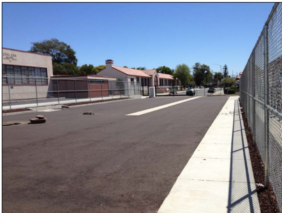
SMHS – Camino Colegio Parking Lot Paving Receives Final Details
