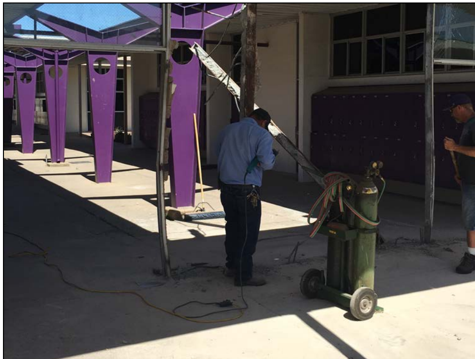
ERHS – José Placencia and Denton Tilley Remove the Block Walls that Restricted Student Flow and Supervision
