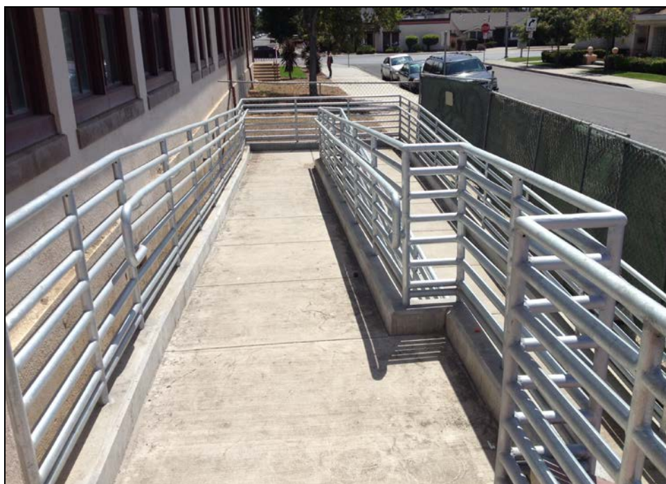
SMHS – Camino Colegio Parking Lot Required a New ADA Ramp to the Front Entrance
