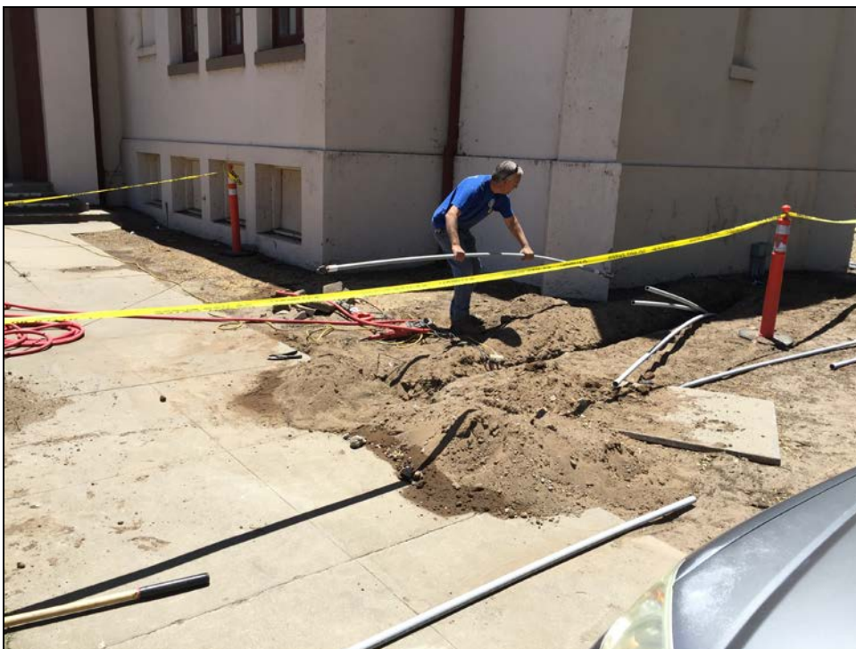
SMHS – Del Ward Installs Conduit to Communicate with the New Marquee
