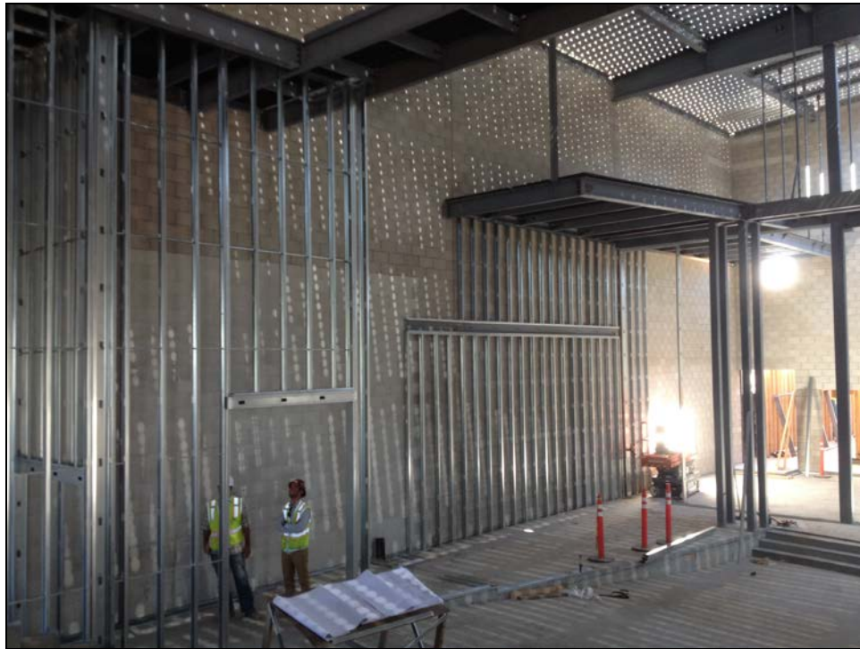
PVHS – Theater Interior Walls and Roof Decking in Progress
