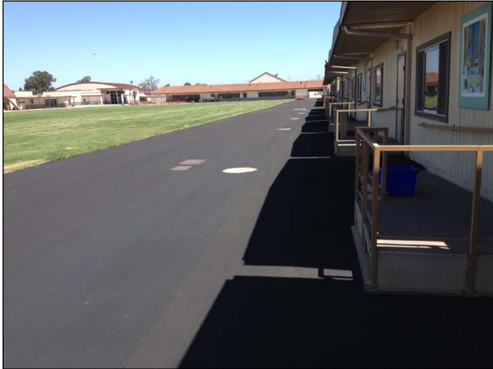
SMHS - New Asphalt Slurry Seal for Student Walkway
