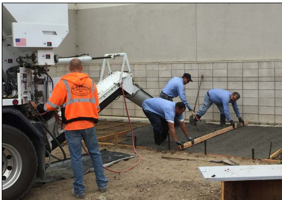
PVHS – Concrete for the School Garden Storage Unit is Poured
