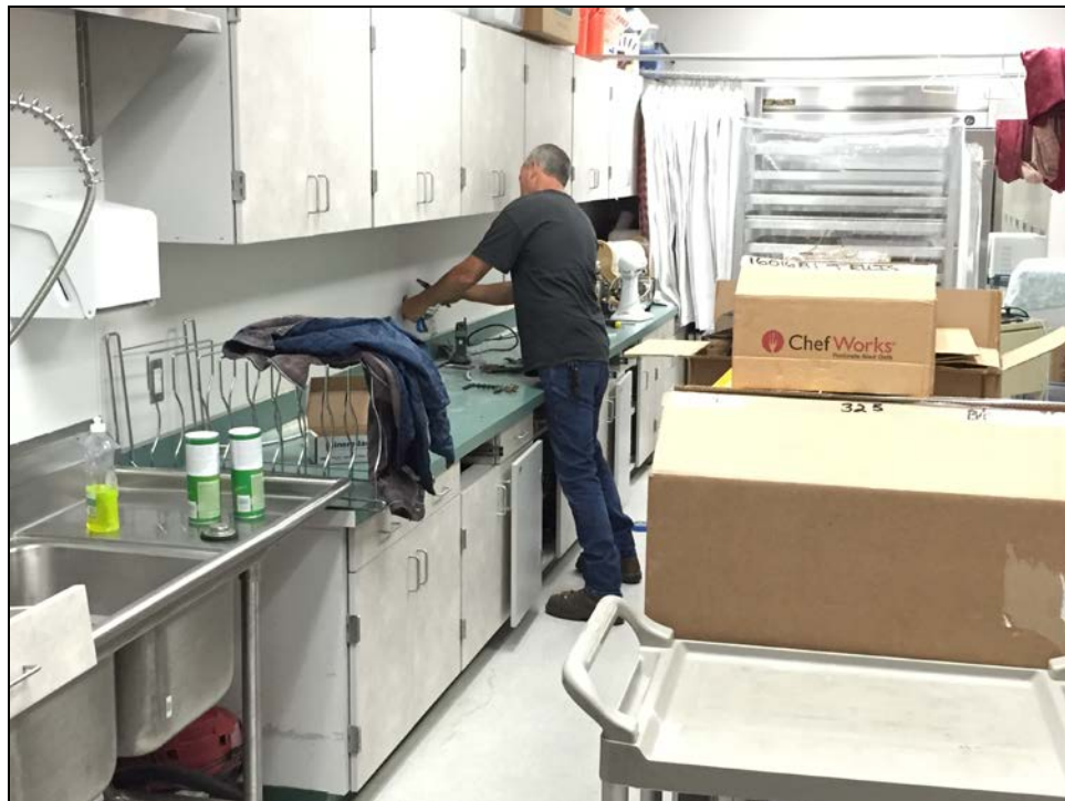
PVHS - Del Ward Installs New Electrical Outlets in the Foods Lab
