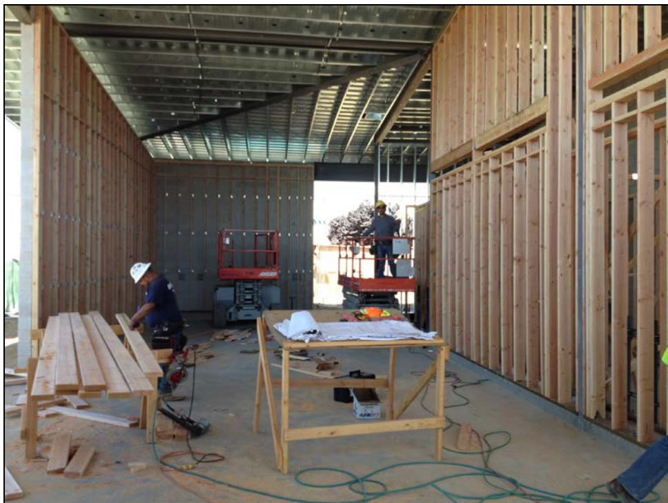
PVHS - Performing Arts Center Lobby Interior Begins to Take Shape
