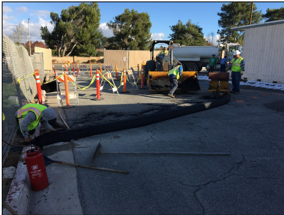
ERHS – Emergency Repairs are Completed due to Rain Damaged Bradley Parking Lot
