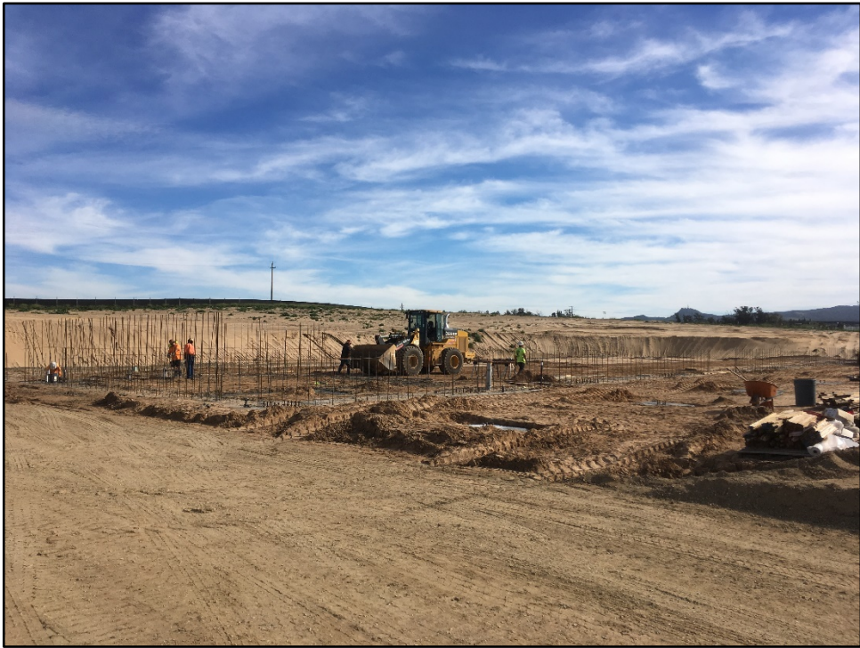
CTE Ag Center – Barn Footings are Prepared for Concrete with Rebar
