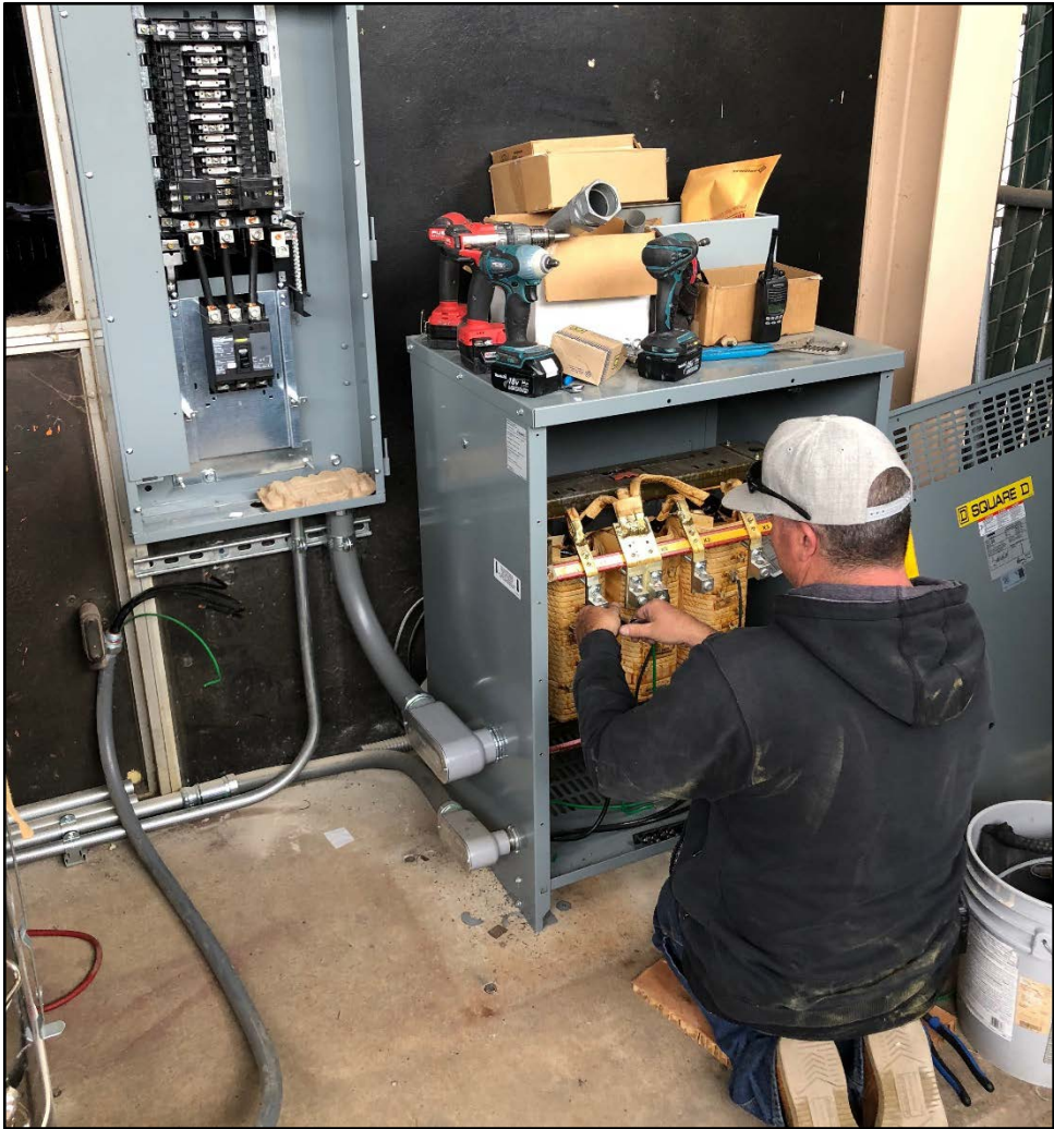
ERHS – Andy Freitas Connects Power to the Art Kilns
