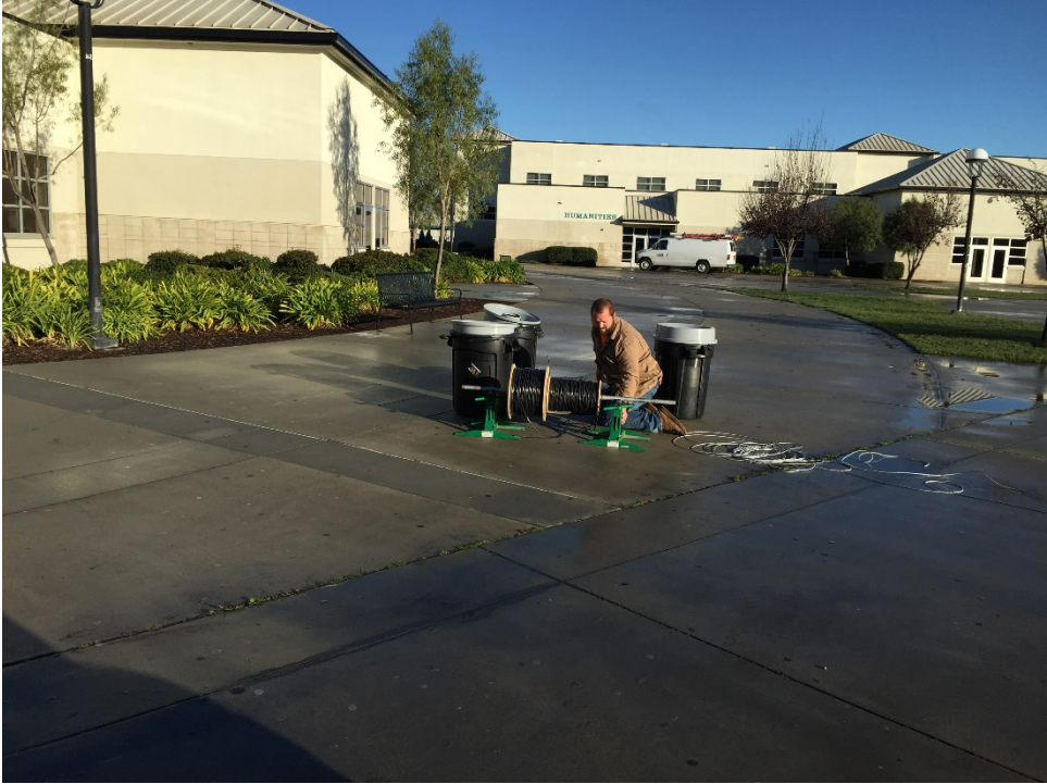
PVHS - Fire Alarm Wiring Replaced to Reduce False Alarms
