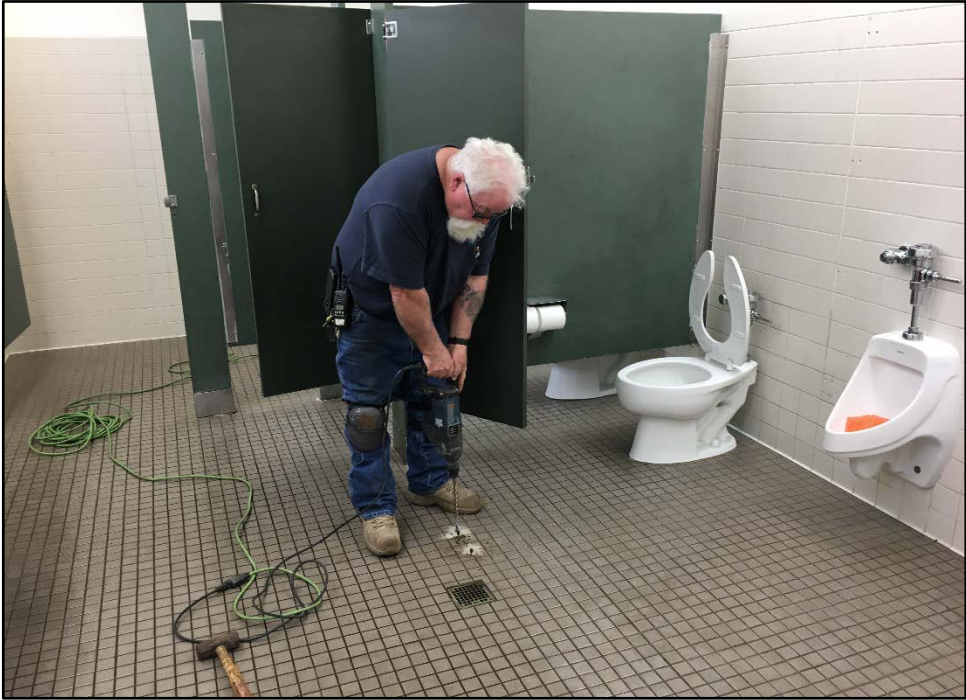
SMHS – Rain Greg Matthews Replaces a damaged Partition Pilaster in 320 Boys' Restroom
