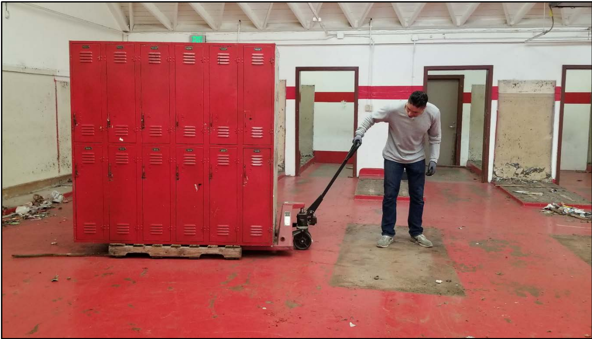
SMHS - Joel Amezcua Removes a Bank of Old Lockers and Hidden Trash
