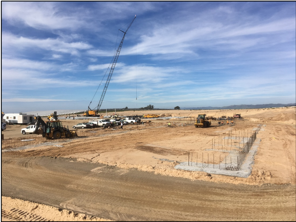
CTE Ag Center – Excavation for the Barn Foundation Footings is in Progress
