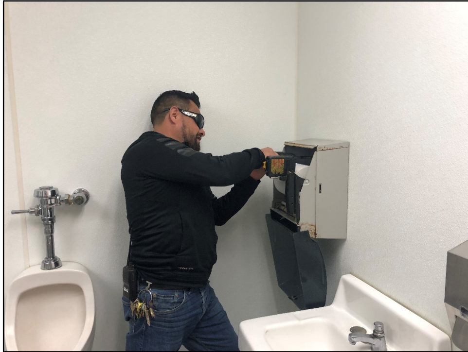
ERHS – Leo Avila Repairs Damaged Restroom Equipment in the Press Box Boys’ Restroom
