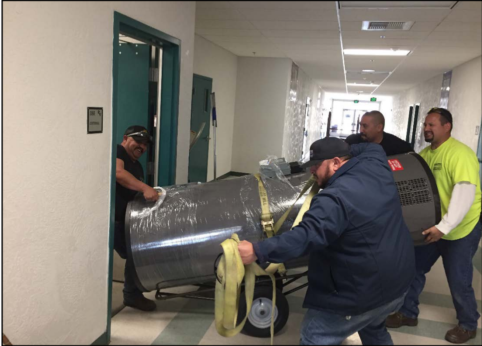
PVHS – Plumber and PVHS Maintenance Crew Position the Heat Pump Water Heater for the Foods Lab
