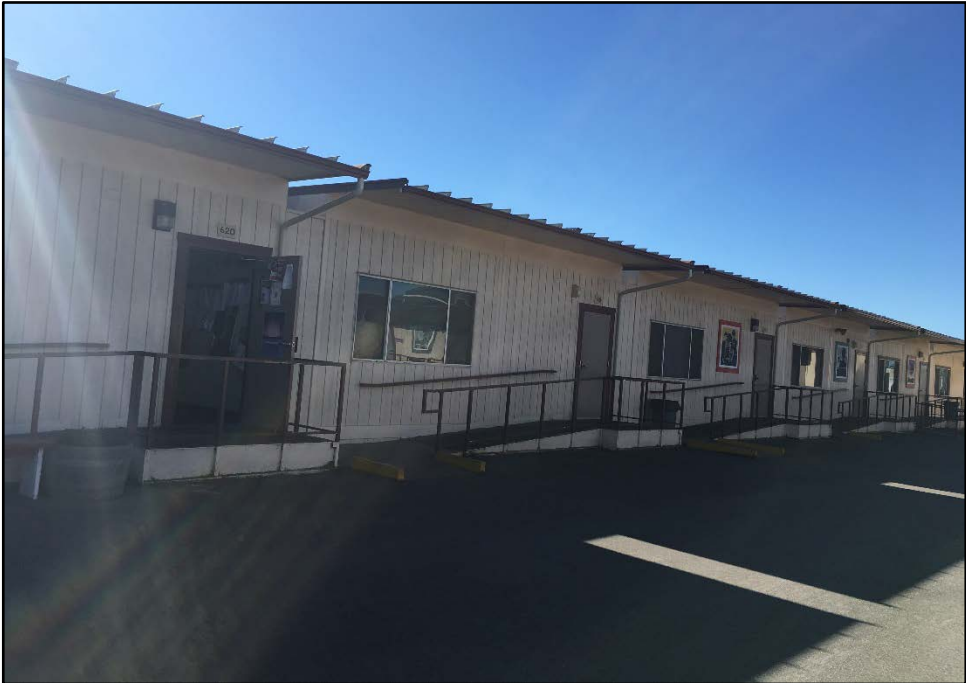
SMHS – Rain gutters and down spouts are replaced on Thirteen Portable Classrooms
