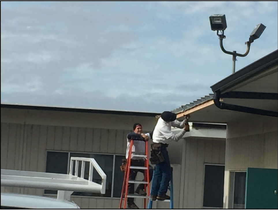
PVHS - New Rain Gutters and Downspouts are Installed on Fourteen Portable Classrooms
