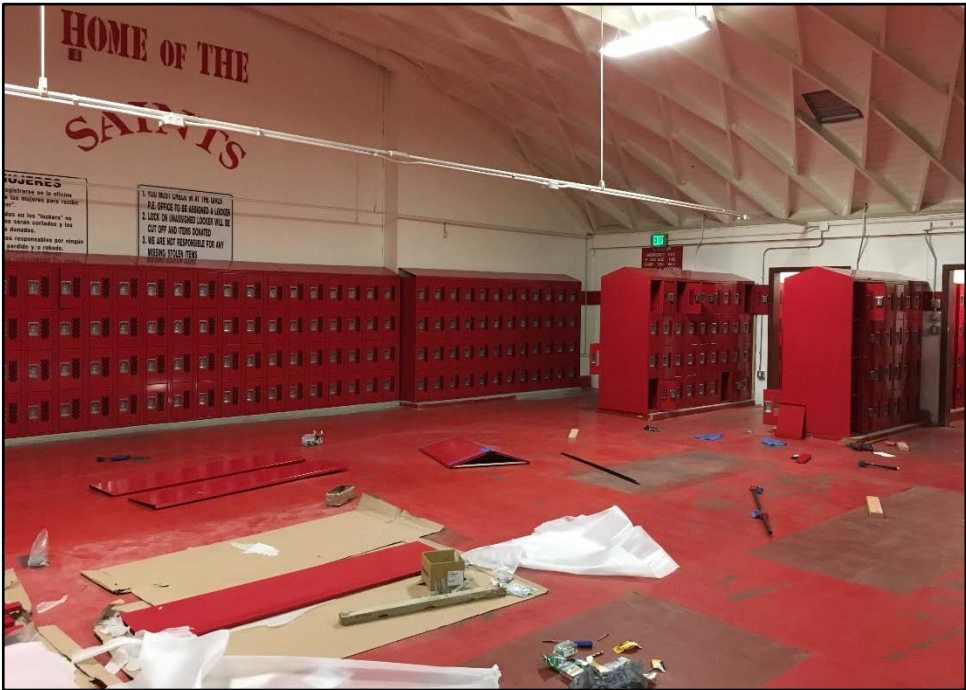
SMHS - New Locker Installation In-progress in the Girls' Locker Room
