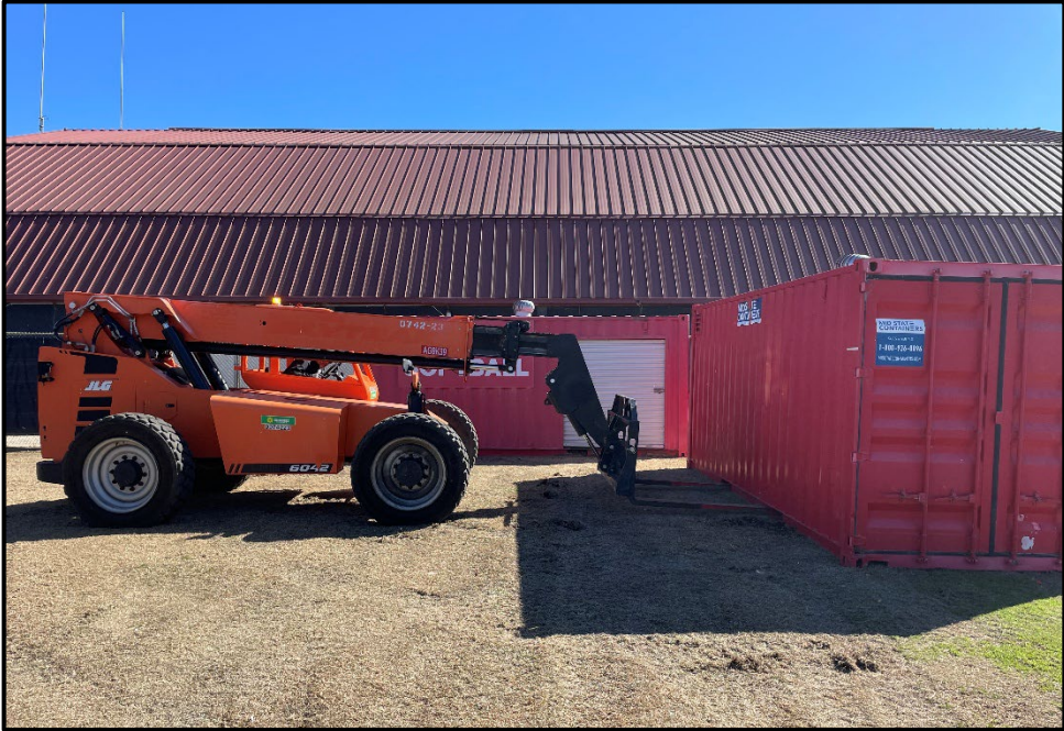
SMHS – Relocating PE Storage Containers
