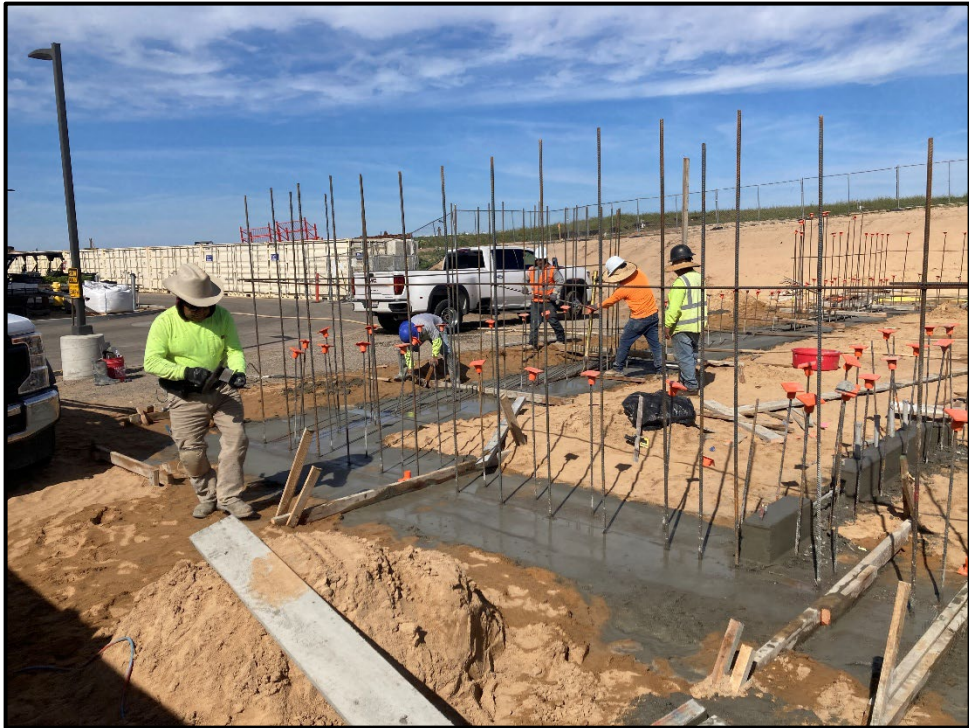
MRCTECAF M&O Building – Foundation Finishes Being Poured
