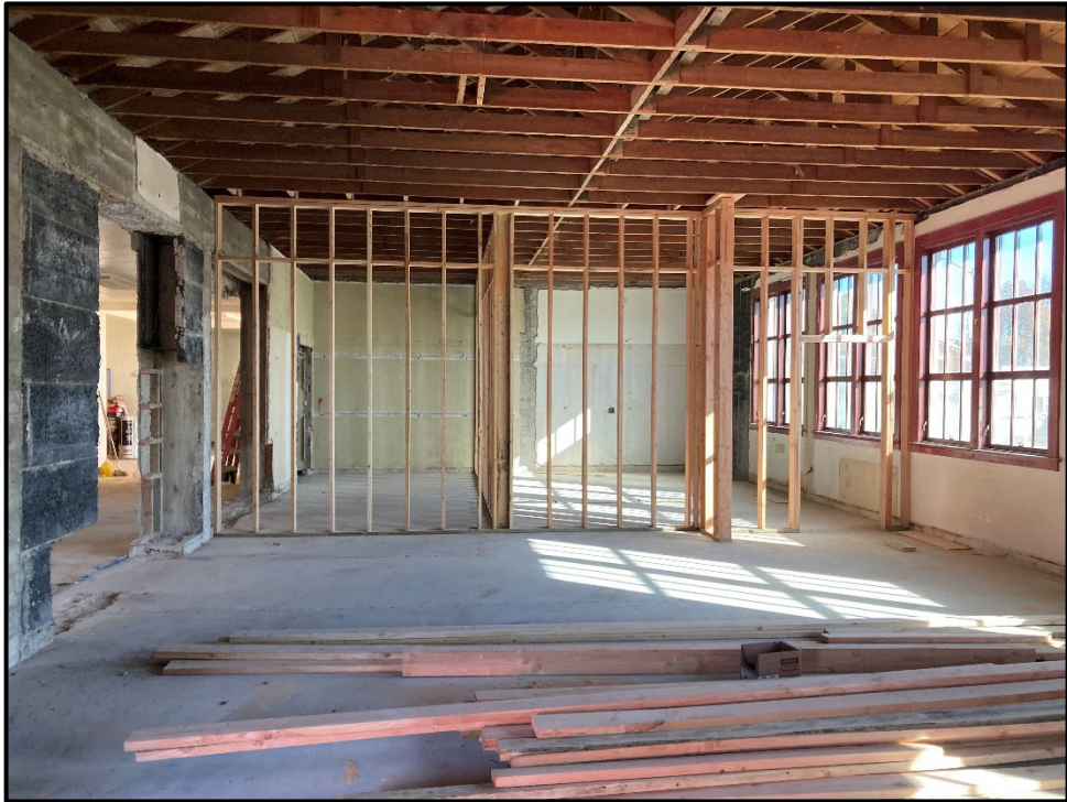
SMHS Admin to Classroom – Framing of New Classrooms Begins
