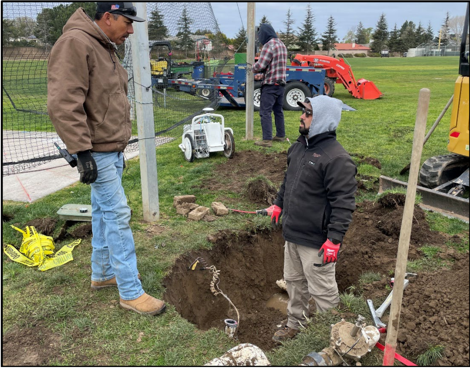
PVHS – Jose Gamino and Ricardo Eliserio Replacing a Water Valve
