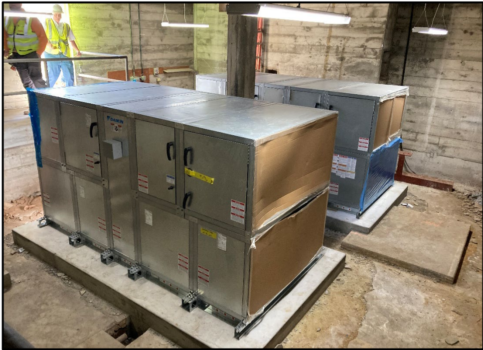
SMHS Admin to Classroom – New Ventilation Units Being Installed
