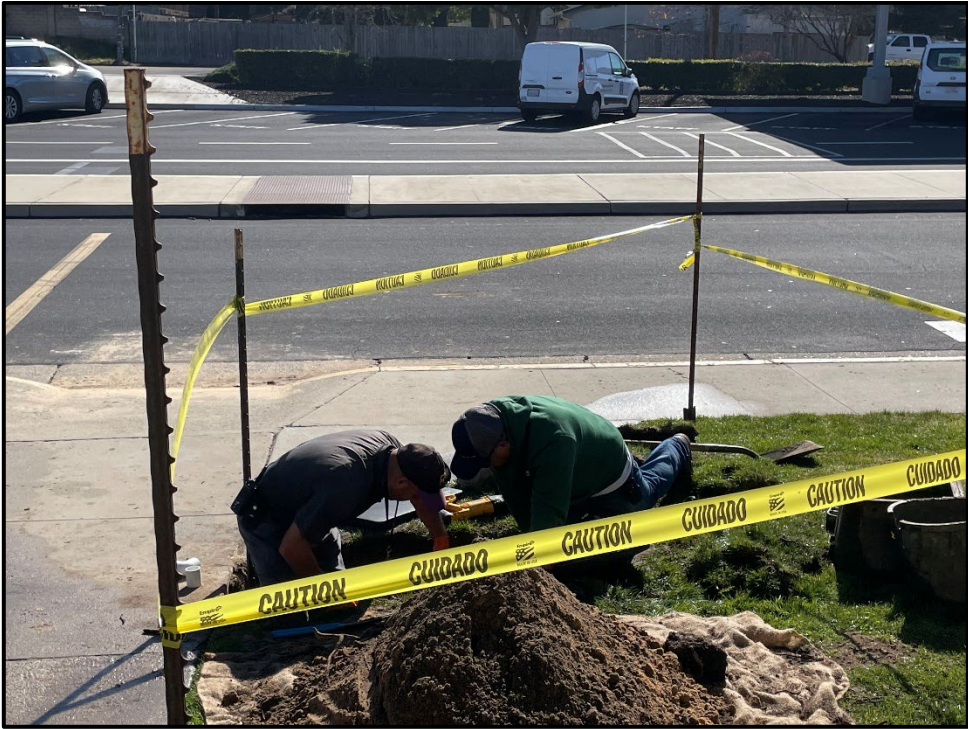
ERHS – Jose Gamino and Erick Escobar Repairing and Irrigation Leak
