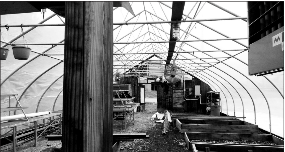
Greenhouse under repair
