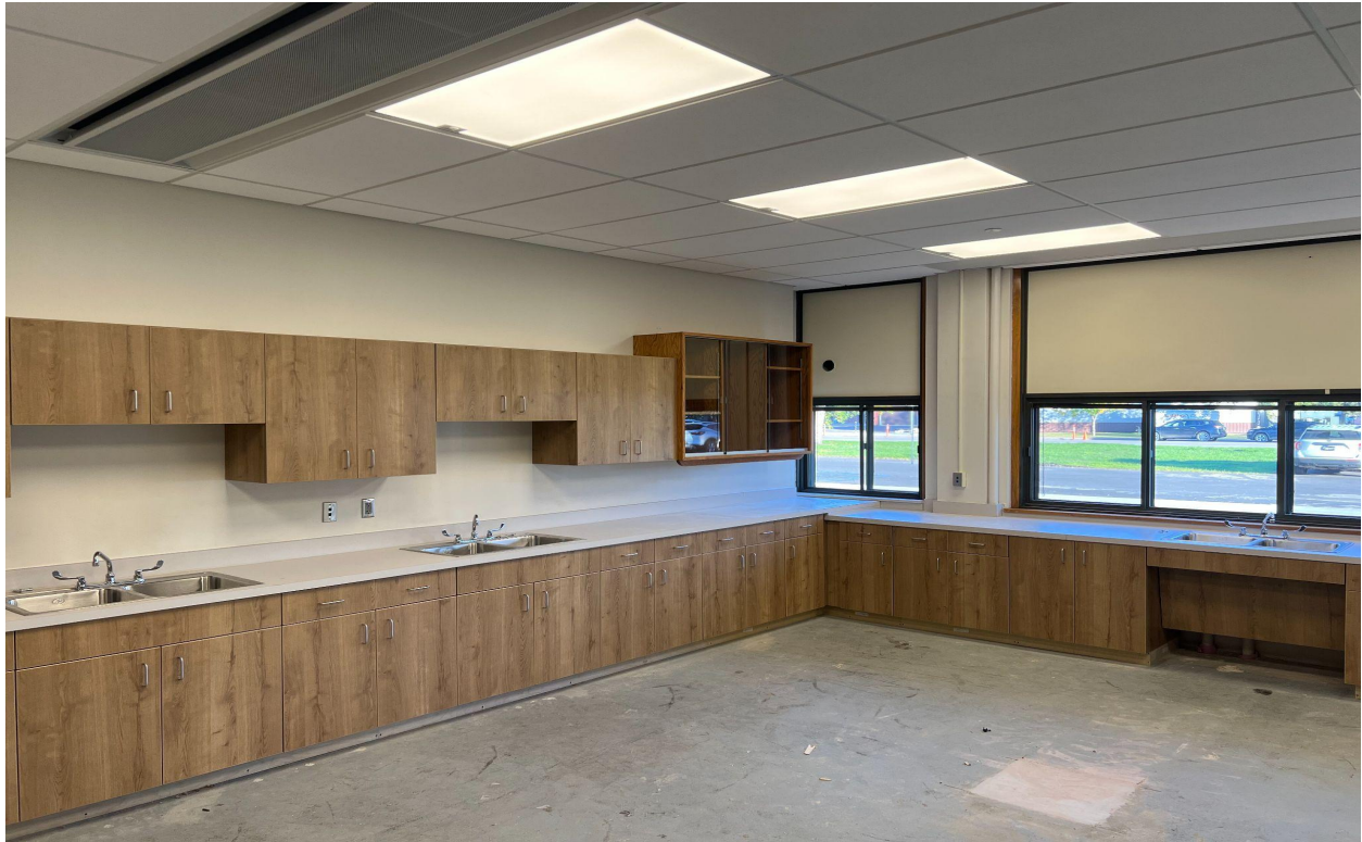
Progress in the HS science classrooms
