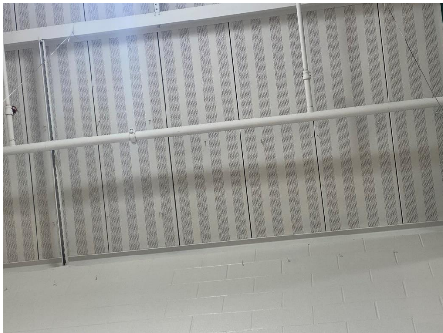
Photo 6: Variations in clip spacing and single screws
