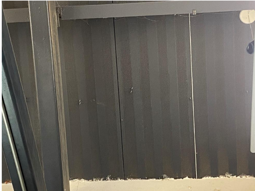
Photo 1: Variations in screw spacing, some at perforated deck sections
