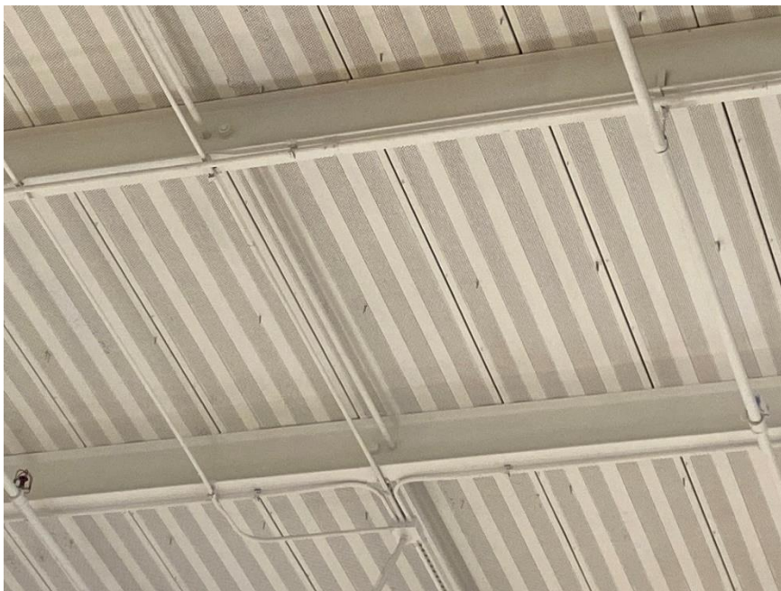
Photo 2: Line of single screws at gymnasium
