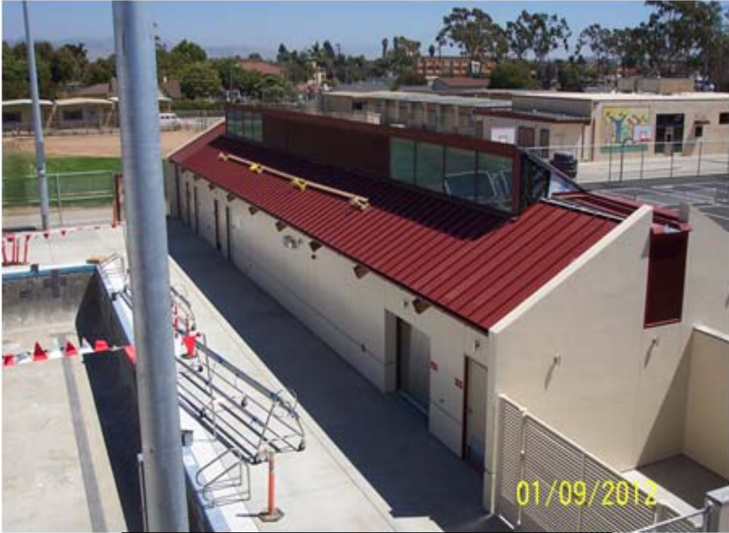
SMHS –Pool Construction Continued
