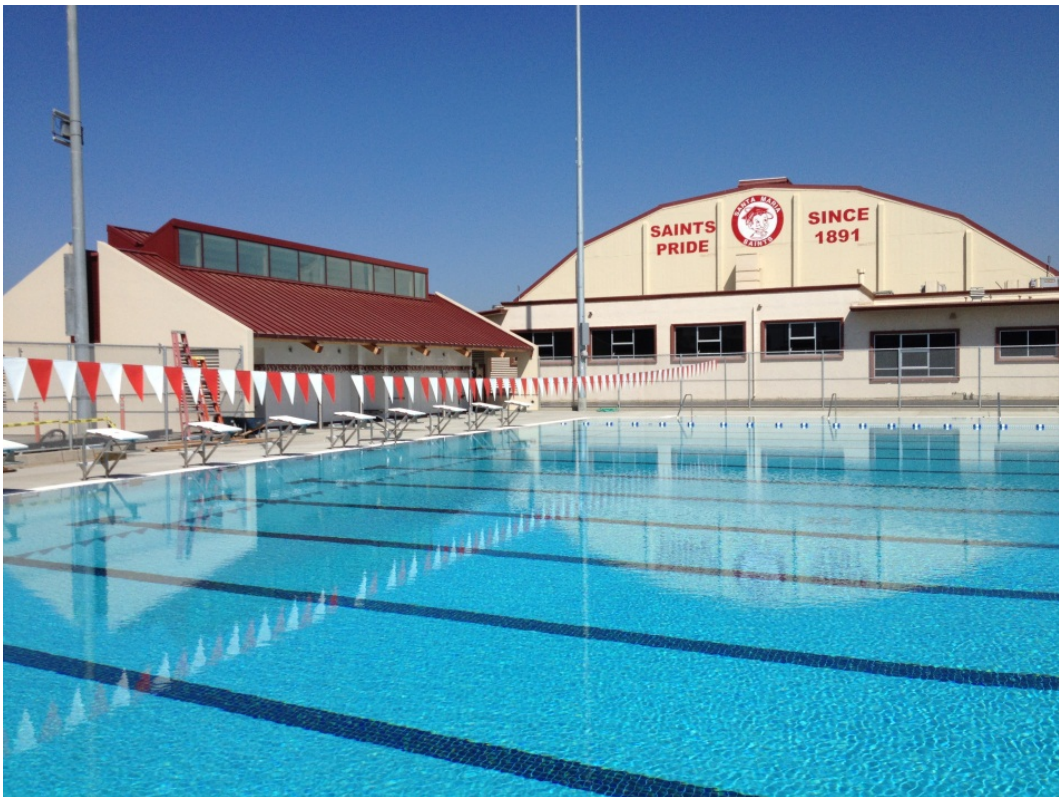
SMHS –Pool After Final Construction Complete
