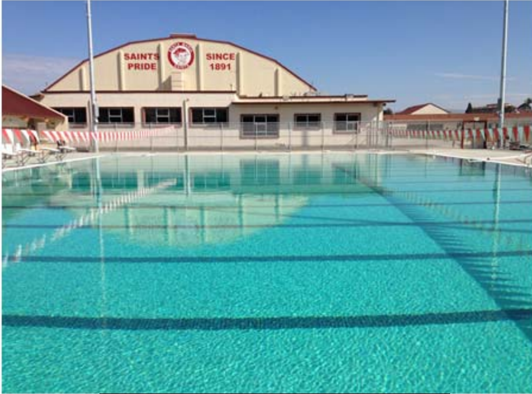
SMHS –Pool Construction Continued
