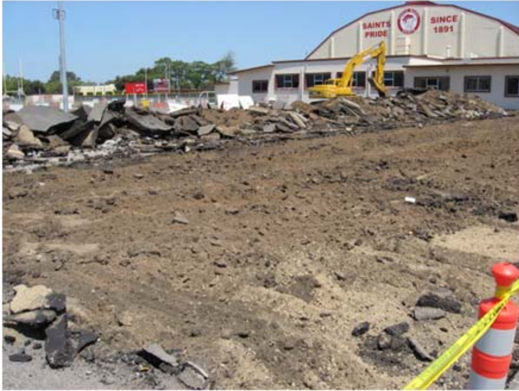
SMHS – Initial Pool Construction
