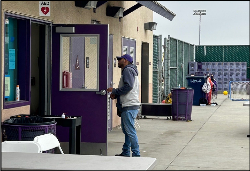
ERHS – Armando Guterrez Repairing the Doors at the Pool Office
