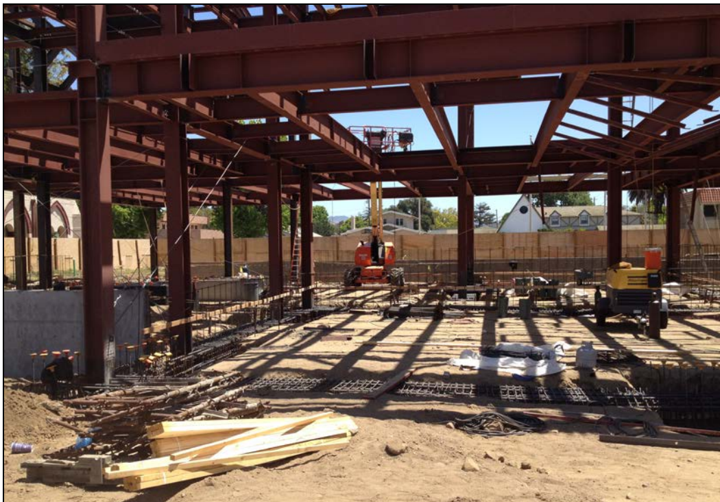
SMHS - 14 Classroom Building Band Room Before it has a Floor
