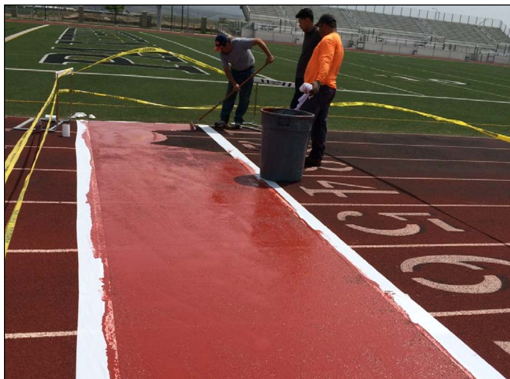
PVHS – Track Repair Underway
