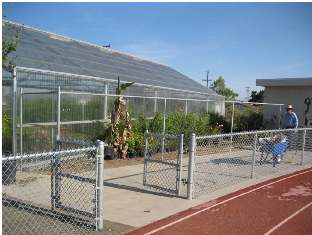
ERHS – Juan Rodriguez Builds a New Fence Between the Stadium and the Greenhouse
