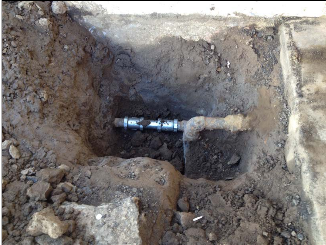
SMHS – Glamorous Plumbing Repair at the Old JC Building
