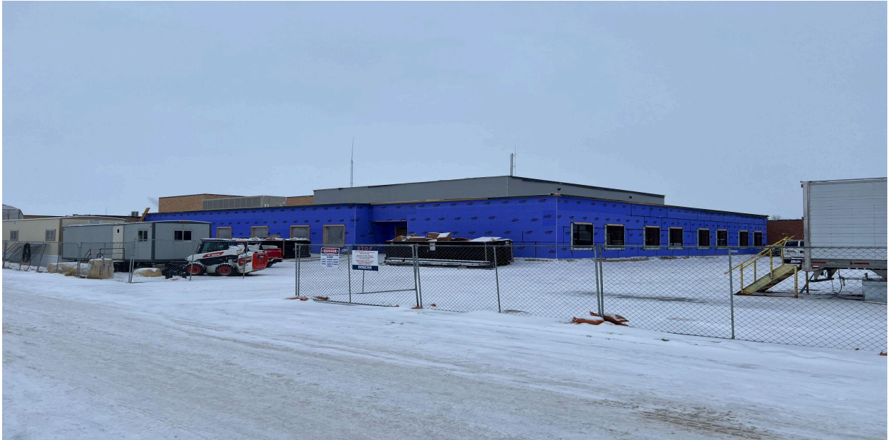
South side of the new addition.
