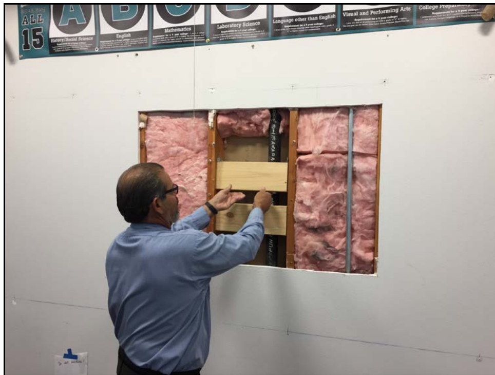
PVHS – José Placencia Fits Support Blocking for an Interactive Flat Panel Monitor
