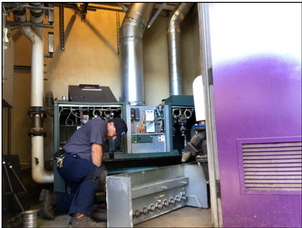
ERHS - Bernie Rayner Services the Hydronic Heater Burners
