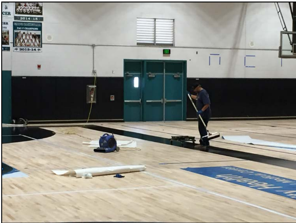
PVHS – Gymnasium Floor Receives New Lines and Lettering
