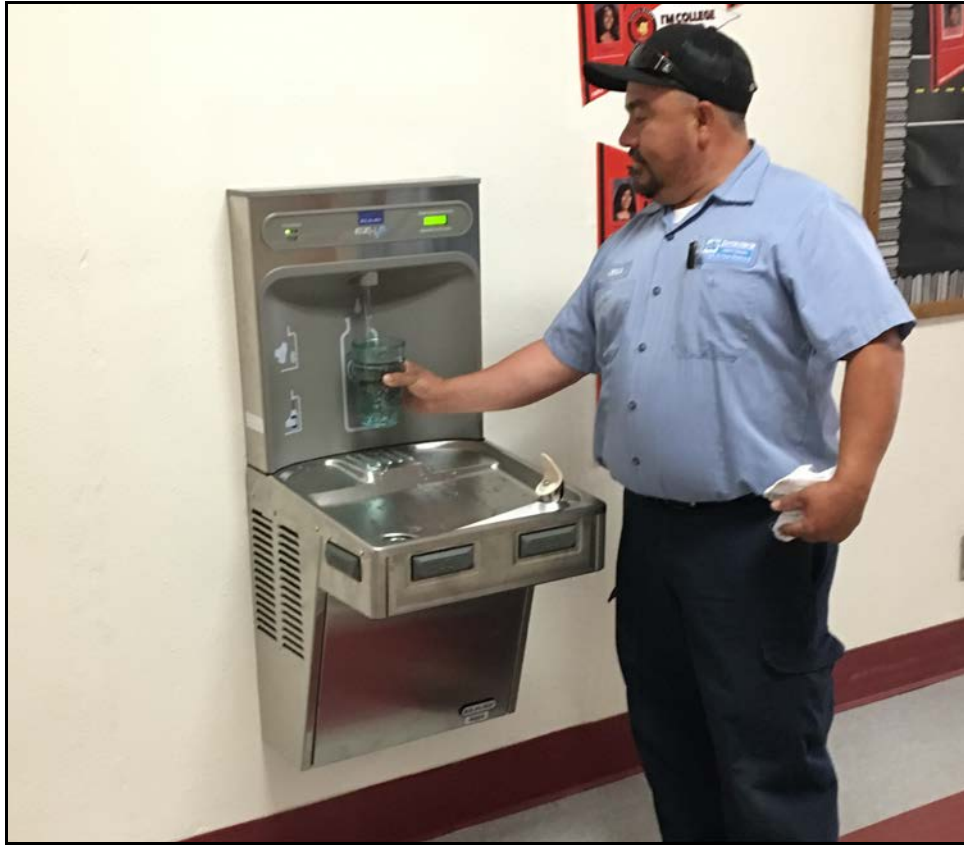
SMHS - Plumber Jesus Reyes Checks the New Hydration Station
