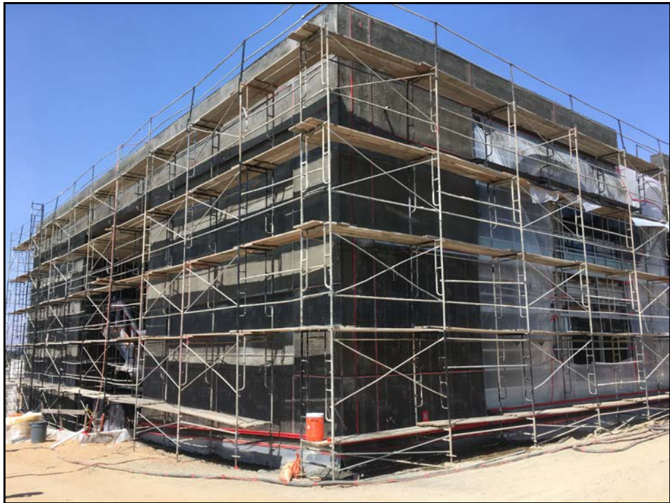
ERHS 38-Classroom Building – Scaffolding In Place and Exterior Plaster Underway
