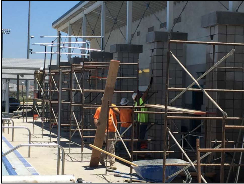
PVHS Pool Lighting – Pool Building Column Repair Completes the Original Project
