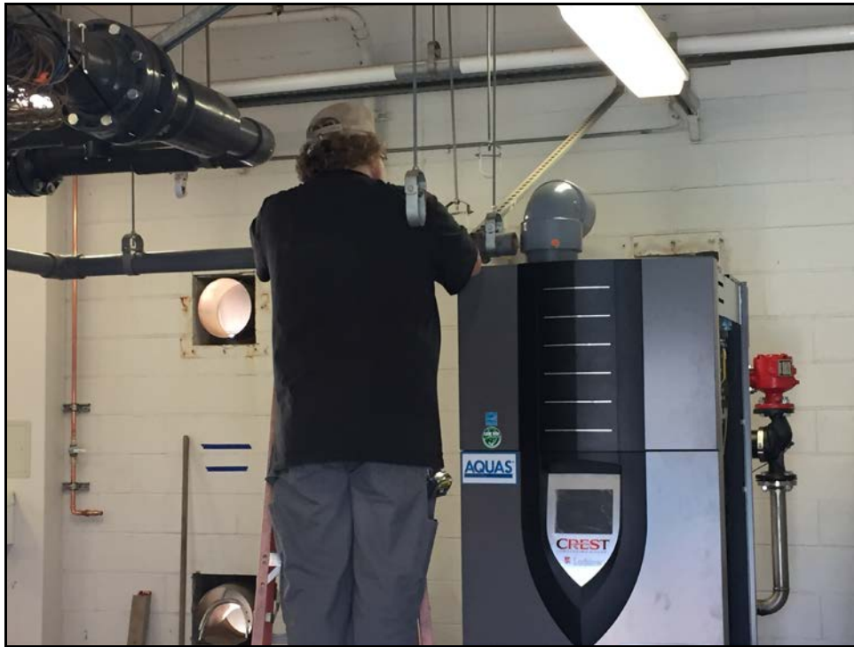
Proposition 39 - PVHS High Efficiency Pool Heater Installation
