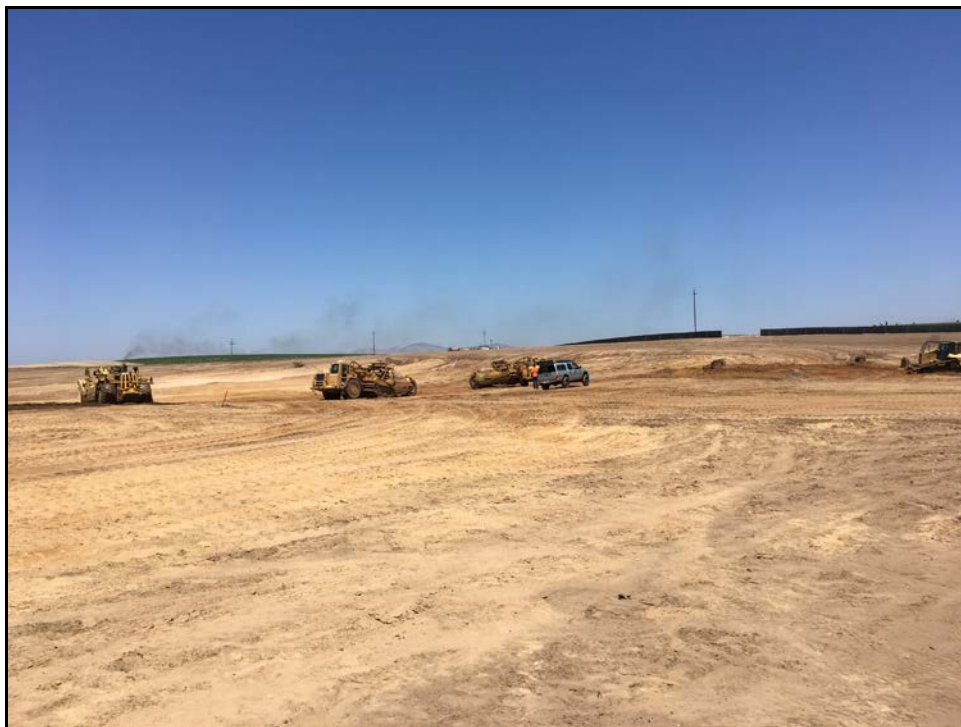
CTE Ag Center - Scrapers Move Thousands of Yards of Earth to Form the Building Pads
