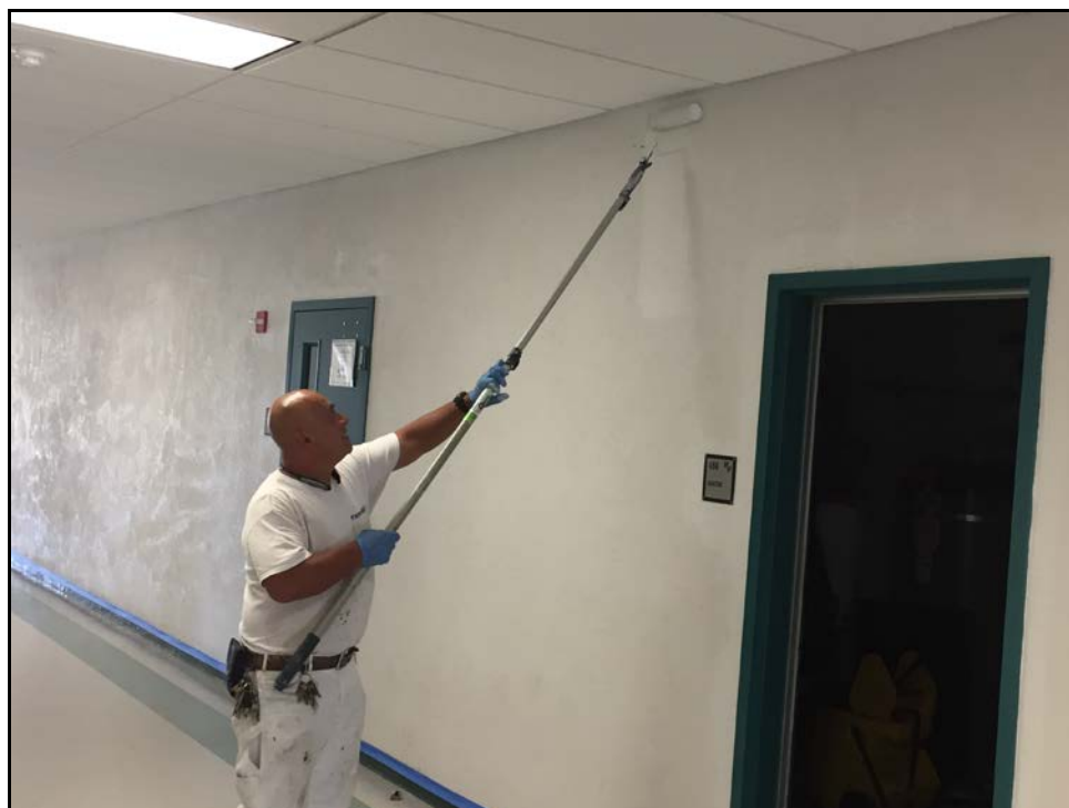
PVHS – Ray Segovia Repainting the Interior Hallway of the 400 Building
