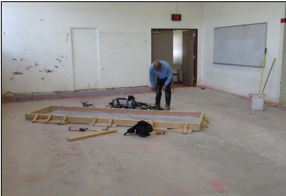
SMHS – José Placencia Builds Concrete Forms for Locker Curbs in the Boys' Locker Room
