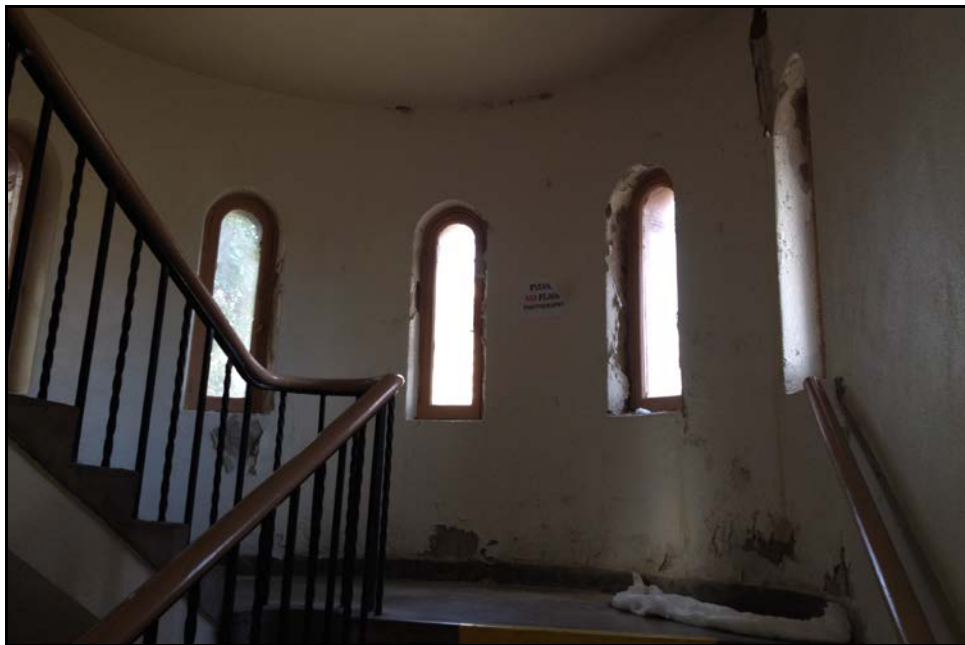
SMHS - Ethel Pope Auditorium Stairway Plaster Damage Due to Roof Leak ...
