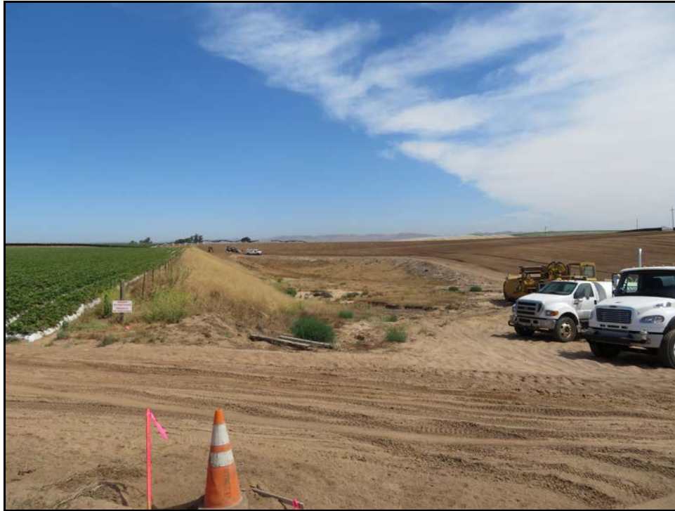
CTE Ag Center - The Squash is Harvested and Earth Moving Equipment Moves In
