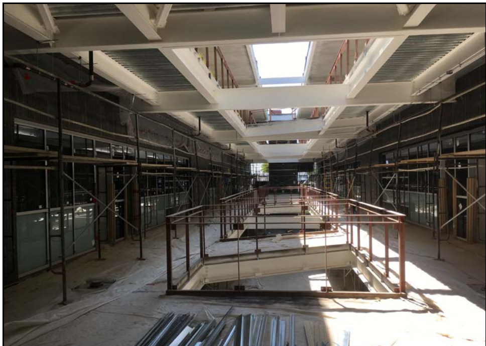
ERHS 38-Classroom Building – Classroom Windows Installed and Plastering In Progress
