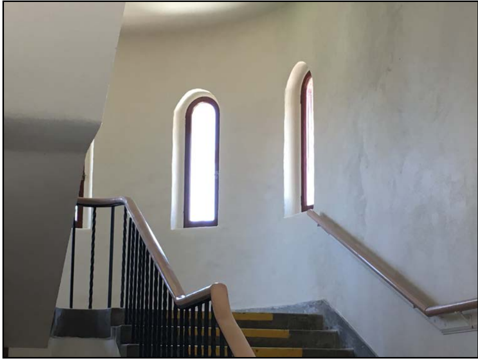
SMHS - ... and Following Roof Repair, Plaster Repair, and Paint
