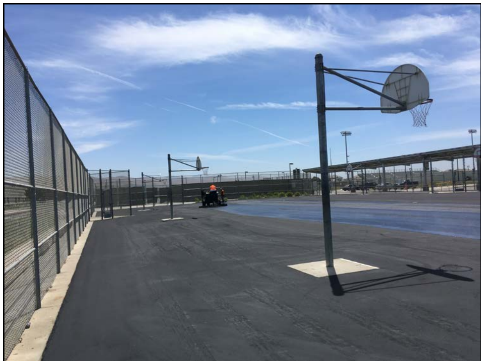
PVHS - Slurry Seal Goes Down on the Outside Basketball Courts
