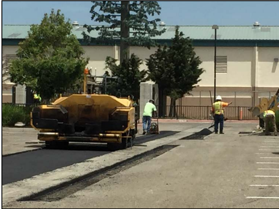
PVHS - Asphalt Replacement in the Front Parking Lot
