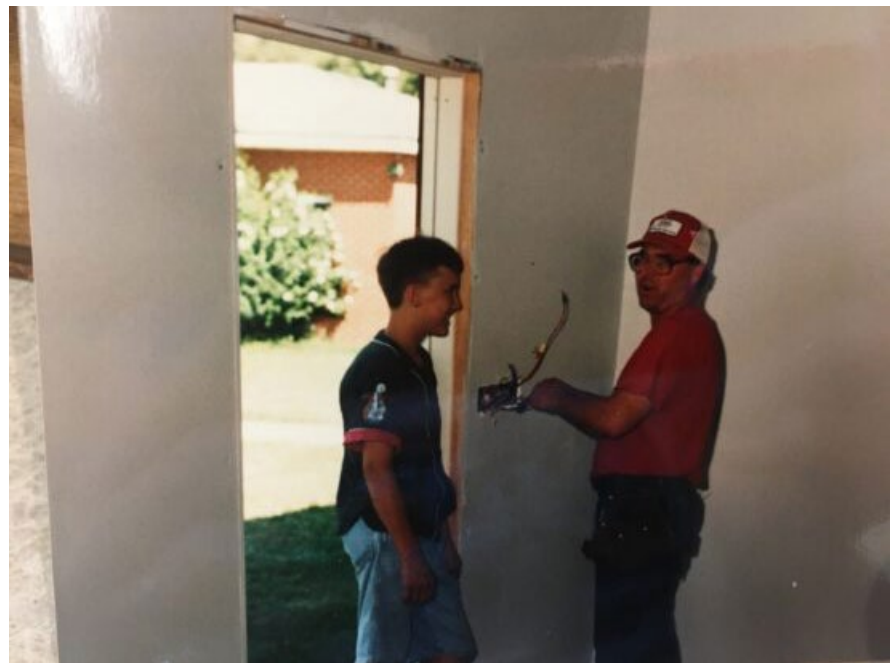
John Patrick (left, class of '99) helps with wiring new switches across campus.
