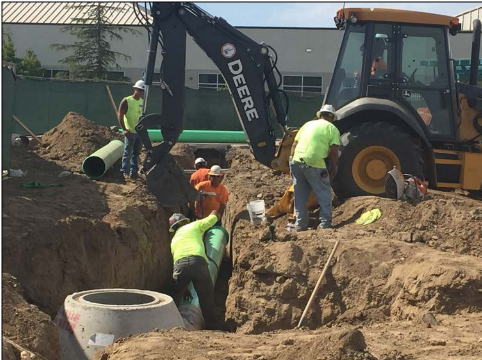
PVHS – Performing Arts Center Storm Drain is Relocated
