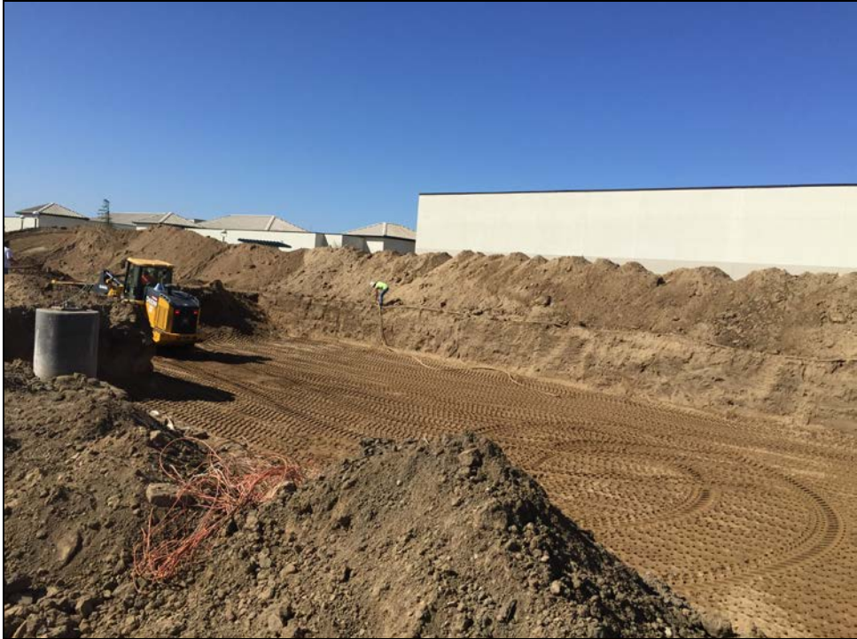
PVHS – Foundation Base Compaction Begins at the Performing Arts Center
