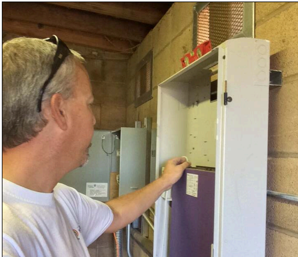
ERHS - Del Ward Upgrades the Communications Switch Installation at the Well Pump House
