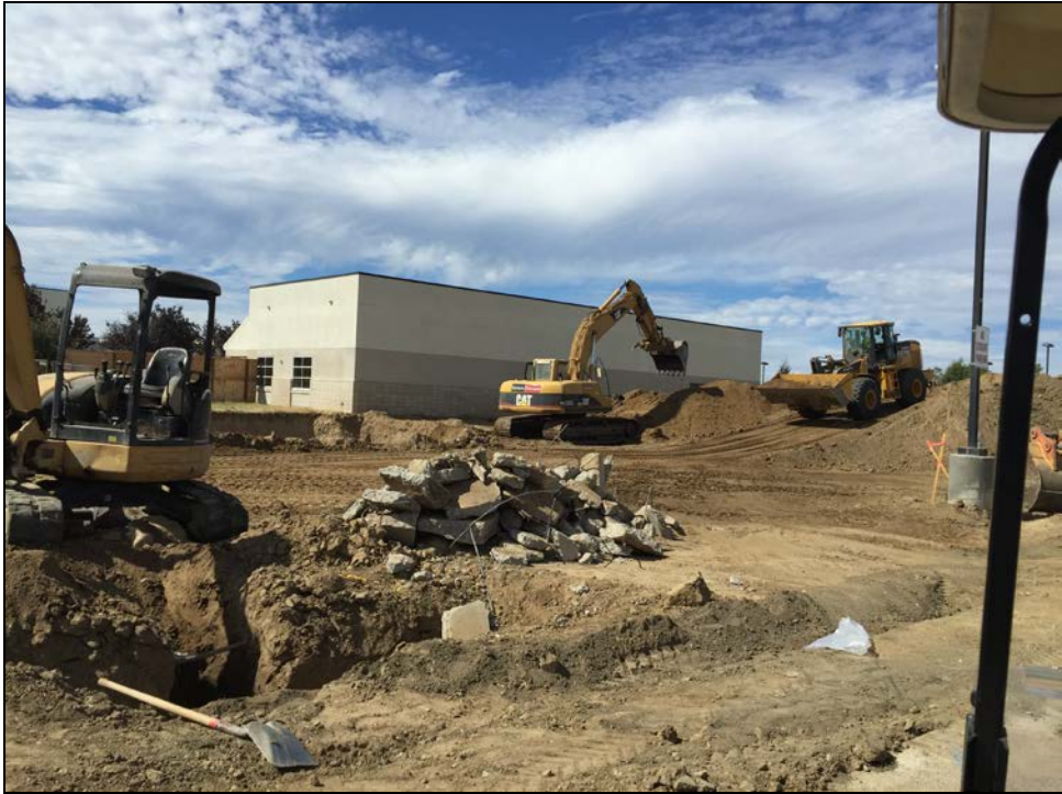
PVHS – Compaction of the Foundation Base Requires Moving a lot of Earth
