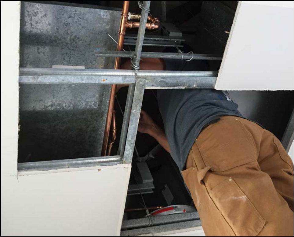
PVHS - Flavio Rodriguez Installs a New HVAC Condensate Drain Pump and Line
