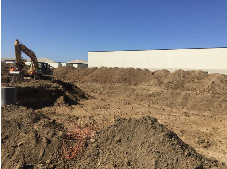
PVHS – Foundation Excavation Underway for the Performing Arts Center
