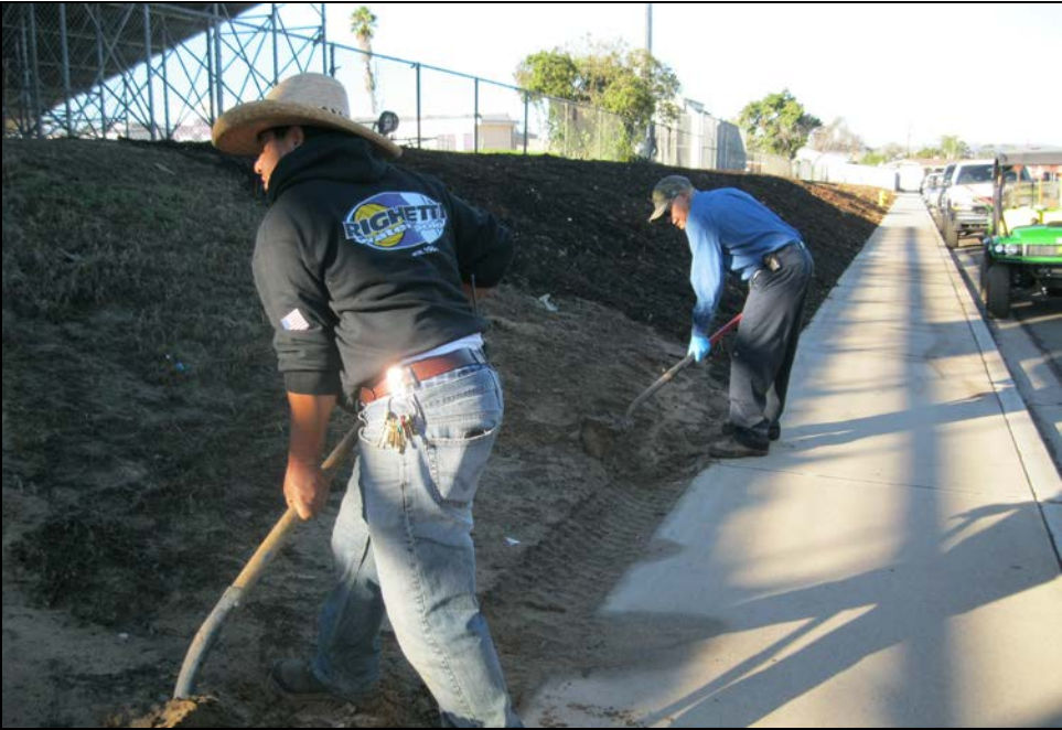
ERHS - Leo Avila and Juan Rodriguez Prepare Larch Street Slope for Recycled Material
