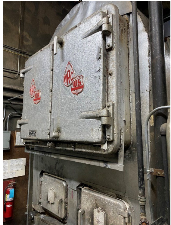
Existing Pellet Boiler
