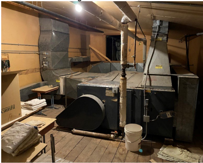
Existing Classroom AHU (Retired)
