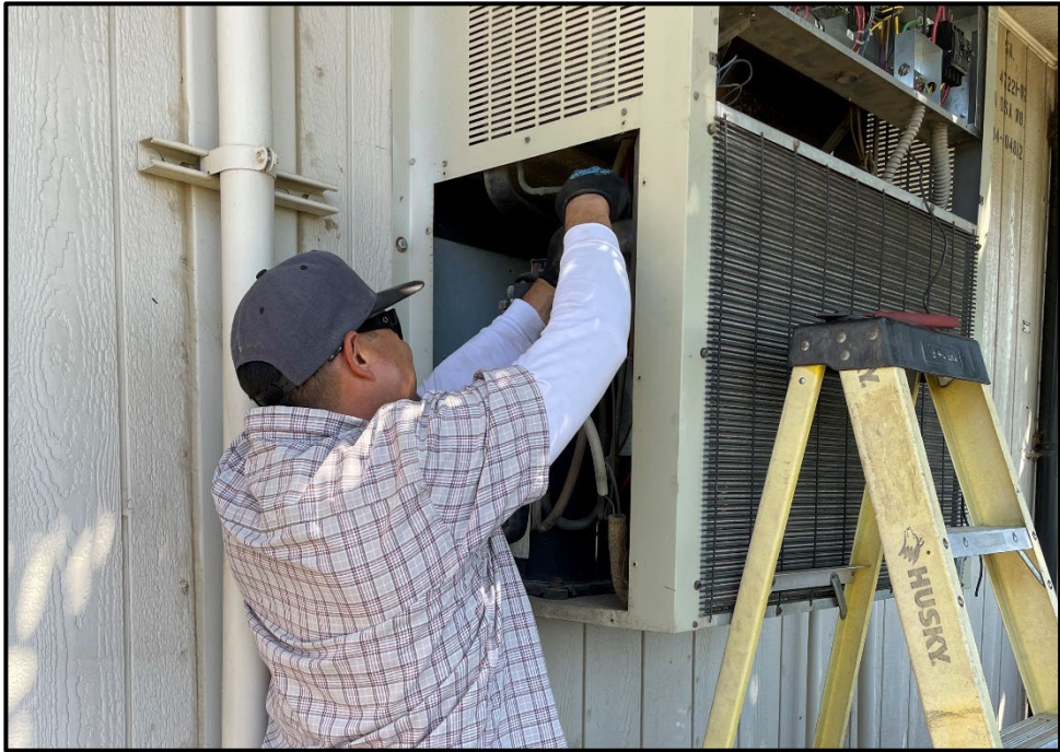
PVHS – Elias Camacho Repairing an HVAC Unit
