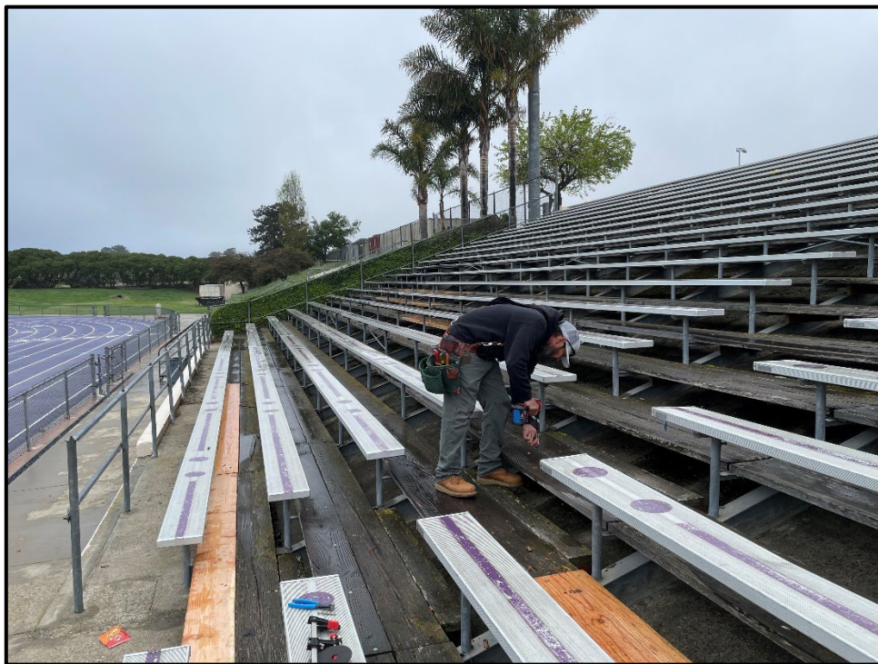
ERHS – Tom Harbold Repairing Stadium Bleachers for Graduation
