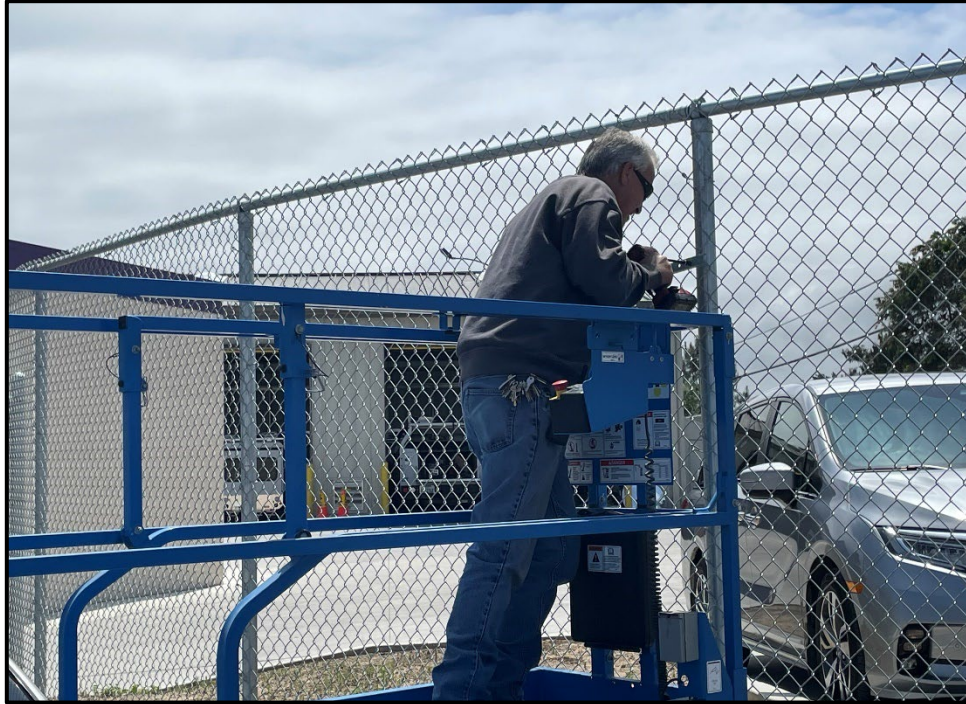
ERHS – Del Ward Installing a Convex Mirror at the Maintenance Shop
