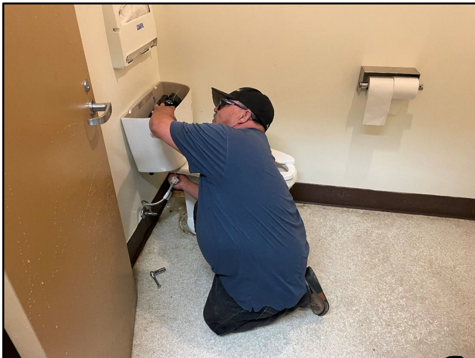
SMHS – Jesus Reyes Repairing a Leaking Toilet
