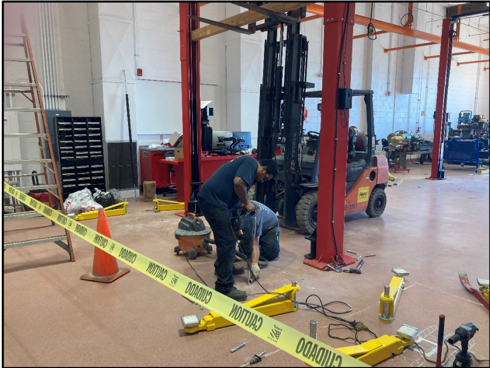
SMHS CTE Modernization – Installing Vehicle Lifts for the Auto Shop
