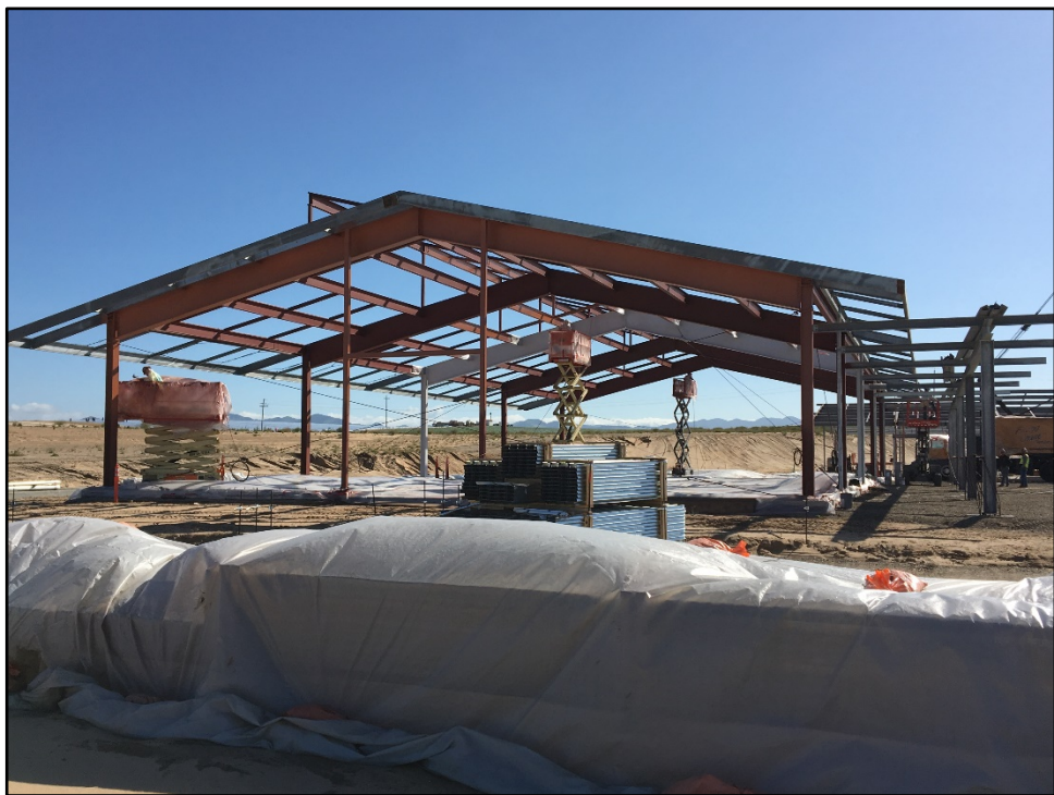
CTE Ag Center – Shop Building B Steel Receives Paint from Three Painters
