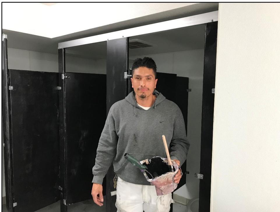
ERHS – New Painter Joel Amezqua Paints over Vandalism in the Press Box Restrooms
