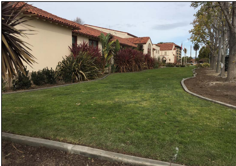
SMHS – Plastic Landscape Border Replaced with Concrete in Broadway Planter
