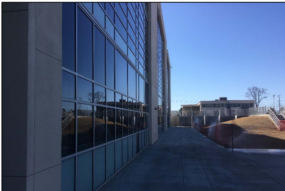
ERHS 38-Classroom Building – Grass is Planted on the North side of the New Building
