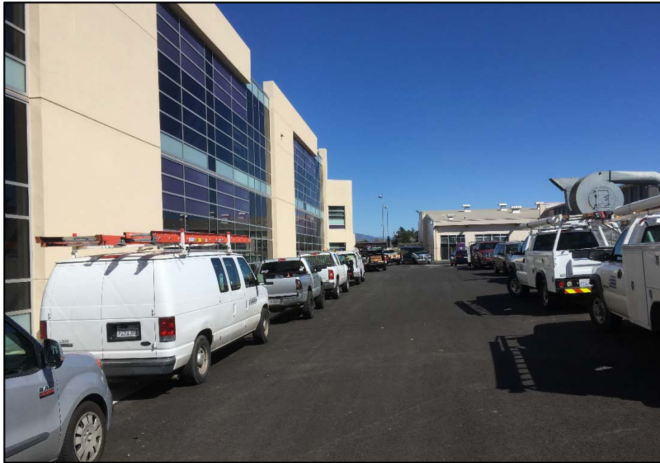
ERHS 38-Classroom Building – The Final Push to Finish Construction – New Paving Makes a Great Construction Parking Lot
