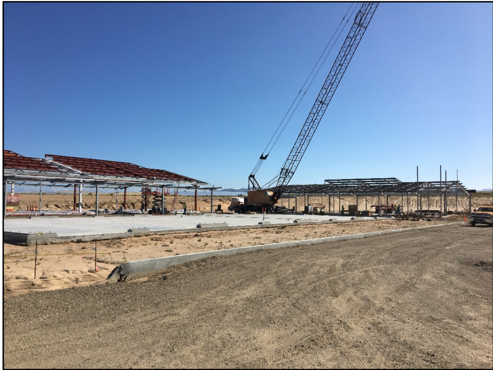
CTE Ag Center – Culinary Arts Building Steel is Erected
