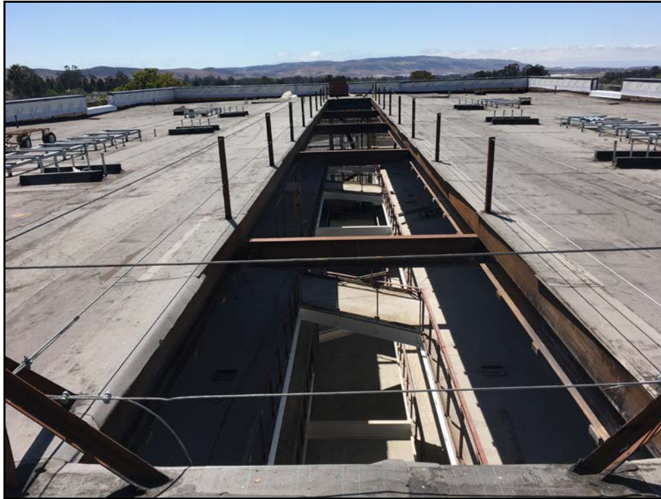
ERHS 38-Classroom Building – Roof-top View: First Phase of Roofing
