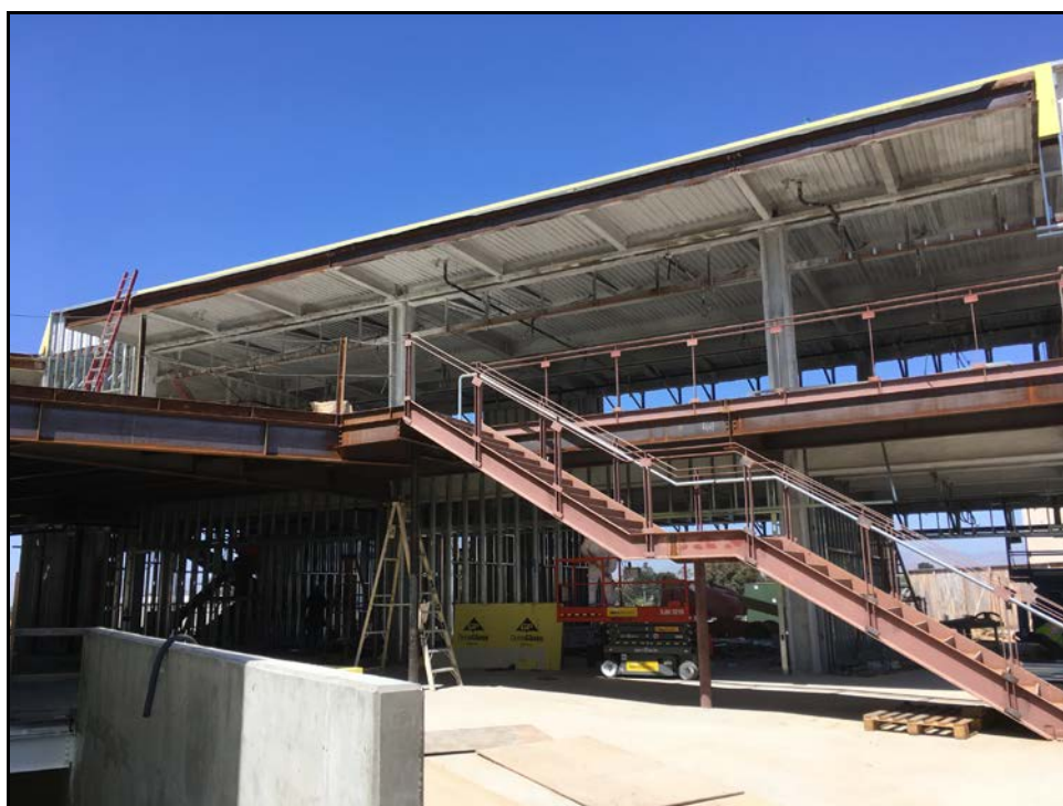
ERHS 38-Classroom Building – Top and Second Floor of the East Building for Framing Classrooms
