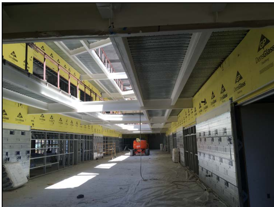
ERHS 38-Classroom Building – Various Stages of Painting, Insulation, and Waterproofing
