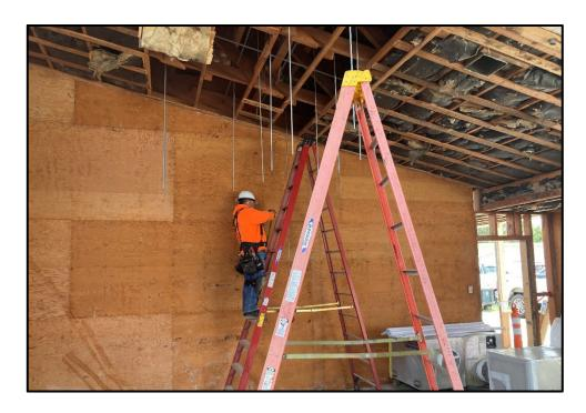
SMHS 37 Classroom – Installing Hanging Supports for HVAC Installation
