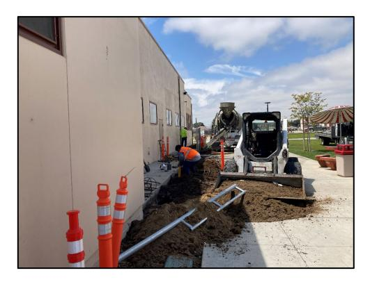
SMHS 37 Classroom - Pouring Concrete Pads for HVAC Unit Installation
