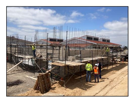
MRCTECAF M&O Building – Building the Exterior Walls and Installing Electrical
