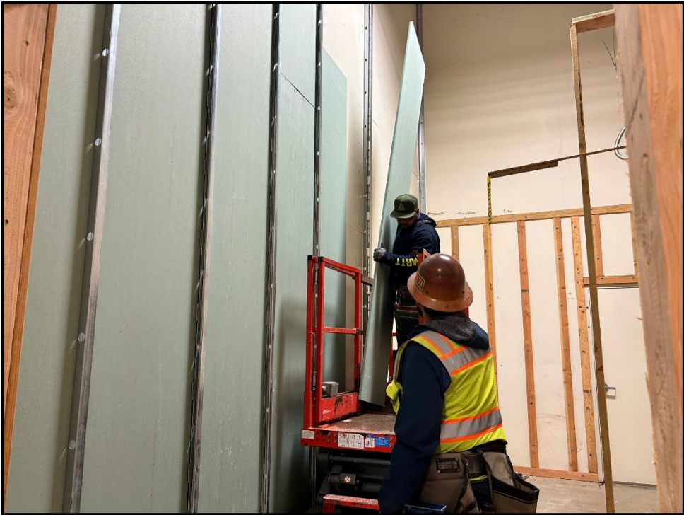
SSC Tire Room Reconfiguration – Drywall Installation Begins in the Old Tire Room
