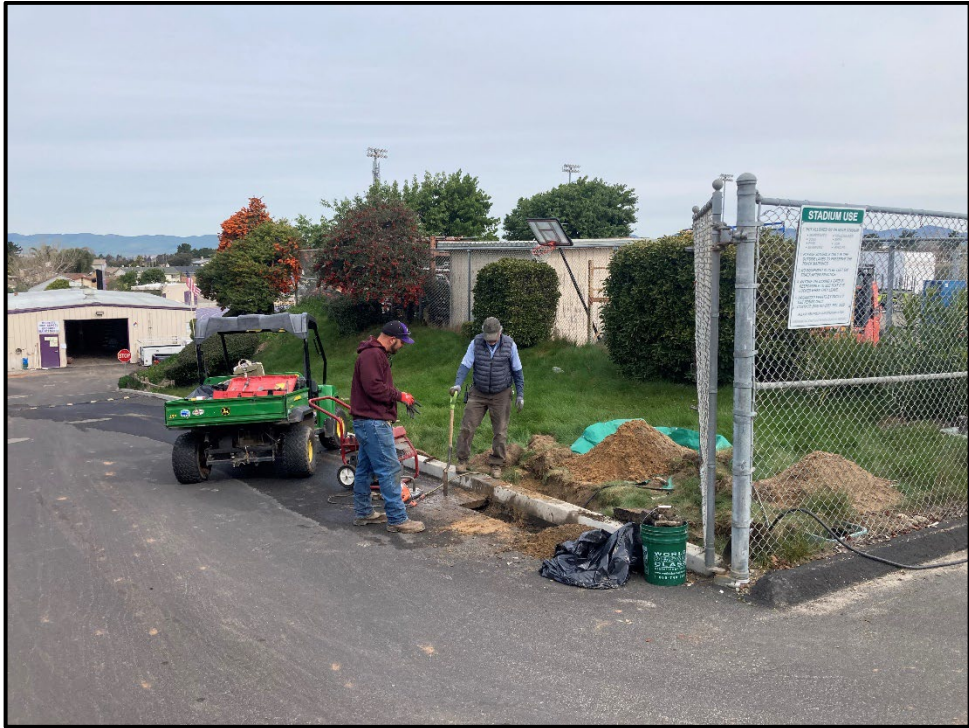
ERHS – Jordan Markstone and Juan Rodriguez Repairing an Irrigation Leak
