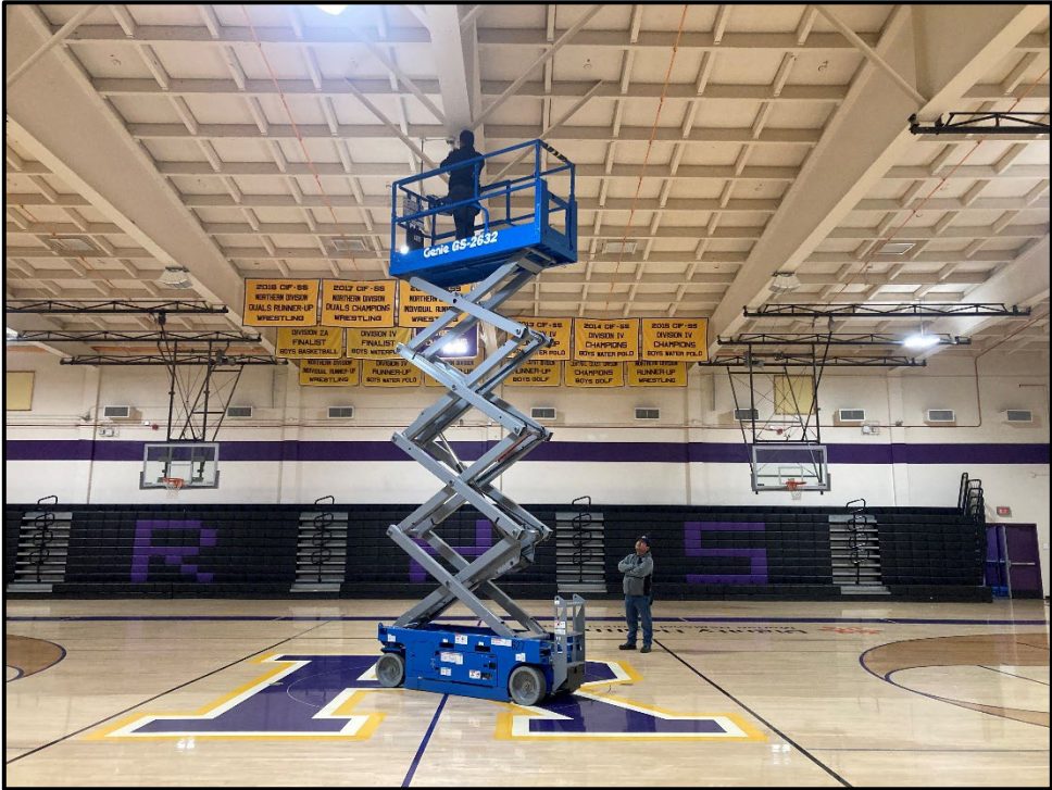
ERHS – Leo Avila Replacing the Basketball Safety Strap in the Gymnasium
