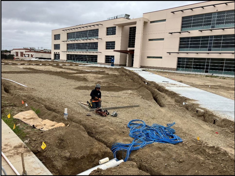
SMHS 50-Classroom Building – Irrigation Control Wire and Branch Piping are Installed
