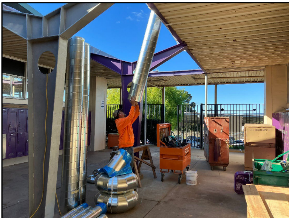
ERHS Modernization – Installation of New HVAC Ducting Nears Completion
