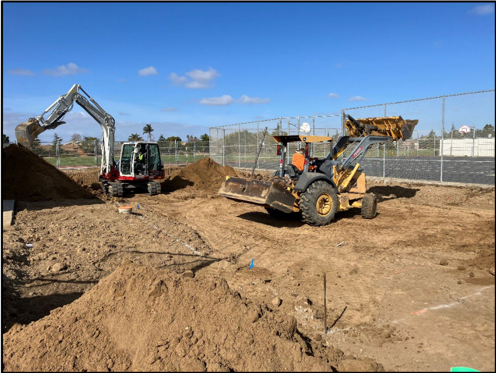
PVHS New Modular Classrooms – Over Excavation for Footings is Underway
