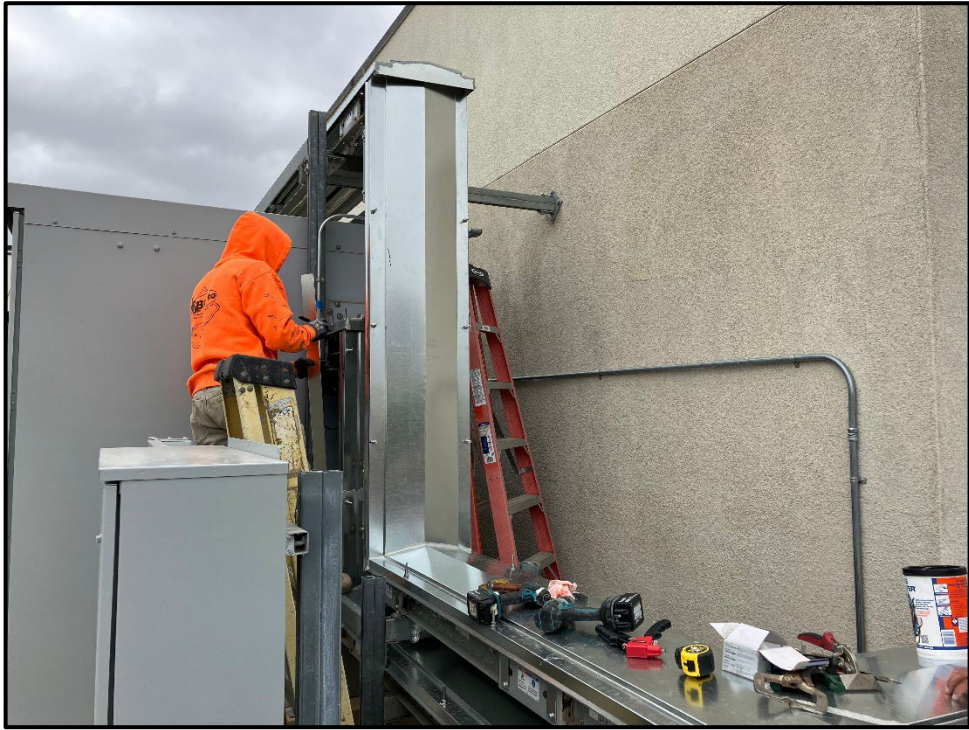
PVHS – Main Electrical Feeder Busway Receives a Protective Roof
