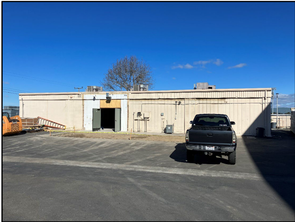
ERHS Modernization – The Agriculture Science Building without the Beef Kill Room
