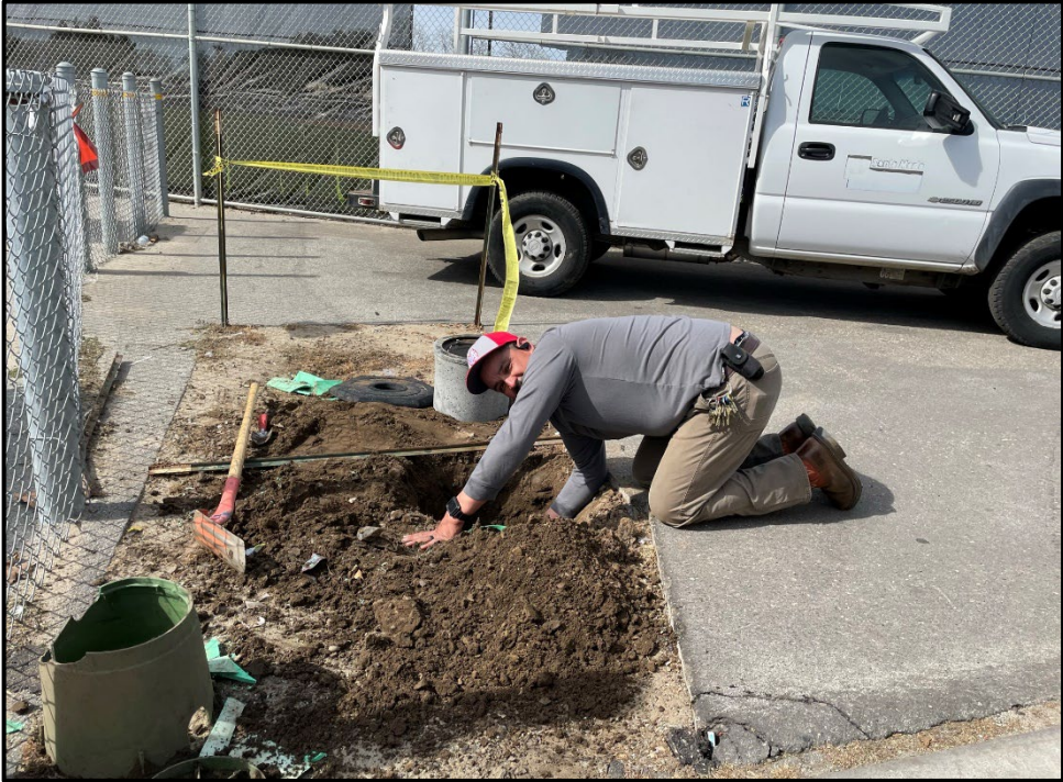
SMHS – Alan Rodriguez Installing a New Irrigation Valve Box
