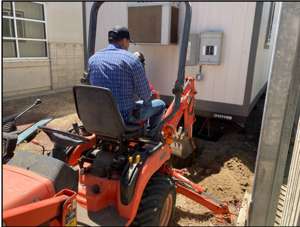
PVHS – Jose Gamino and Daniel Pinon Trenching for the New Communication Lines to the New Office IT Trailer
