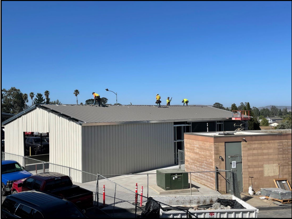
ERHS M&O Building – The Metal Roofing is Completed
