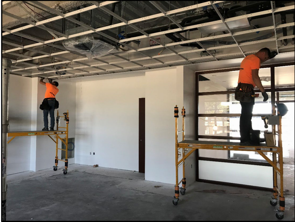
SMHS 50-Classroom Building – Suspended Grid Ceiling Installation
