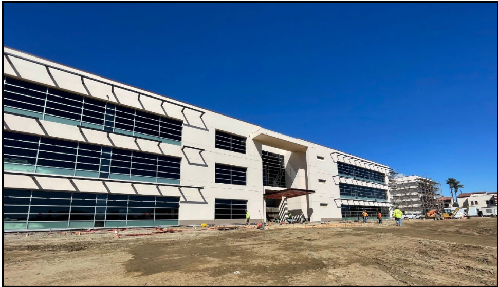
SMHS 50-Classroom Building – The Southern Exterior is Nearing Completion and Awaiting Shade Panels
