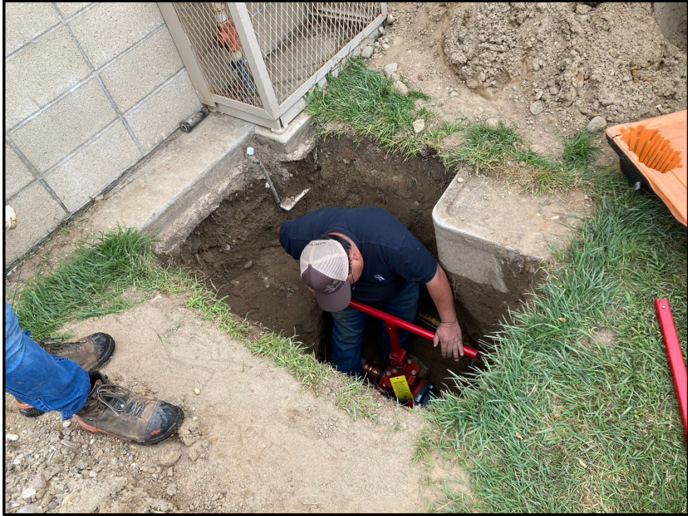
PVHS – Jesus Reyes Replacing a Leaking Valve on the Cafeteria Water Line
