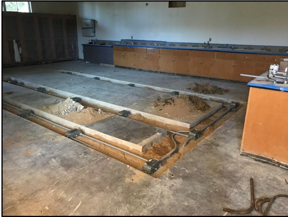
ERHS Modernization – Updated Electrical is Installed in the Floor
