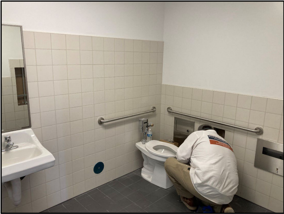
ERHS M&O Building – Restroom Fixtures Installation
