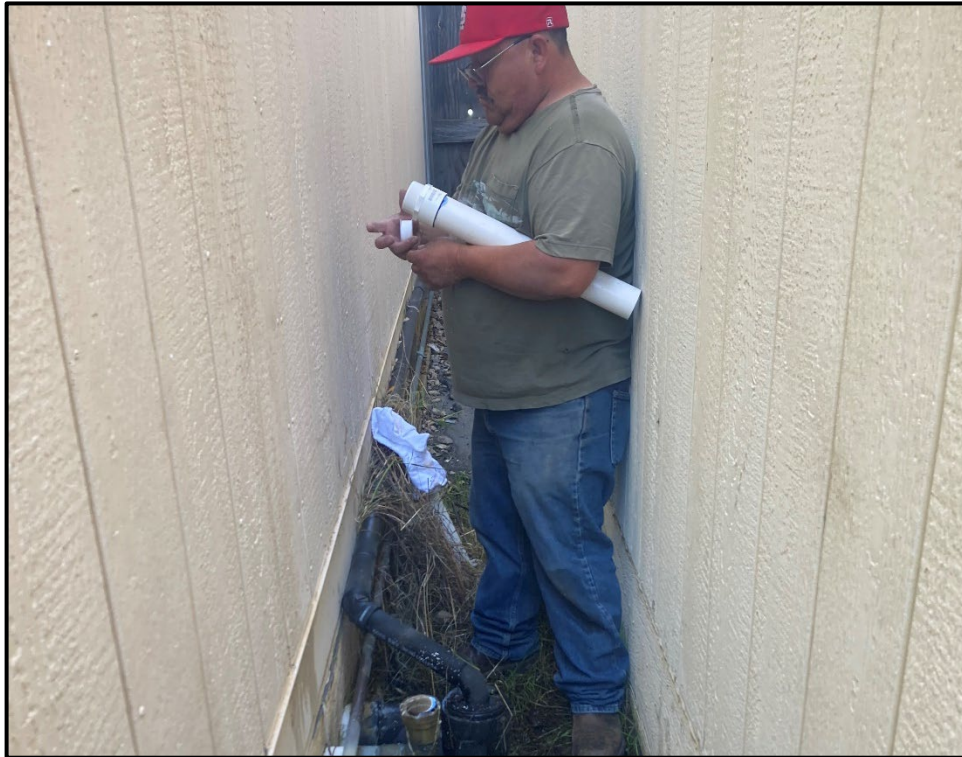
SMHS – Jesus Reyes Repairing the Main Water Line at the Lincoln Center
