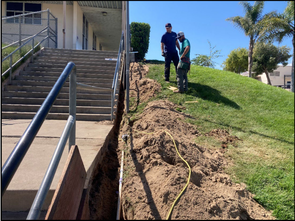
ERHS – Tom Harbold and Jordan Markstone Removing Railroad Ties in Preparation for a New Retaining Wall
