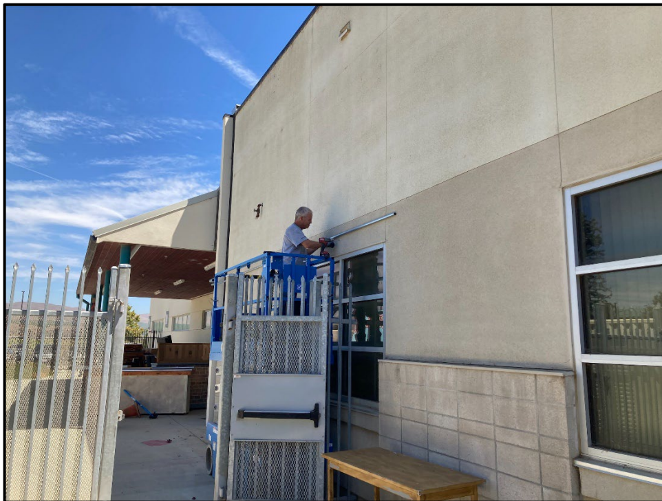
District Maintenance – Del Ward Installing Electrical and Communication Cables to the New IT Trailer
