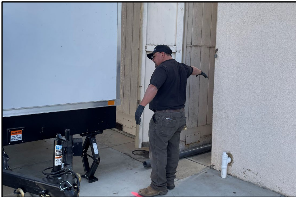
SMHS – Jesus Reyes Connecting the Plumbing for the New Portable Restroom Trailer to Support the Additional Portable Classrooms
