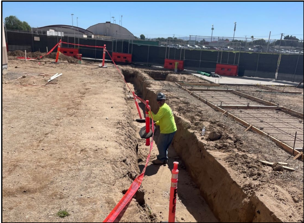
SMHS 50-Classroom Building – Trenching Begins in Preparation for Landscaping and Irrigation
