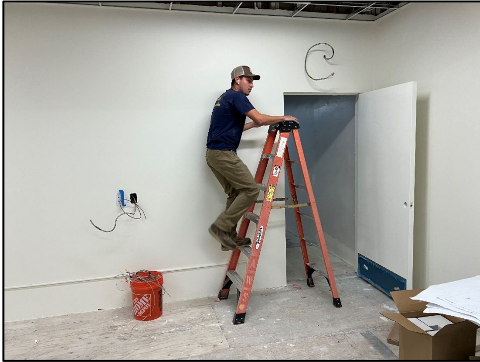
SSC Second Story Reconfiguration – Electrical Installation in Progress
