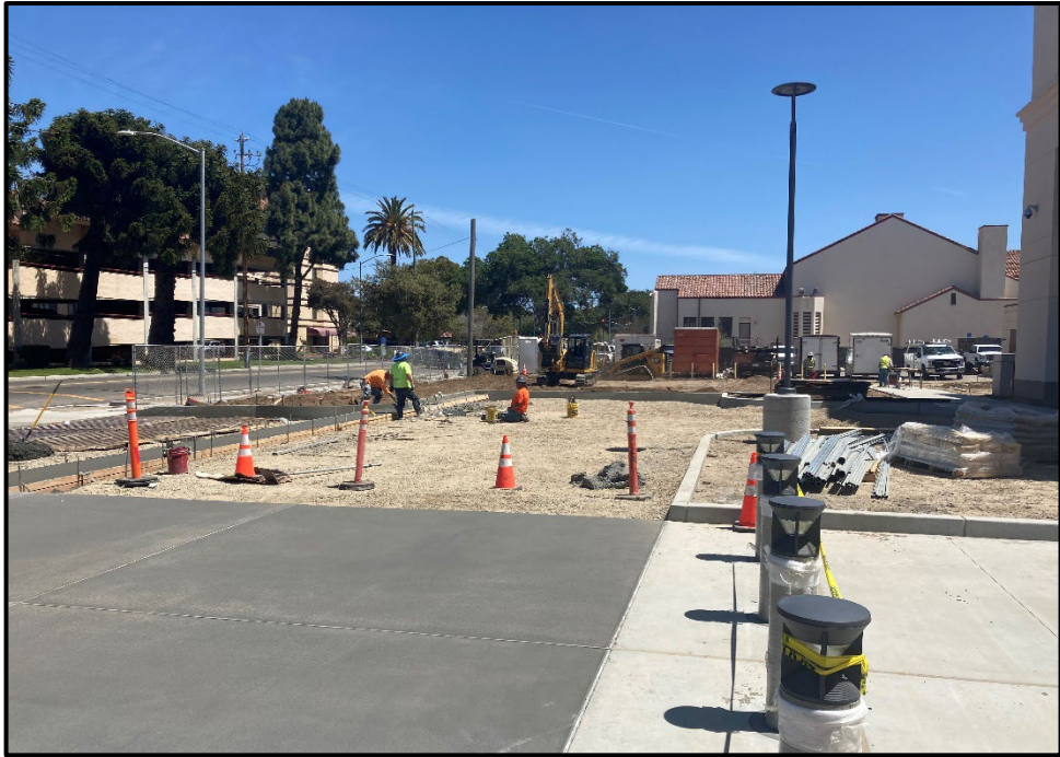
SMHS 50-Classroom Building – Forming Curbs and Gutters for the Parking Lot
