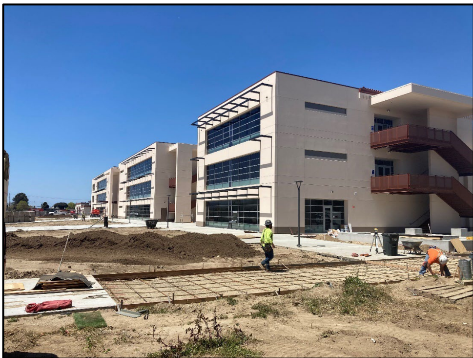
SMHS 50-Classroom Building – Preparing to Pour Concrete Walkways
