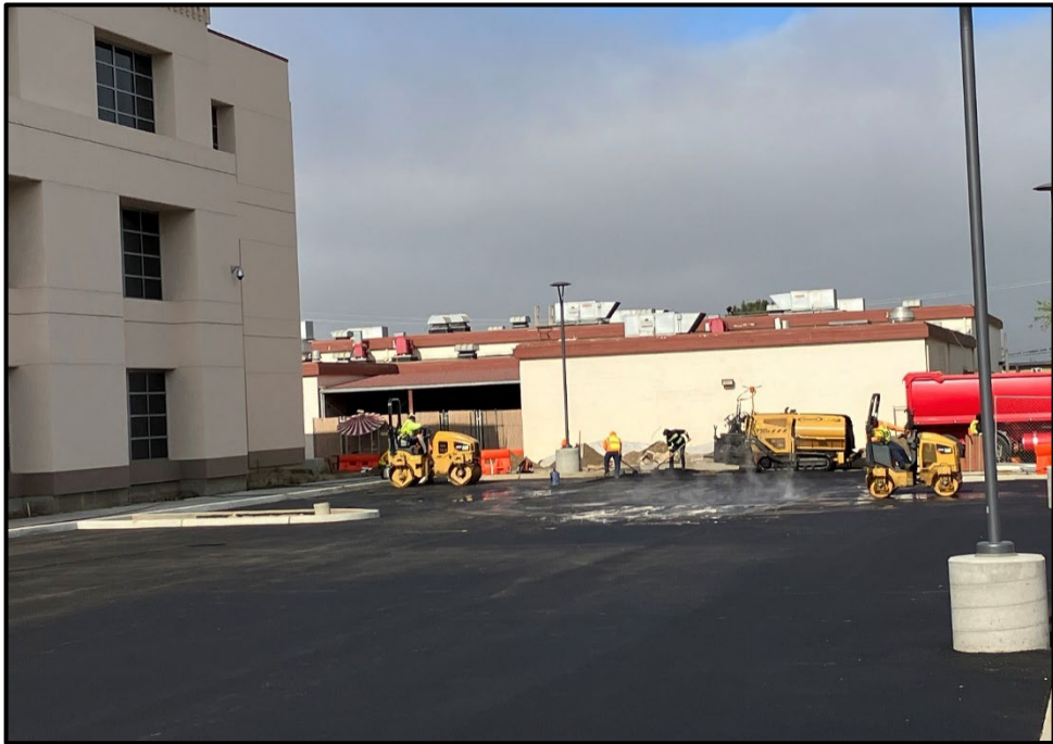
SMHS 50-Classroom Building – Paving Morrison Street Parking Lot
