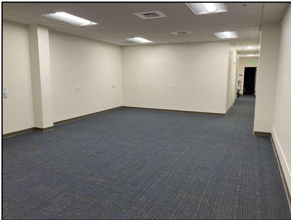
SSC Second Story Reconfiguration – Lighting, Ceiling Tiles, and Carpet are Installed
