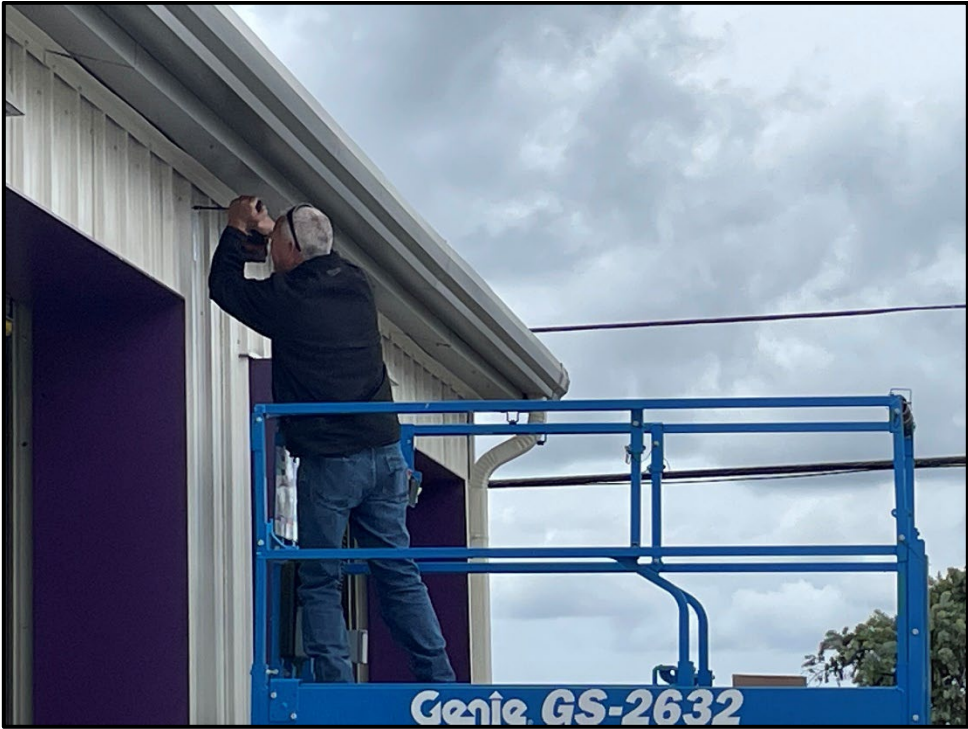
ERHS – Del Ward Begins Security Camera Installation at the Maintenance Shop
