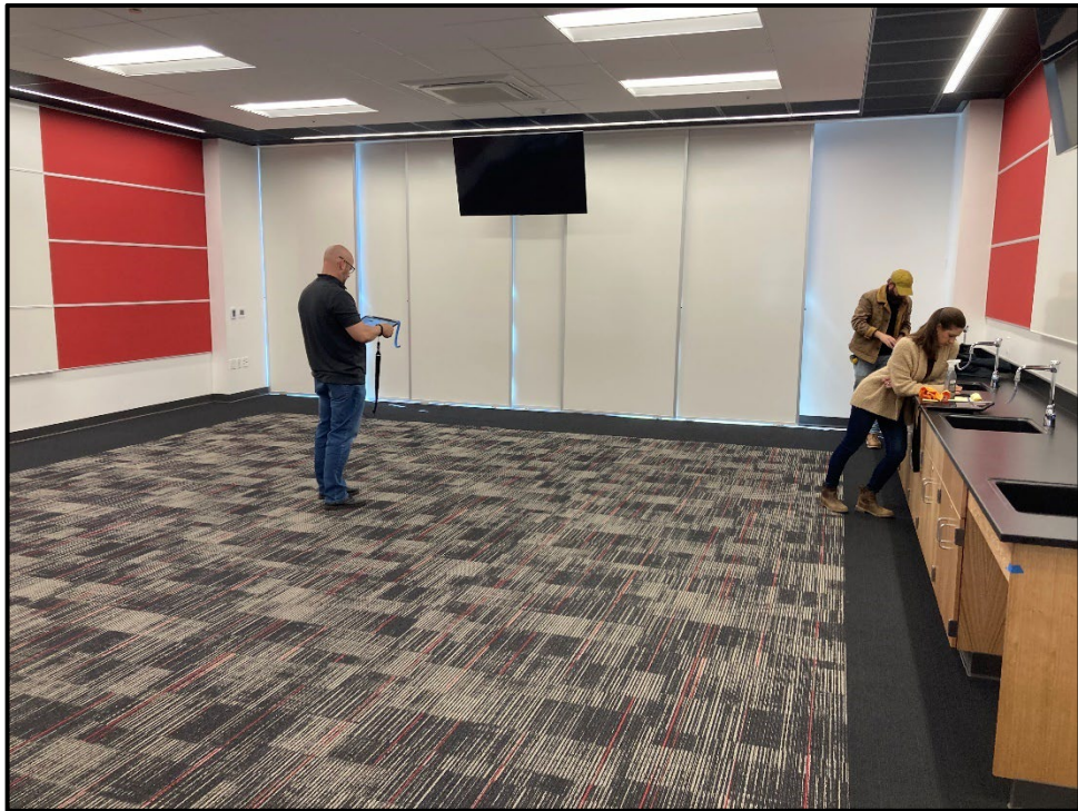
SMHS 50-Classroom Building – Construction Team Checking Punch-list Items
