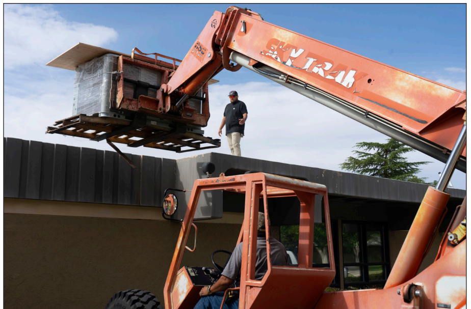
The maintenance crew installs a new HVAC unit on the roof of the high school in August.
