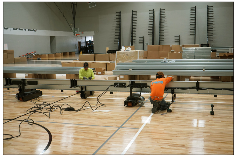
Contractors install new bleachers in the high school's main gym.
