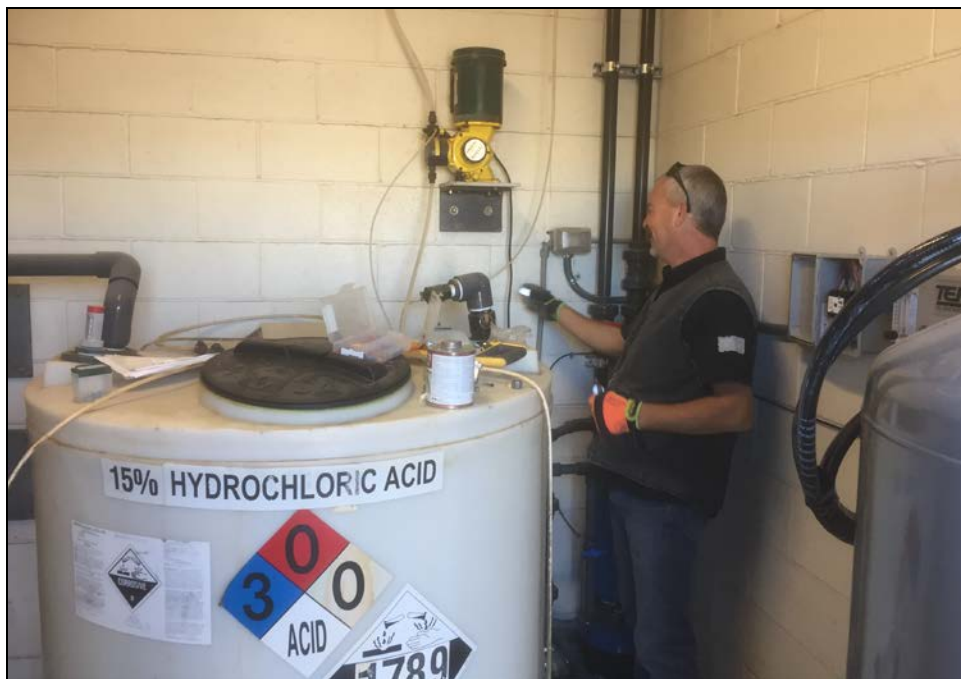
PVHS – Del Ward Completes Wiring for the New CO 2 Dispensing System at the Pool
