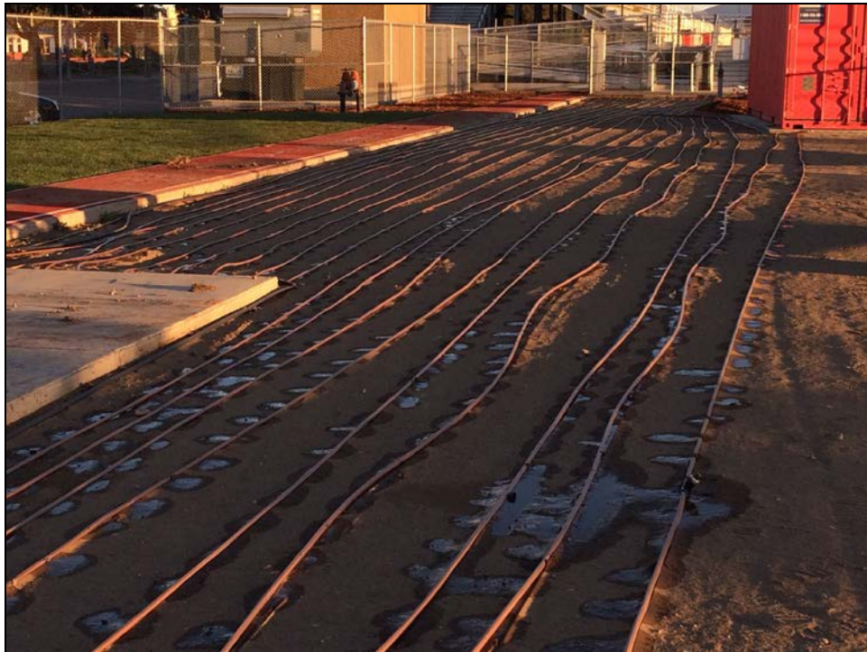
SMHS – Subsurface Landscape Irrigation is Tested Prior to Laying Sod
