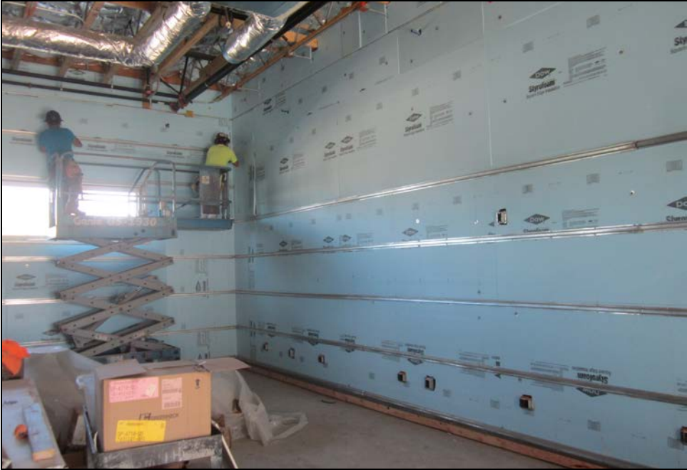
PVHS Performing Arts Center – Interior Insulation and Drywall Installation is Underway
