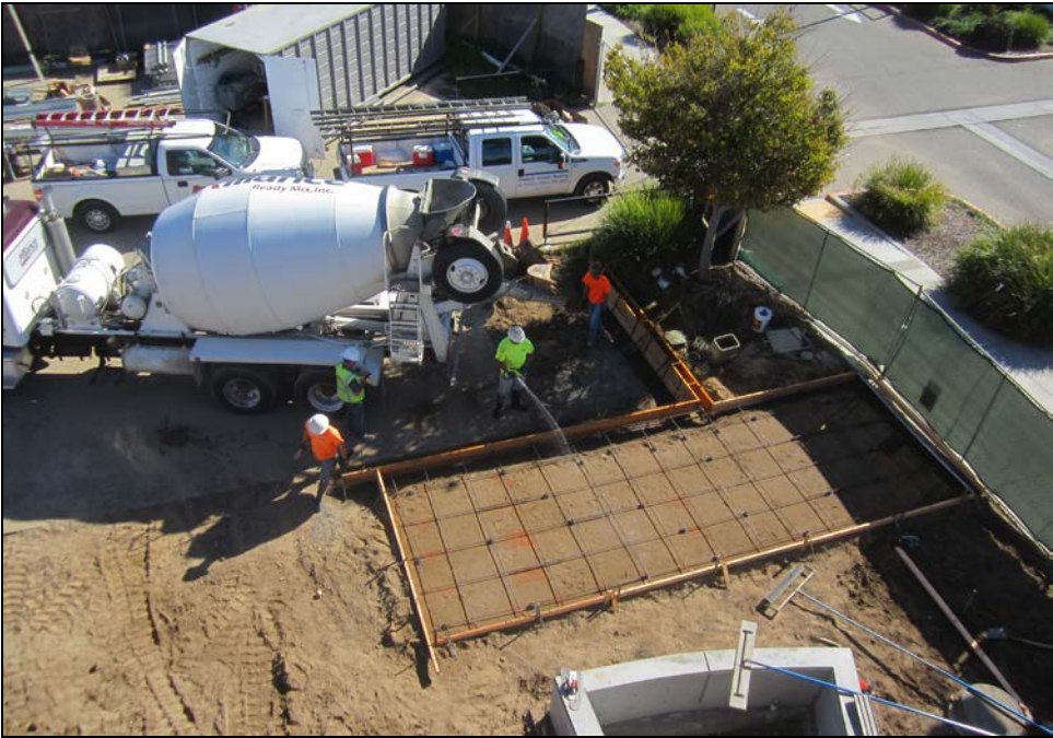
PVHS Performing Arts Center – Exterior Concrete Pour In-progress
