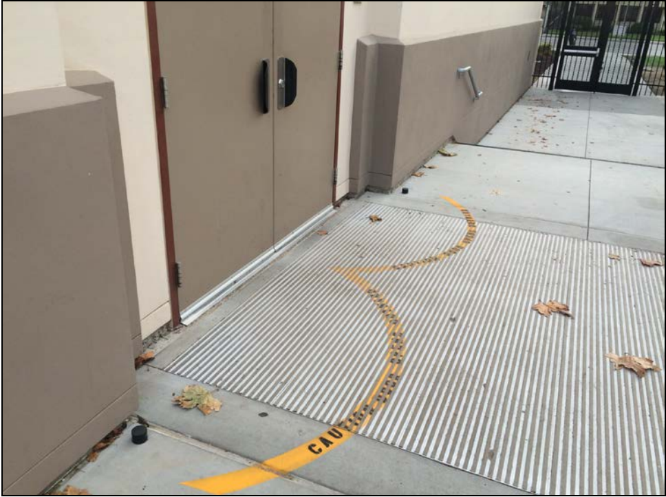
SMHS - Exterior Door Safety Issue is Addressed at the Broadway Classroom Building
