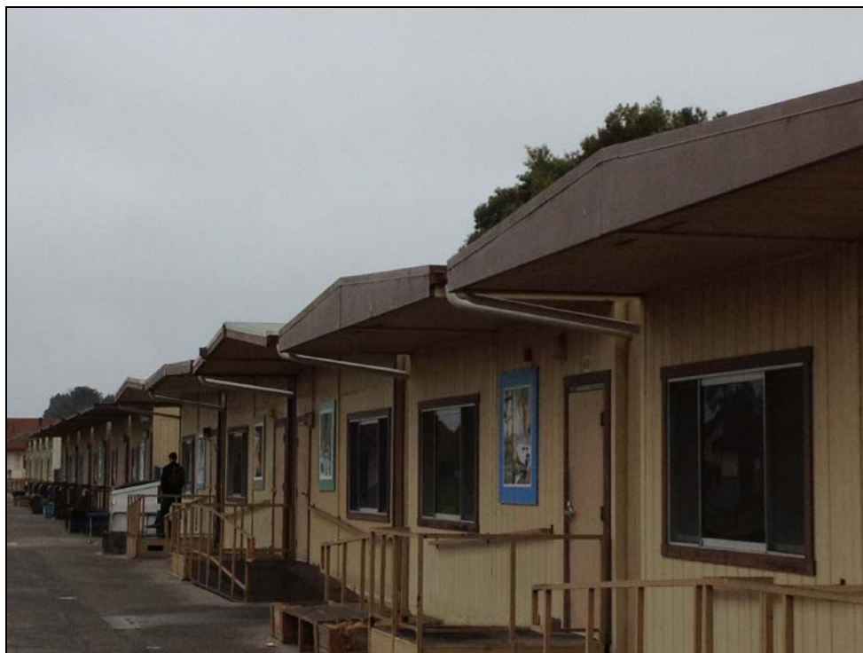
SMHS – Rain Gutter Installation on Five Classrooms
