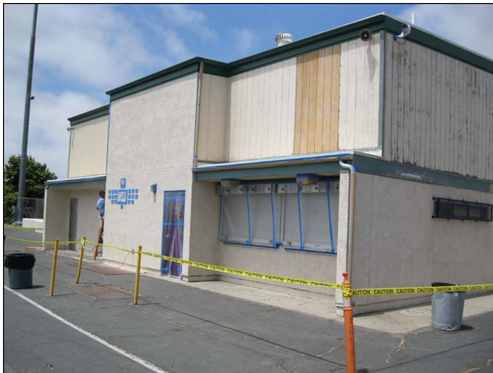
ERHS Press Box - Repainting the Restroom and Concession Area
