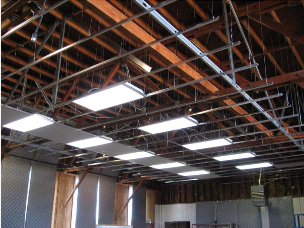
SMHS Band Room Acoustic Ceiling & Lighting Upgrades
