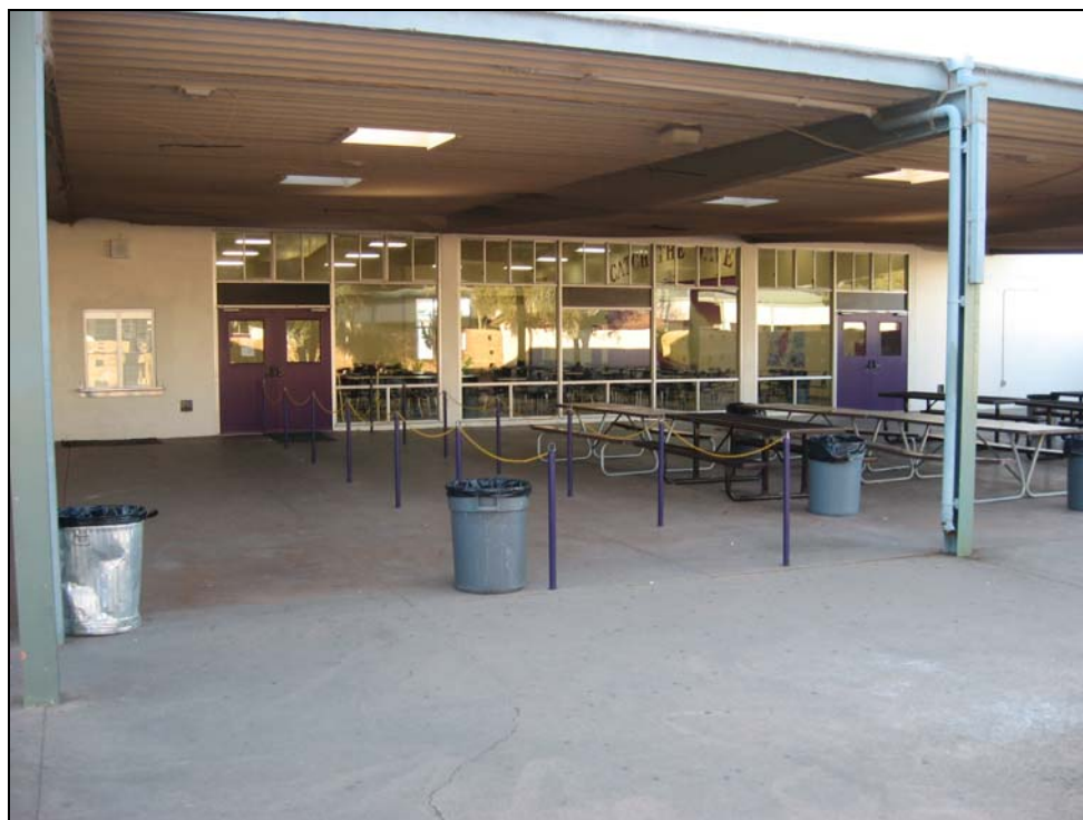
RHS Cafeteria Lunch Line Improvements
