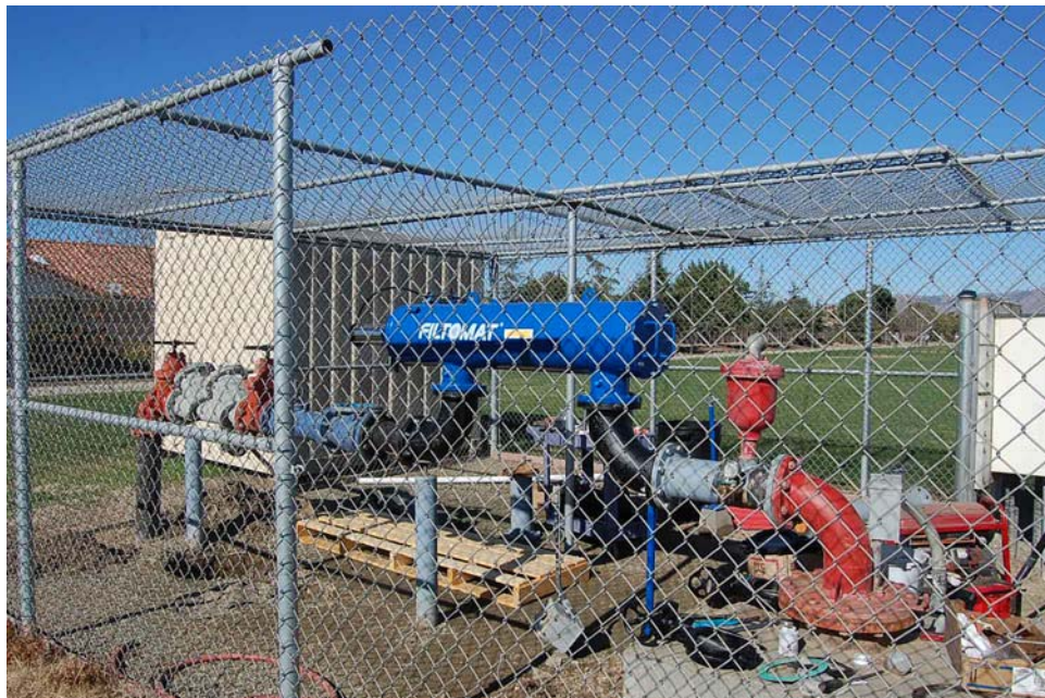
PVHS Irrigation Well Sand Filter Installation
