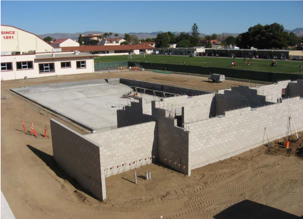
SMHS Pool Equipment Room Walls Erected
