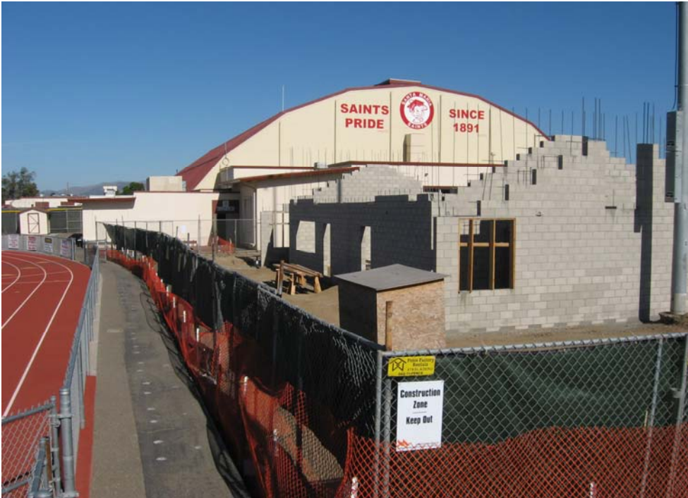
SMHS Pool Concession and Restrooms Proximity to Football Stadium
