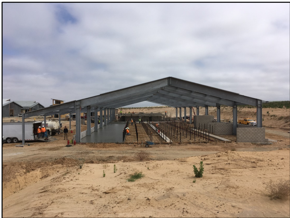
CTE Ag Center – Barn Concrete Floors Begin to Take Shape
