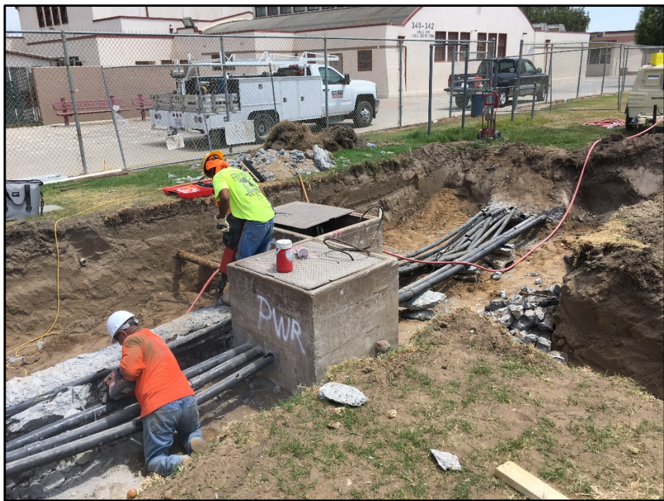
SMHS Reconstruction – 4160 Volt Power Distribution in Progress
