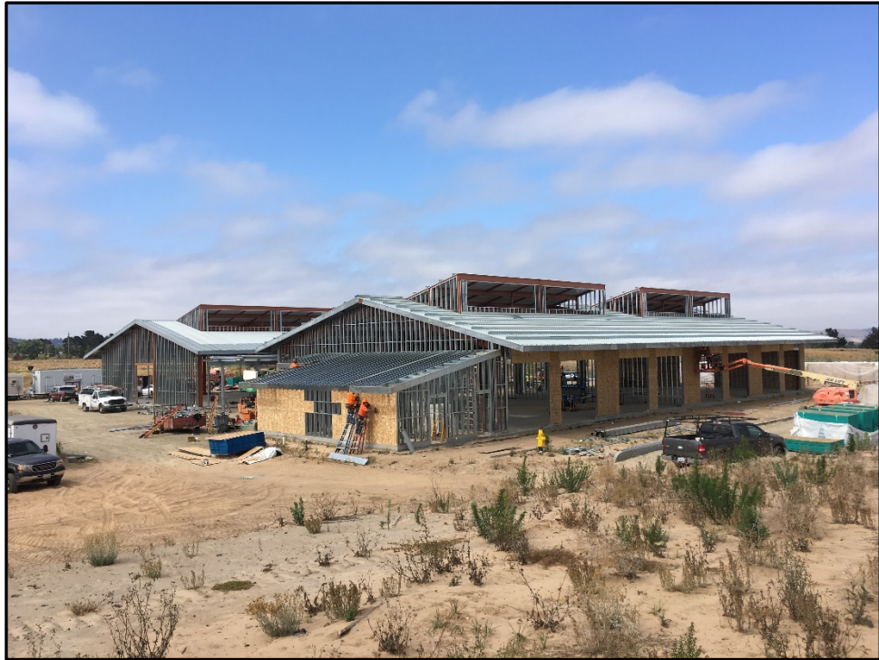
CTE Ag Center – Shop Buildings Receive Wood Sheathing over Metal Studs
