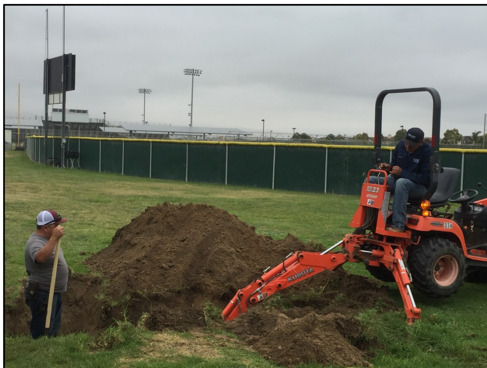
PVHS - José Gamino and Jesus Reyes Excavate to Install Ez-Flo Injection in Irrigation
