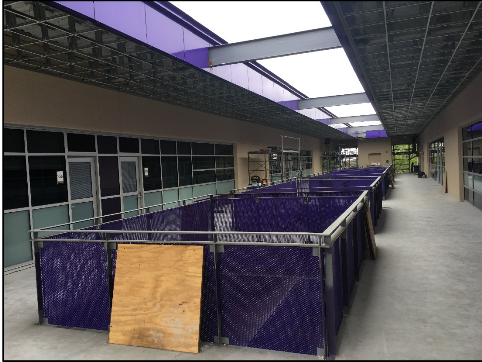
ERHS 38-Classroom Building – Exterior Ceiling Tiles and Revised Walkway Panels are Installed
