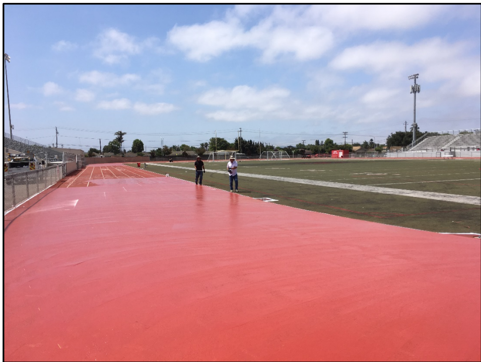
SMHS Track Resurfacing – Slurry Coat is Applied and Awaiting Rubber Granules
