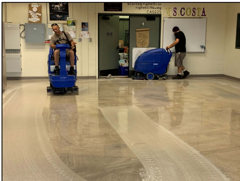
ERHS - Custodians Operate Auto Scrubbers to Prepare Floors for New Finish
