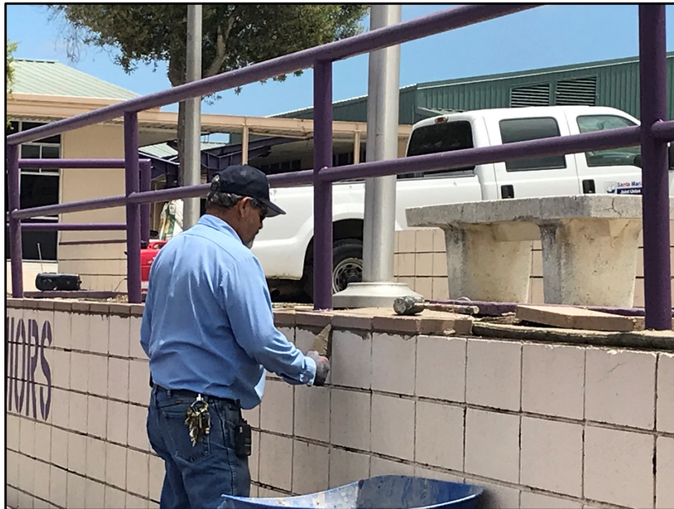
ERHS - José Placencia Replaces Wooden Caps on Block Walls in the Quad
