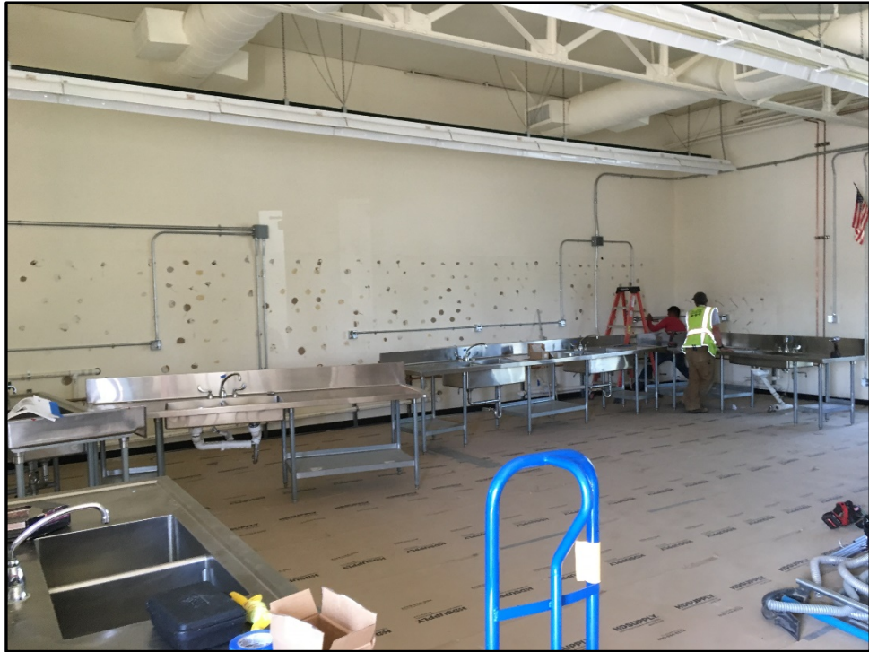
SMHS Reconstruction – Temporary Culinary Arts Classroom Conversion Takes Place
