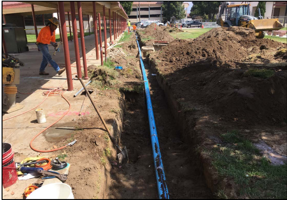
SMHS Reconstruction – Revised Water Line Installation Underway
