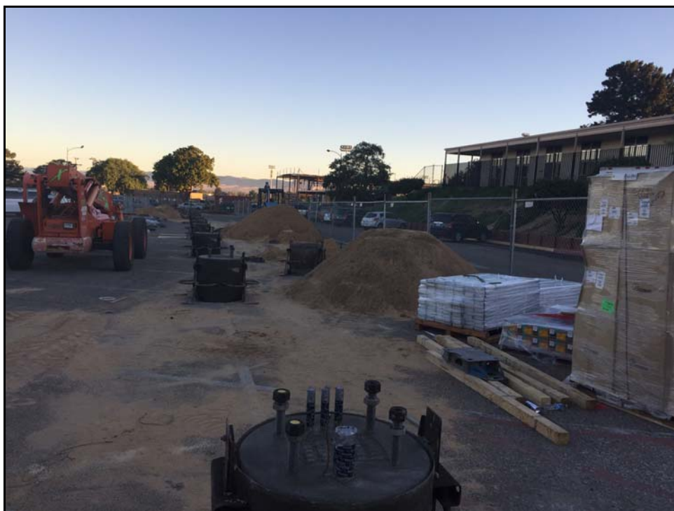
ERHS Solar Installation – Concrete Footings Poured and Curing in Phase I
