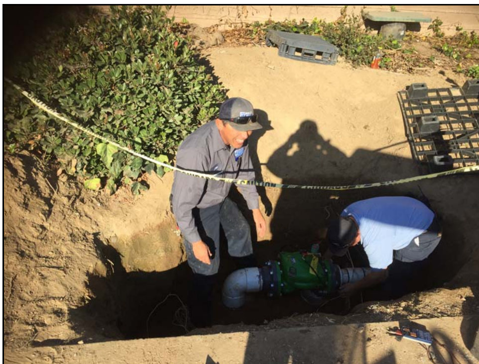
PVHS – José Gamino and Jesus Reyes Replace an Irrigation Control Valve
