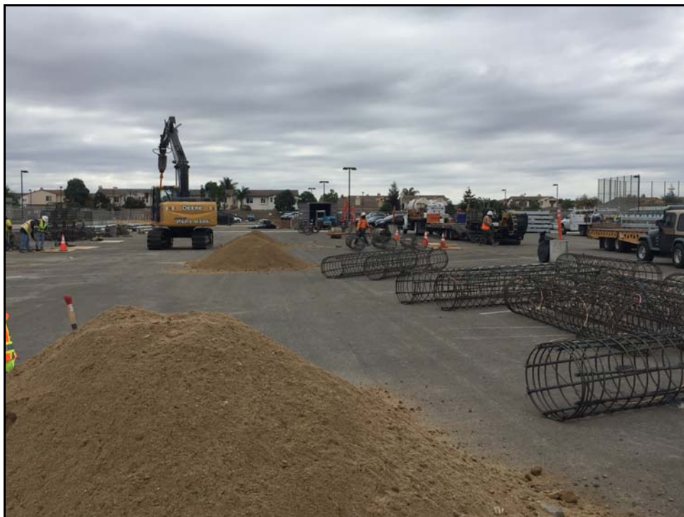
PVHS Solar Installation – Drilling for Footings Underway
