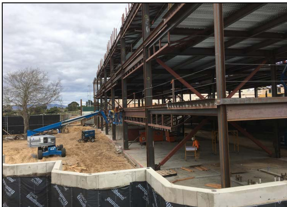
ERHS 38 Classroom Building – Structural Welding in Progress; Floor Decking in Place
