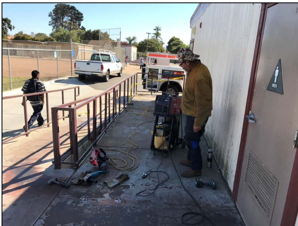
SMHS – José Placencia Performs Welding Repairs on an Access Ramp
