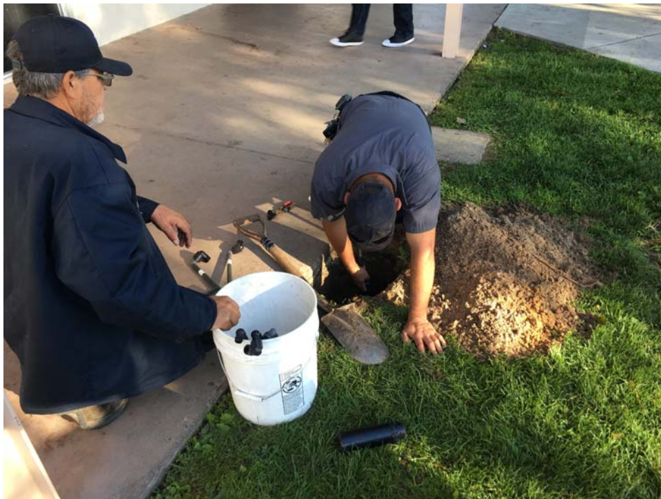
ERHS - Juan Rodriguez Trains Nelson Frutos on Sprinkler Installation Details
