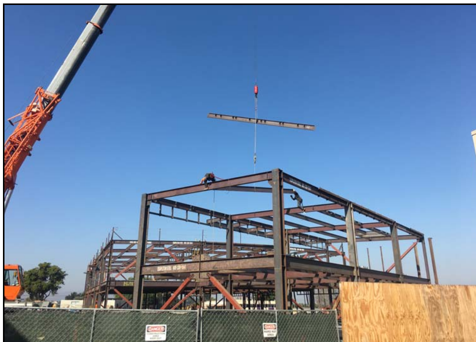
ERHS 38 Classroom Building – Third Floor Steel is Set for the East Structure
