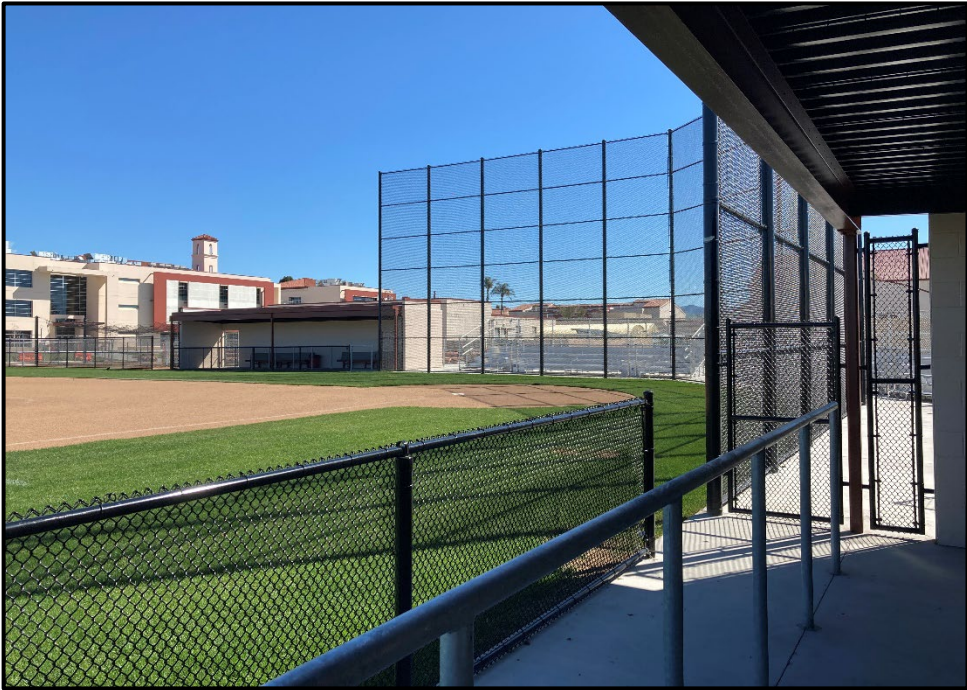
SMHS Softball Field Reconfiguration – Completed Field from the Dugout
