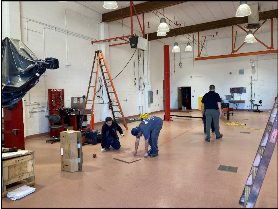
SMHS CTE Modernization – New Two-Post Lift Installation In-progress
