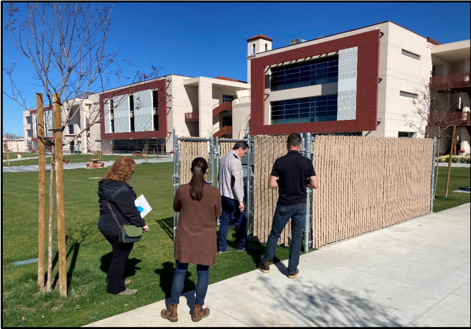
SMHS 50-Classroom – Punch Walk In-Progress
